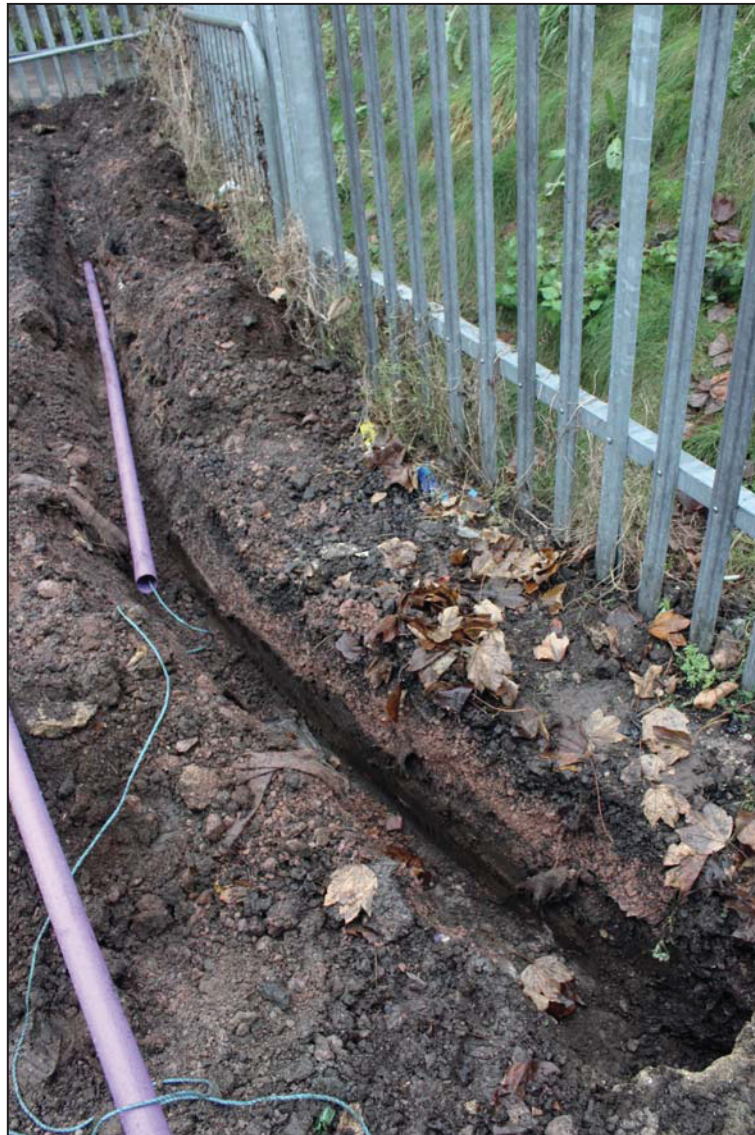
Trench 2, looking north-west
