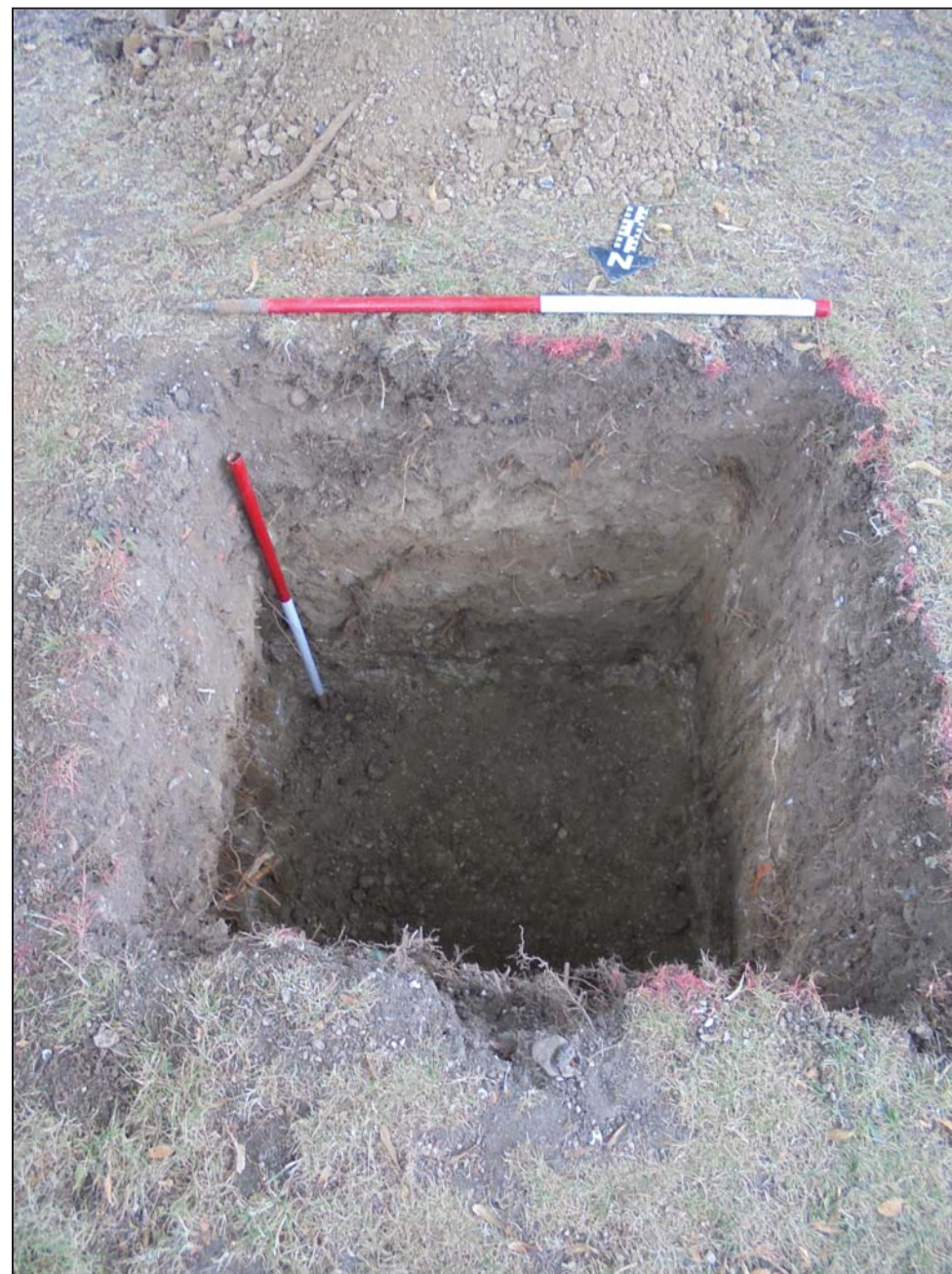
Baulk in Trench 2 soakaway, looking south-east (1m scales)
