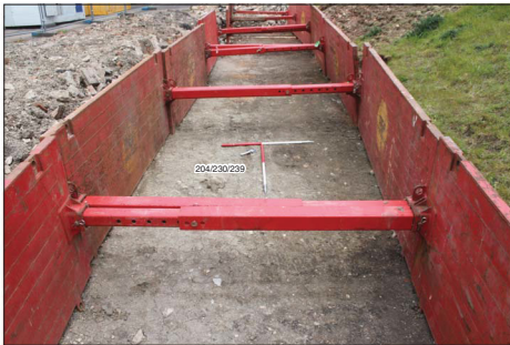
Clay 204/230/239, looking north-east (2 x 1m scales)
