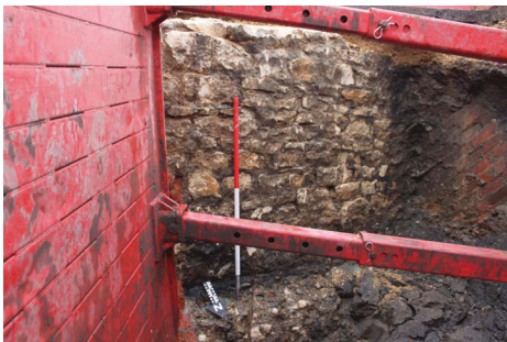
Wall 703, and brick-built buttness 717, looking south (1m scale)
