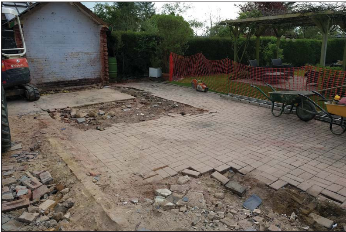
General view of area prior to works, facing north-east
