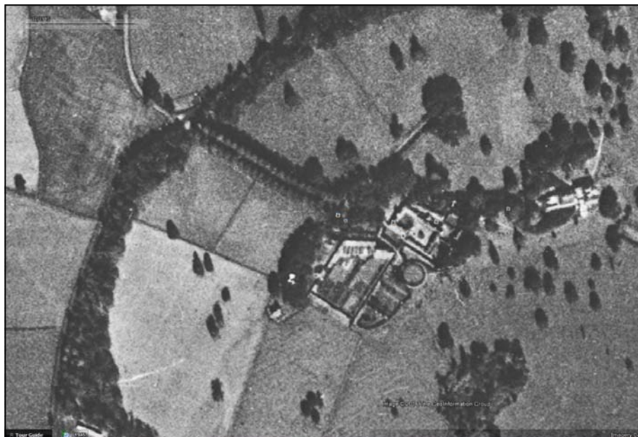
Fig 10. Aerial photograph of Coton House, 1945
