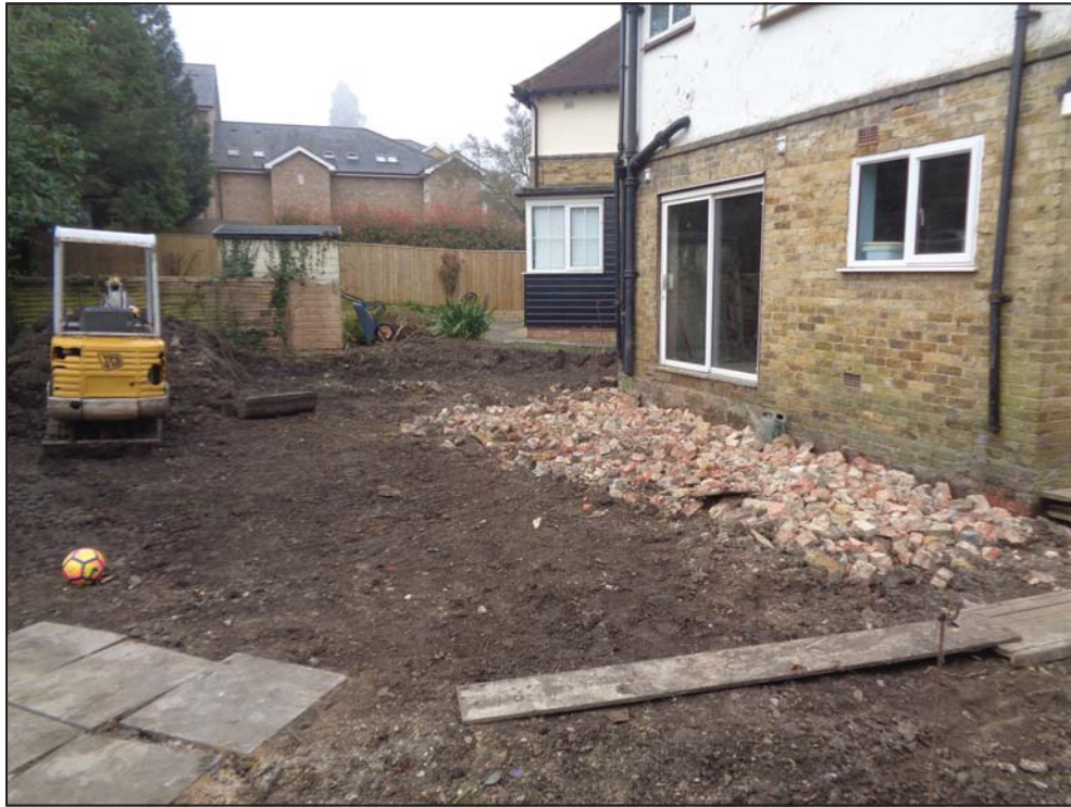
General view of site, looking southwest
