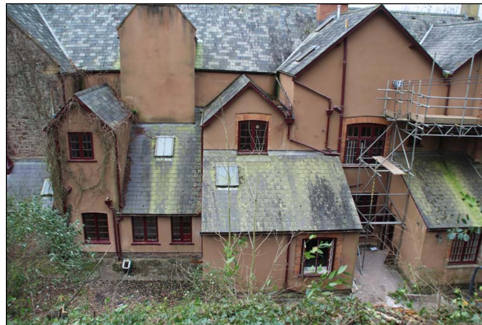
Figure 13: The north elevation of the house showing the rear ranges before demolition
