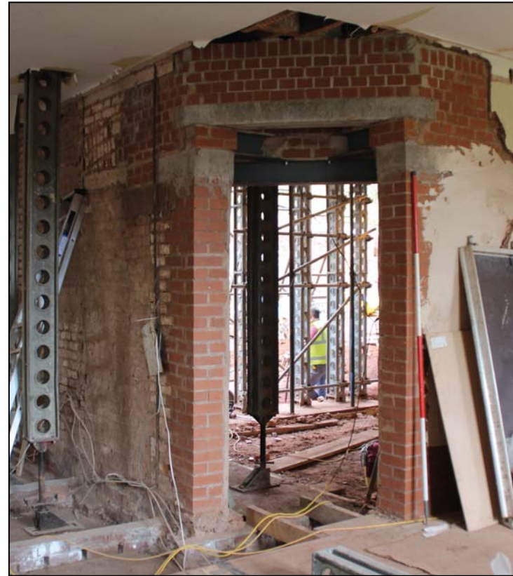
Figure 11: The wall between the rear part of the Games Room and the Kitchen, on left, looking north-east; note blocked doorway with half an arched head. 2017 doorway in centre (scale 2m)
