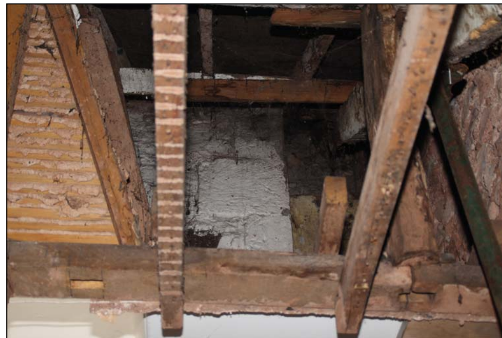
Figure 21: Looking south and up into the roof space of the eastern utility room through the 1930 ceiling joists to the skylight shaft, white painted timbers and hall stack
