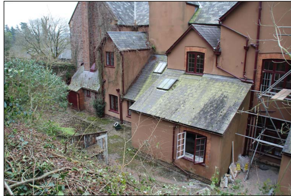
Figure 19: The east end of the rear range, looking south-east
