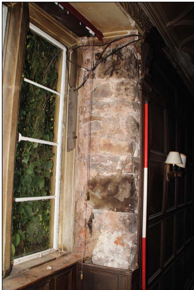
Figure 8: The northern reveal of the west-facing window in the Drawing Room (Oak Room) showing plaster behind panelling (scale in 0.5m divisions)
