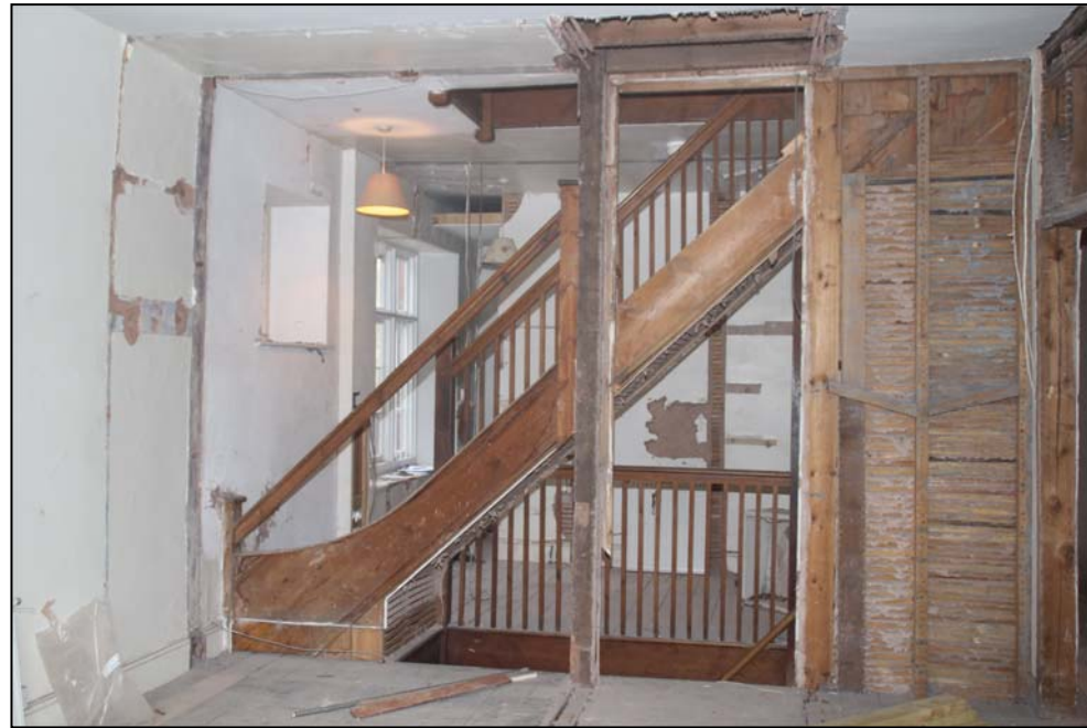
Figure 30: The stair inserted in 1930, first floor looking east
