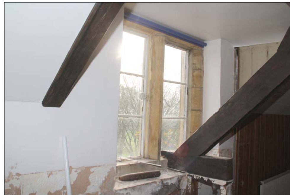
Figure 37: The foot of the eastern truss in the west wing, the later-truncated tiebeam rests on the window cill. Note simplified profile of mullions
