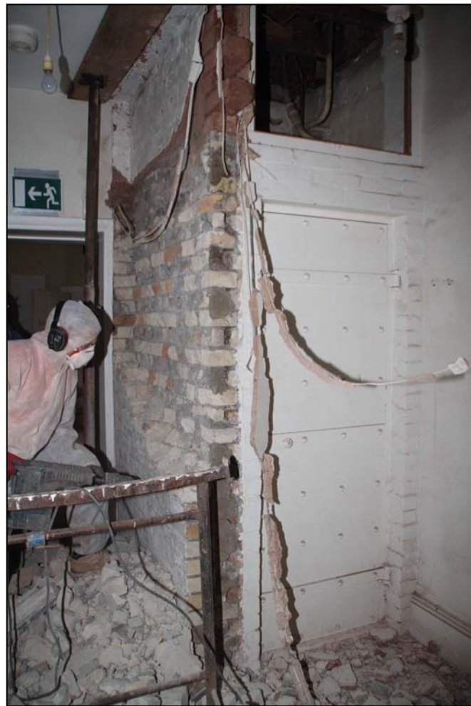
Figure 22: The silver safe during demolition, looking west
