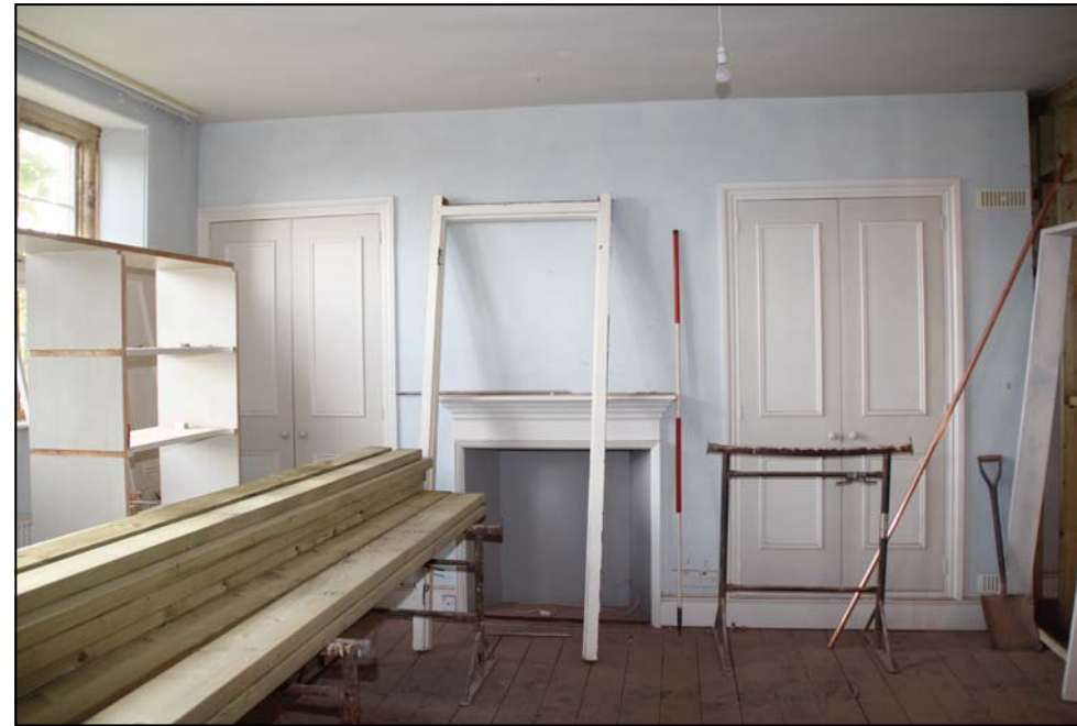
Figure 31: The west wall of Bedroom 5
