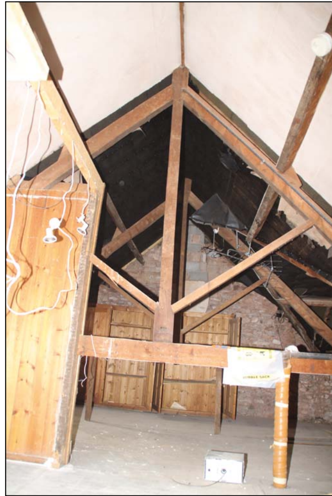
Figure 38: The central and western trusses of the west wing, looking west
