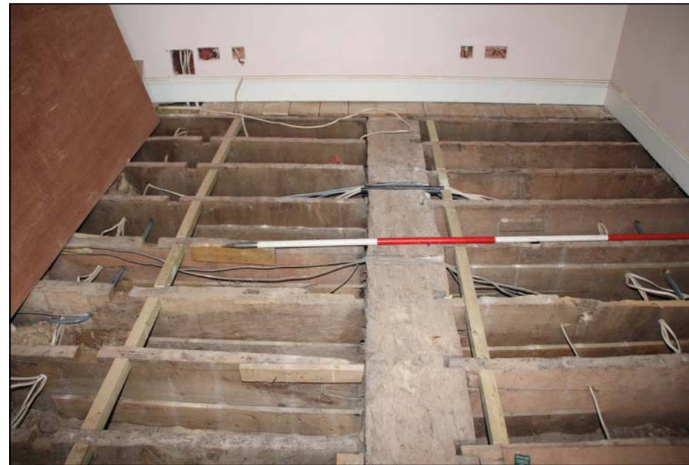
Figure 33: The transverse beam and joists in Bedroom 8, looking north (scale 2m)
