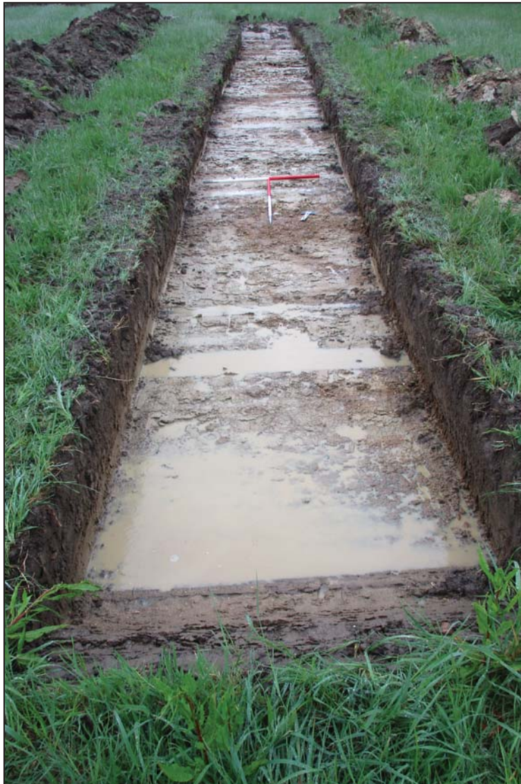
Trench 6, looking north-west (scales 1m)
