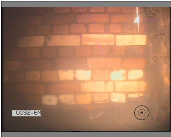
Photo: 2_3A, 00:02:52 32.6m, Finish node type, manhole reference number: CAP END
