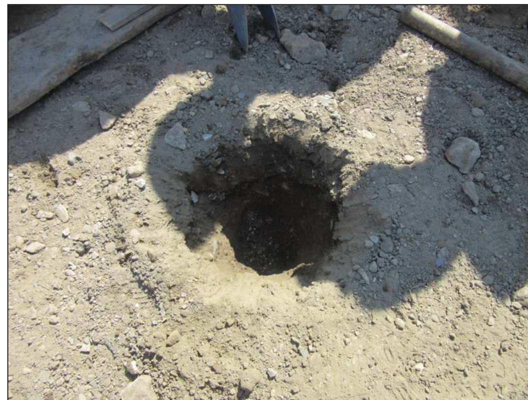
Borehole Test Pit 7
