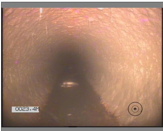
Photo: 4_7A, 00:02:21 23.4m, Material changes, cast iron
