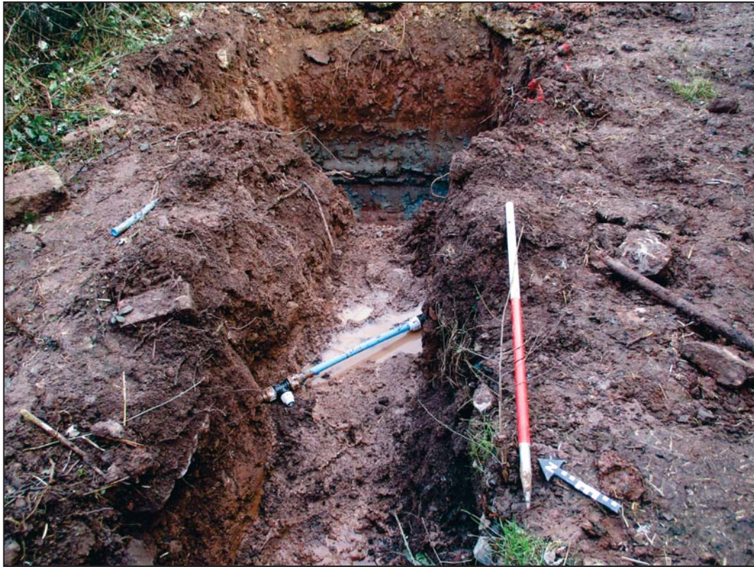
Trench 1, looking north-east (1m scale)
