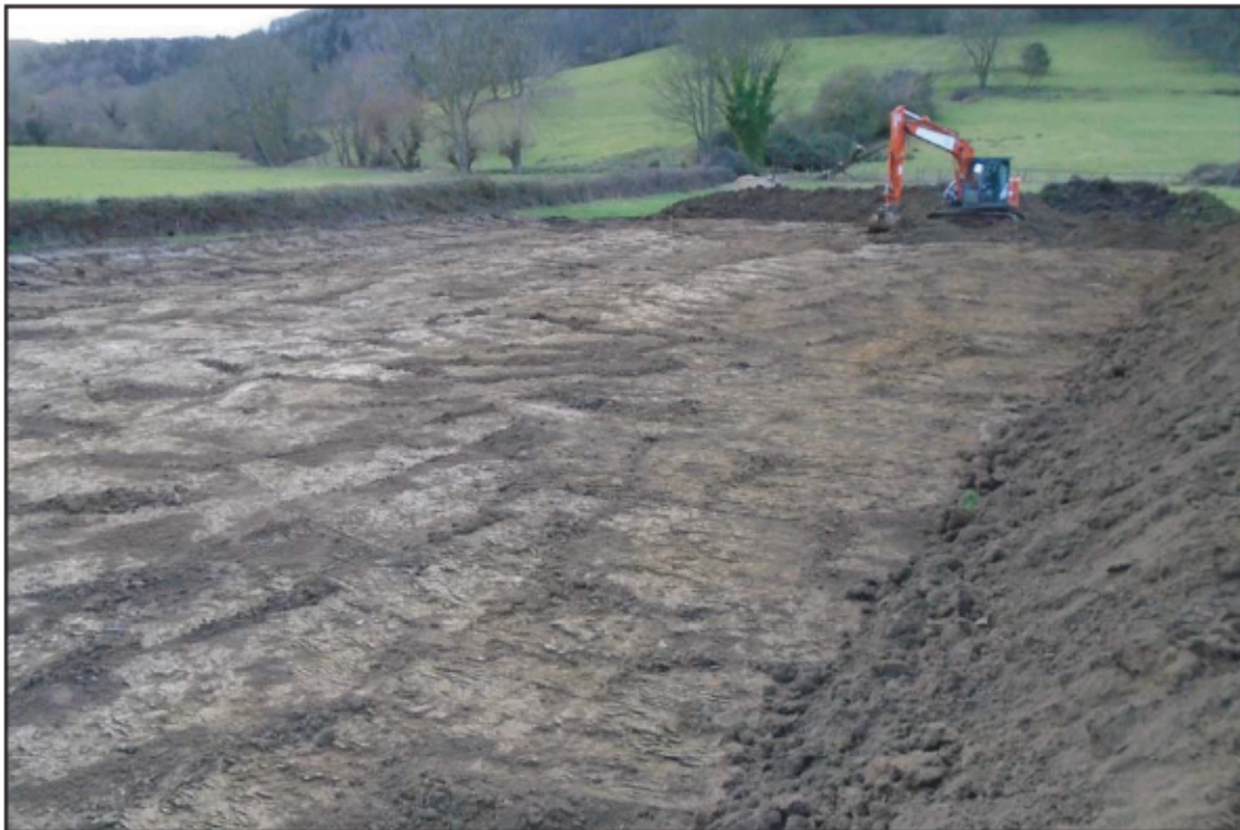
The site, looking south-west
