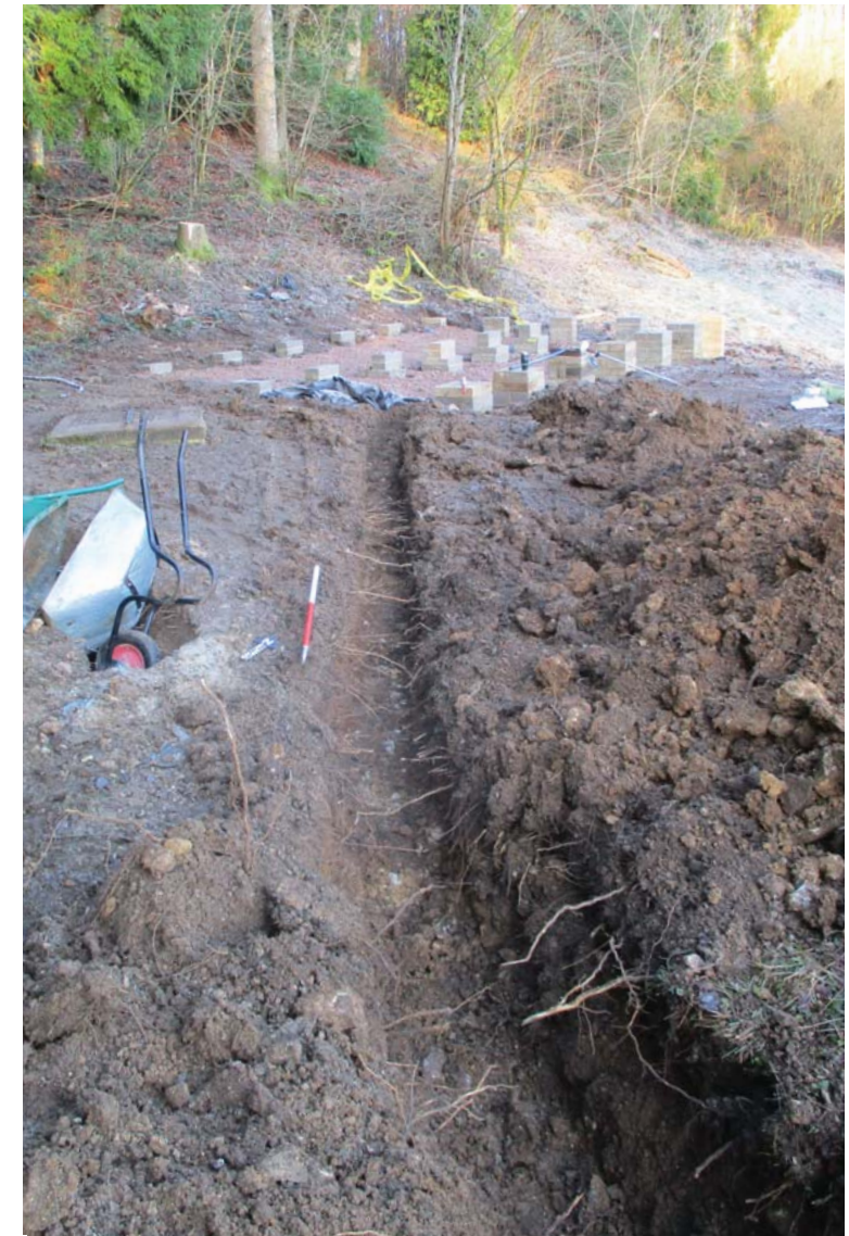
Excavated foundation trenches and service trench, looking north-west (1m scale)
