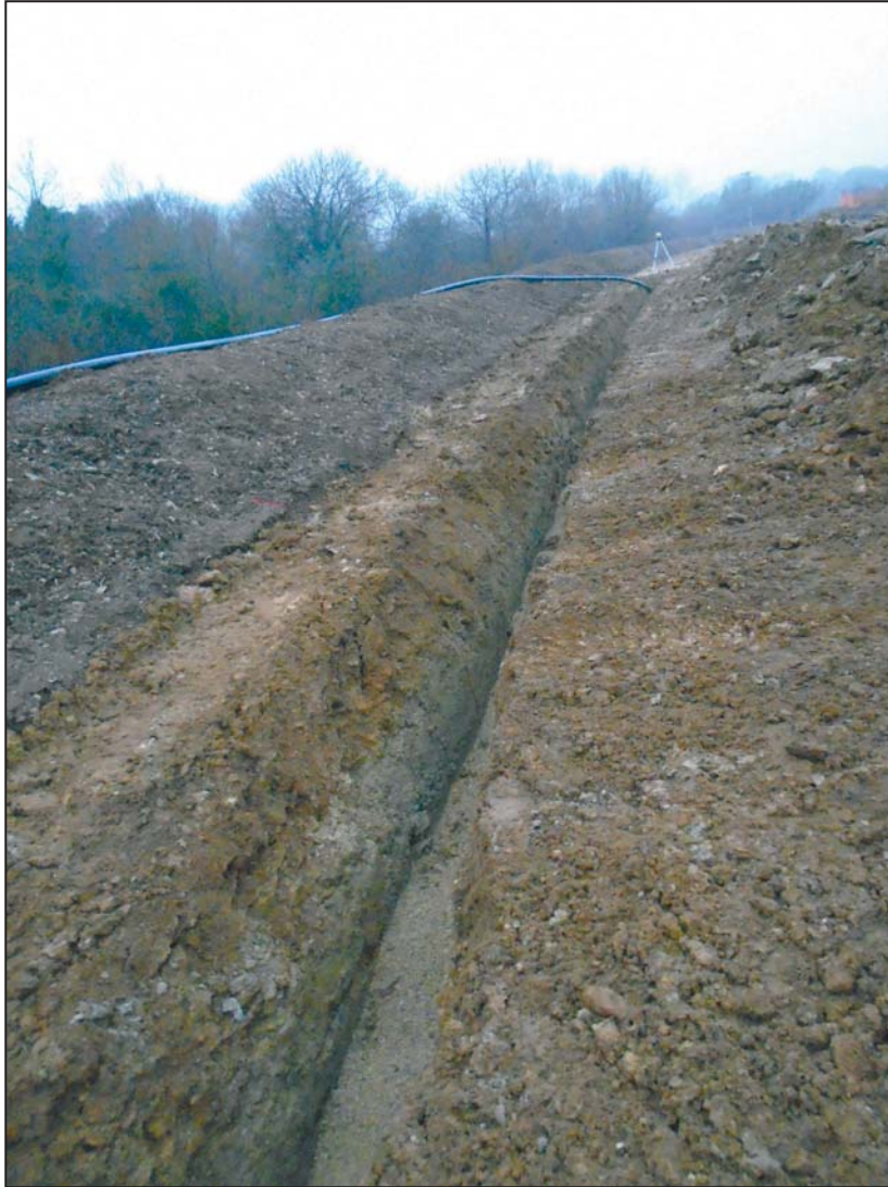
Area 3 (New Rising Main Route), looking north-west
