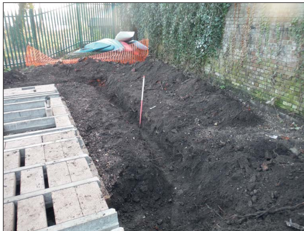
Trench 1, looking south-east (scale 1m)
