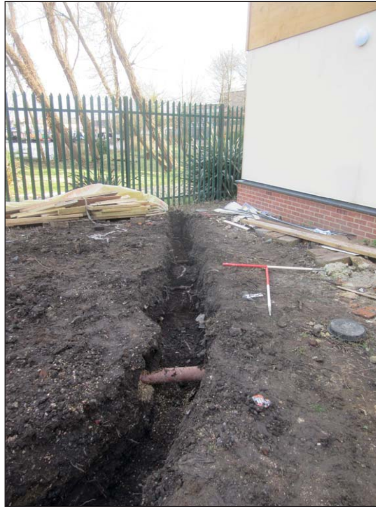
Trench 2, looking east (scales 1m)
