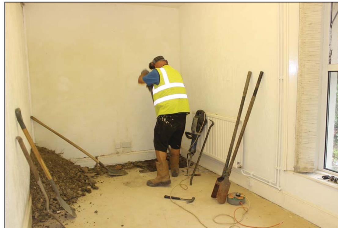
Test Pit 6, working shot
