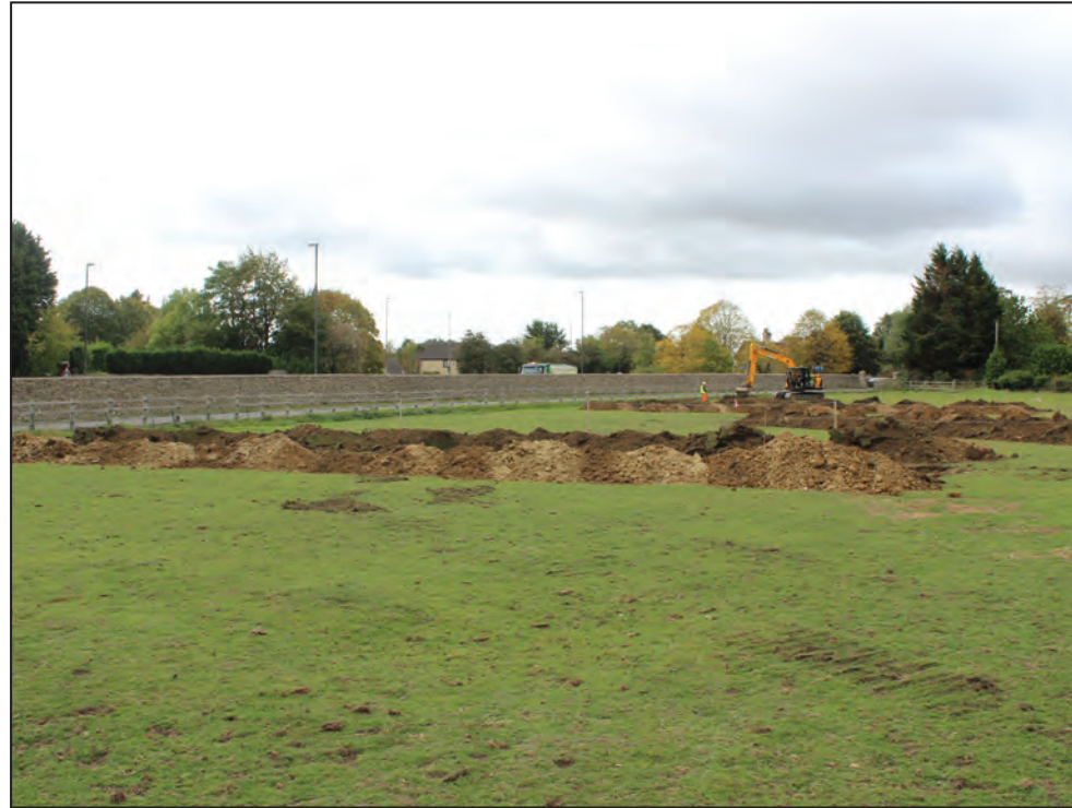
General view of site, looking south-west
