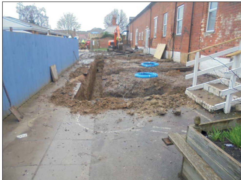
Working photograph of trench 4, looking west
