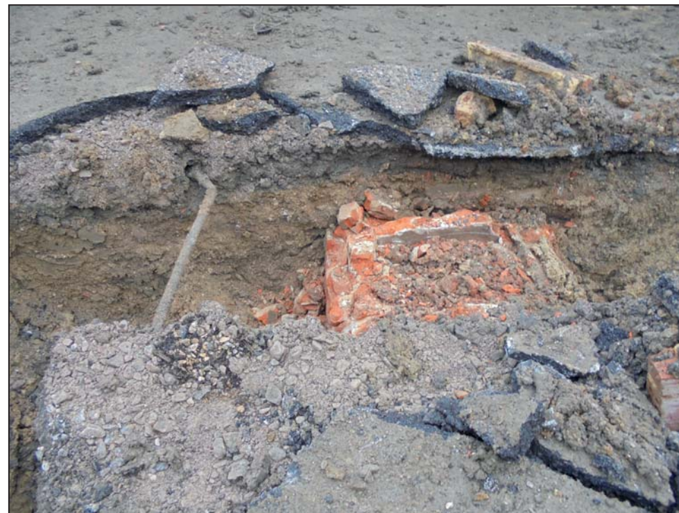
Working photograph of foul sewer
