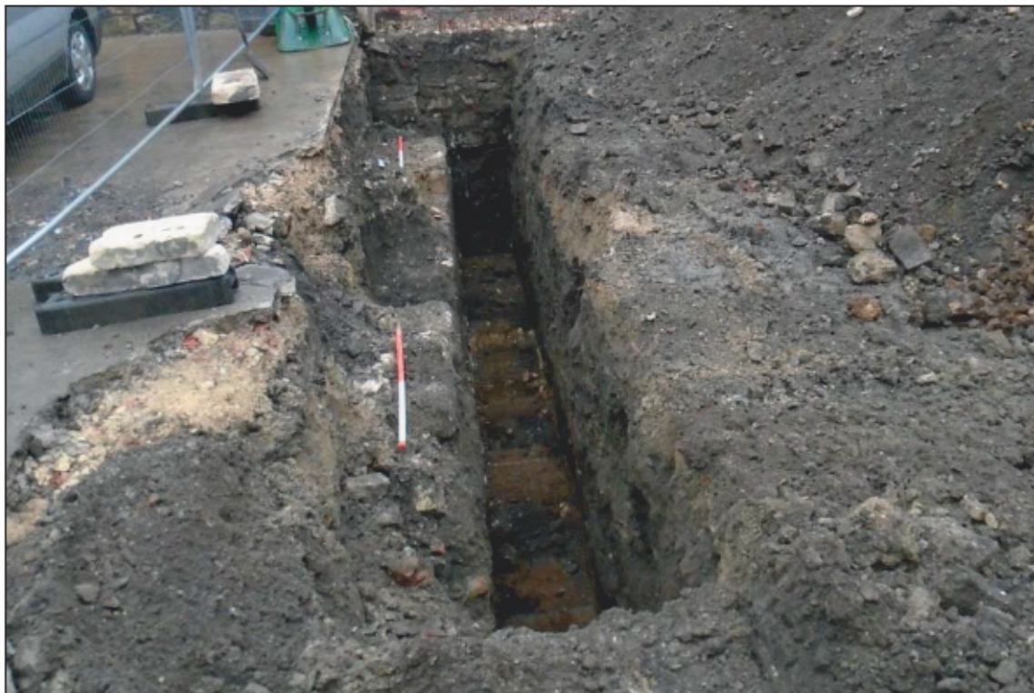
Wall 108, looking north (scales 1m)
