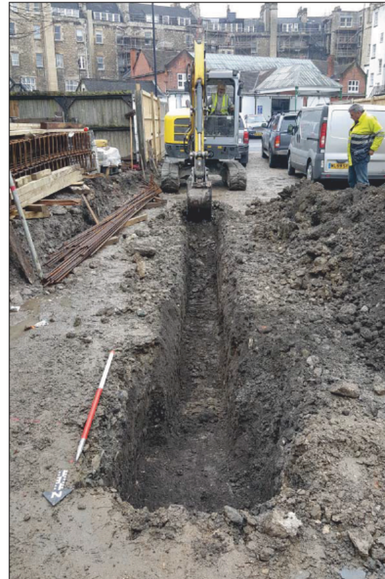
The site showing excavated drainage trench 2, looking south (scale 1m)
