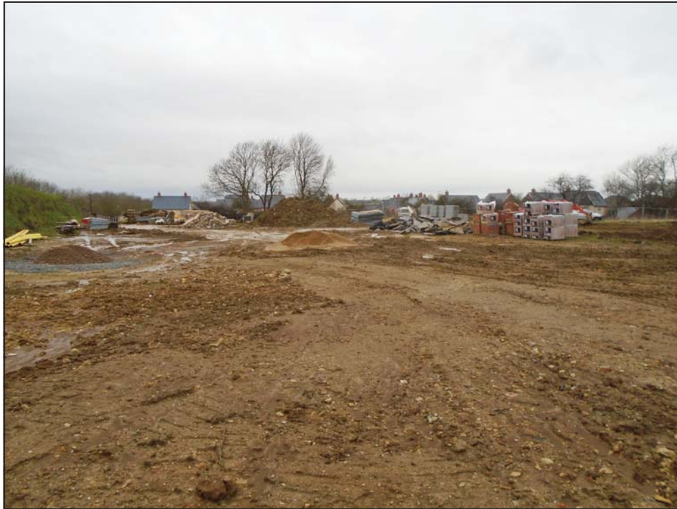
Pre-excavation photograph of south of the site
