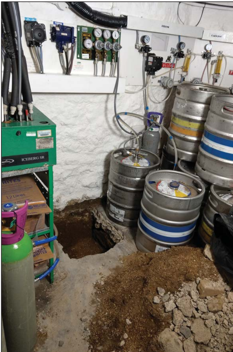
Sump location in basement, looking west
