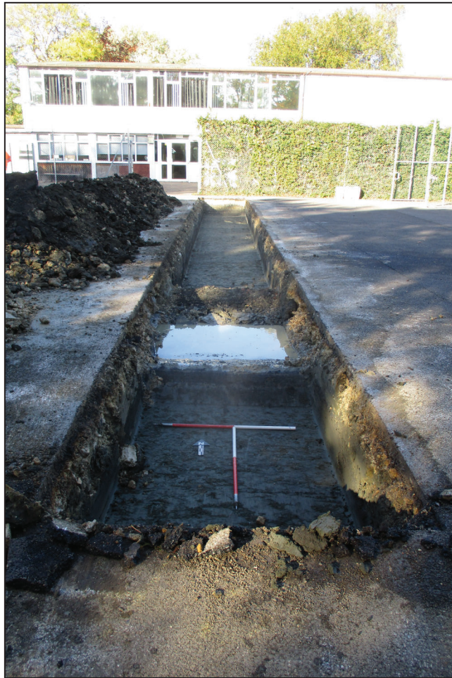
Trench 19, looking north (1m scales)
