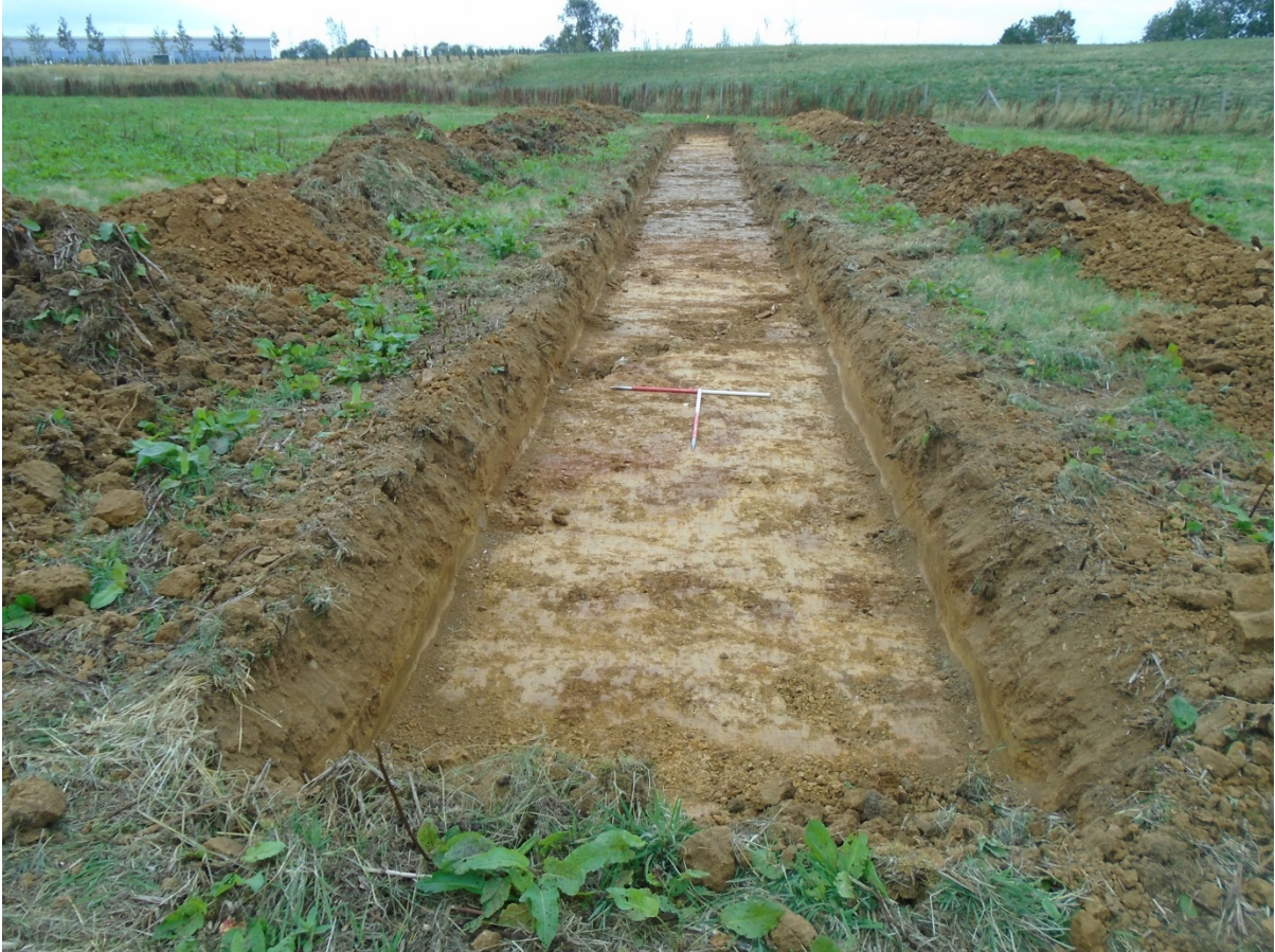
Plate 6, Trench 4, looking west (1m scales)
