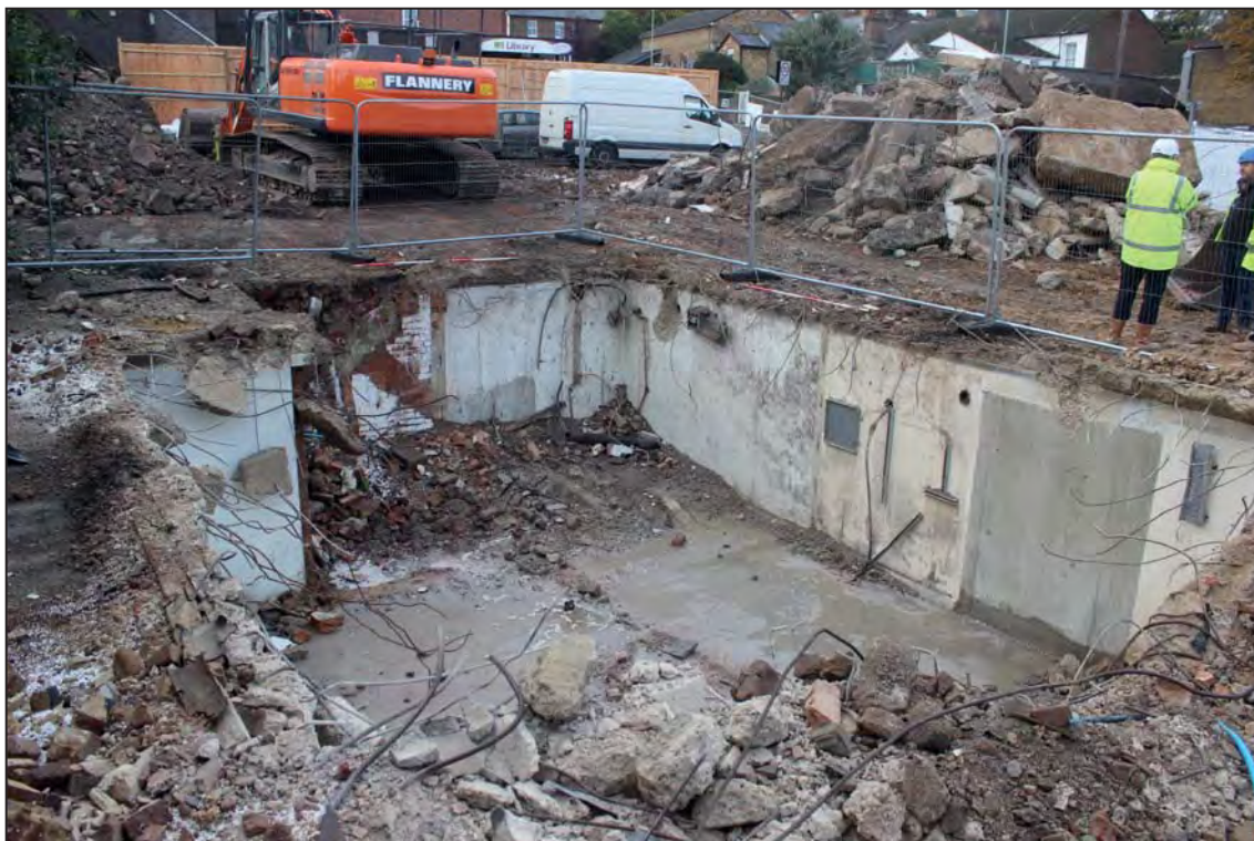
Trench 7, looking south-west (2m scales)
