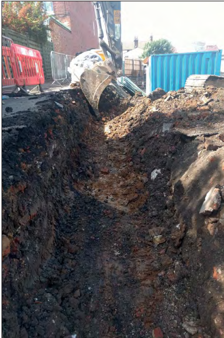
Trench 14, looking north-west
