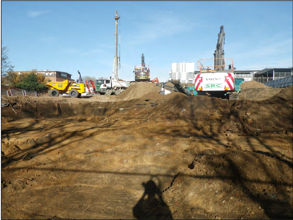
Plate 1. Contractors stripping the eastern half of the site. Looking north
