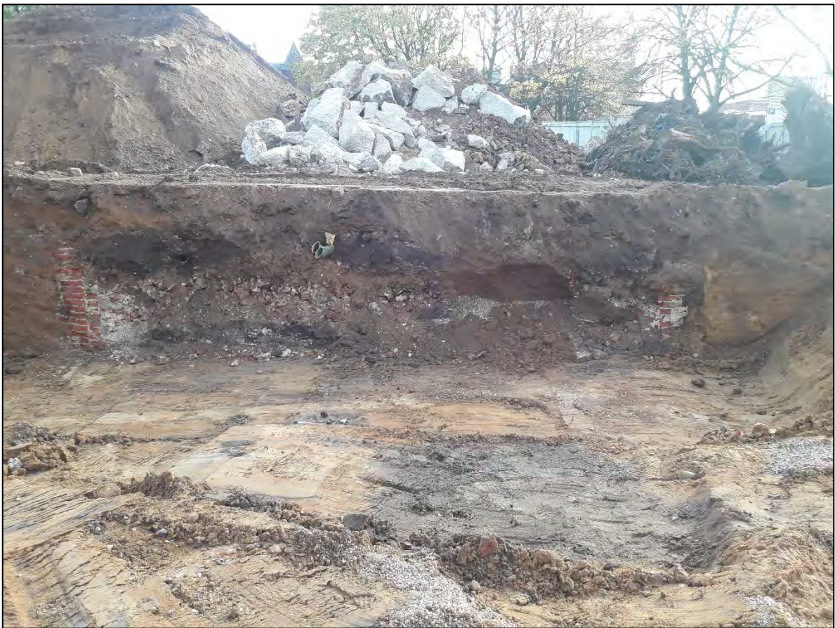
Plate 20. Remains of cellar 0088 in edge of machine strip. The western half of the cellar has been machined away. Looking east
