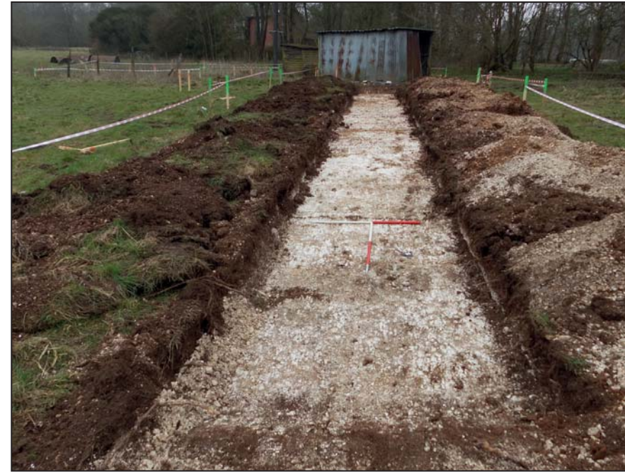
Trench 2, looking south-west (scales 1m)
