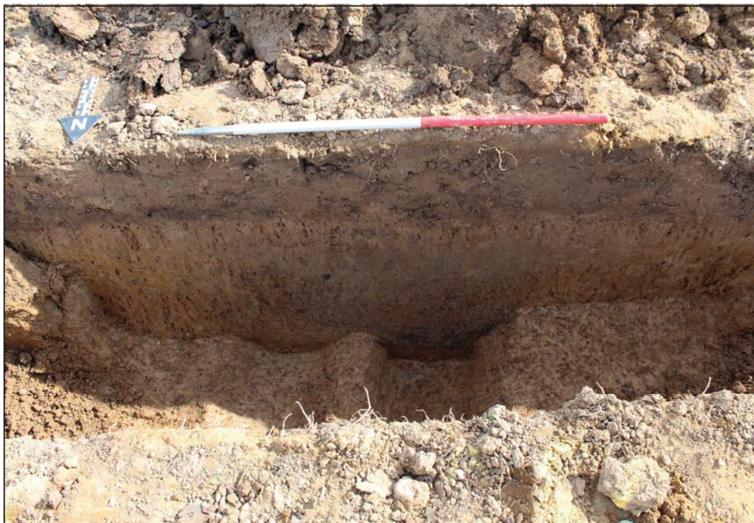
Ditches 2229 and 2230, looking south (1m scale)
