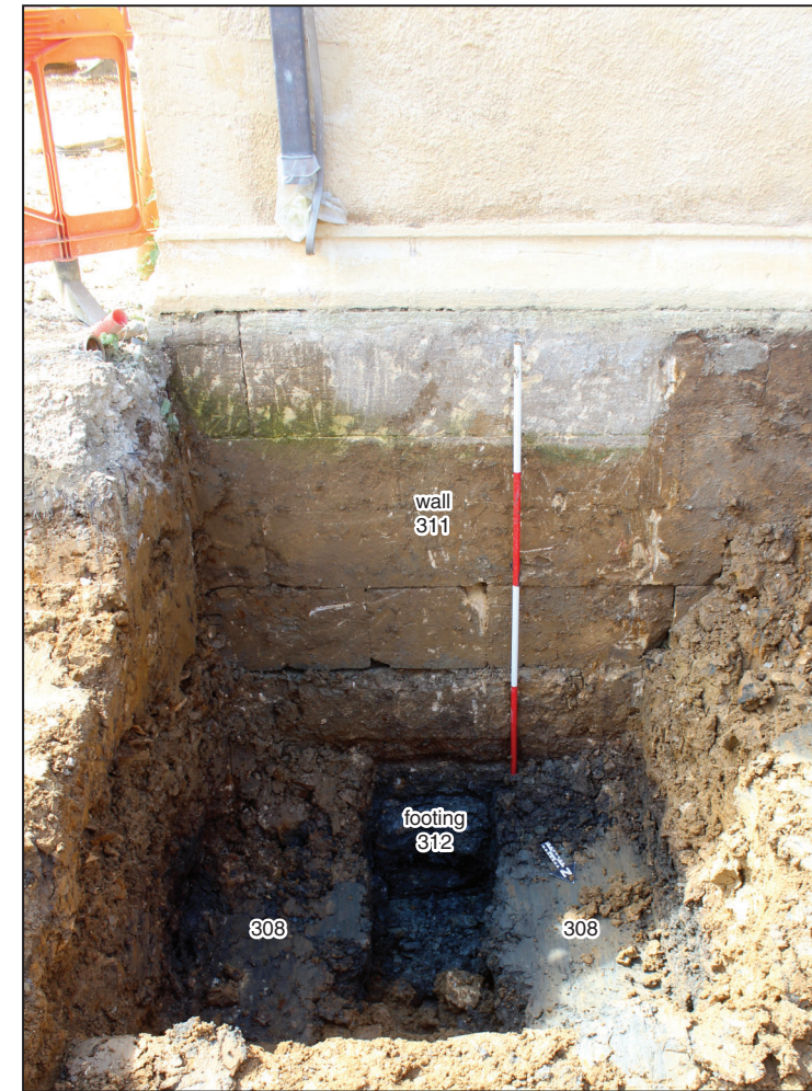
Wall footing 312 and wall 311, looking south-west (2m scale)
