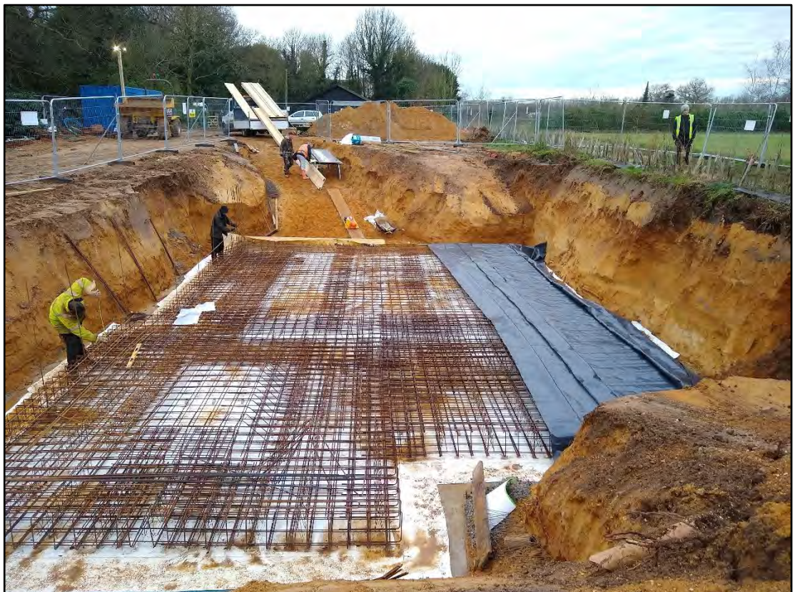
Plate 3: Garage construction hole, looking south-west
