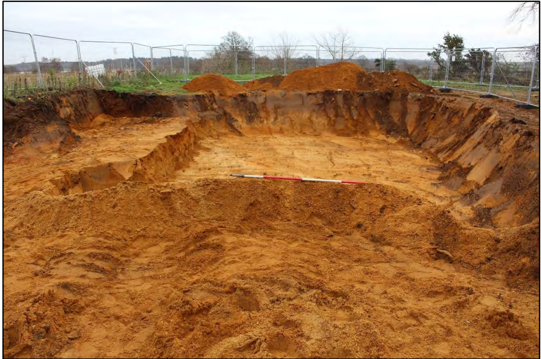
Plate 2: Garage construction hole, looking north-east, 1x2m scale
