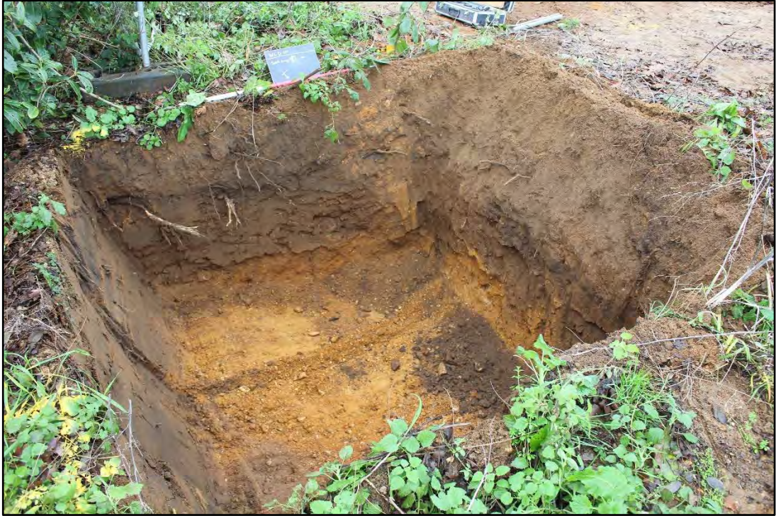
Plate 7: Soakaway 2, looking south-west, 1x1m scale
