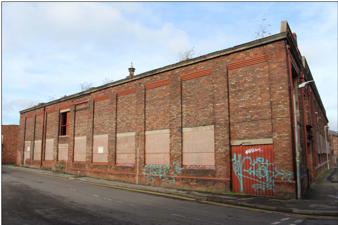
Photo 16: An overview of Elevation 2 from the south-east.
