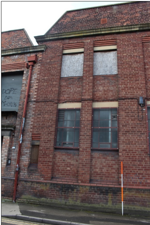
Photo 22: Detail of metal framed windows to Elevation 3.
