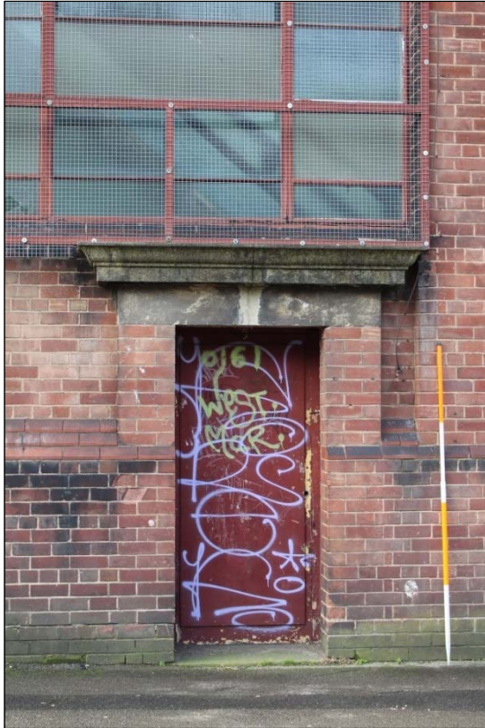
Photo 25: Detail of a door opening at the northern extent of Elevation 3.
