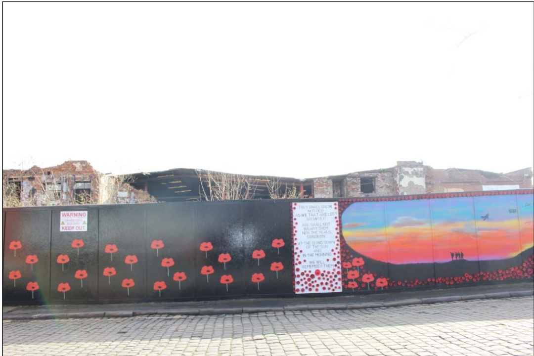
Photo 26: An overview of Elevation 6 from the north-west.
