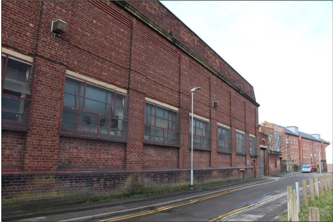
Photo 21: An overview of the northern extent of Elevation 3 from the south-east.
