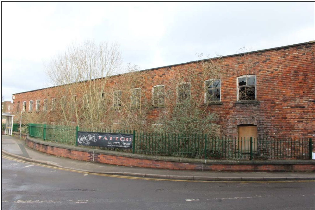
Photo 3: An overview of Elevation 1 from the south.
