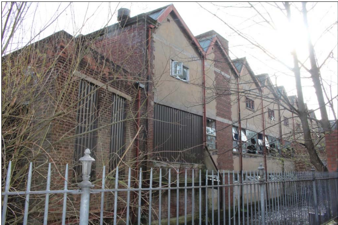
Photo 28: An overview of Elevation 7 from the north-west.
