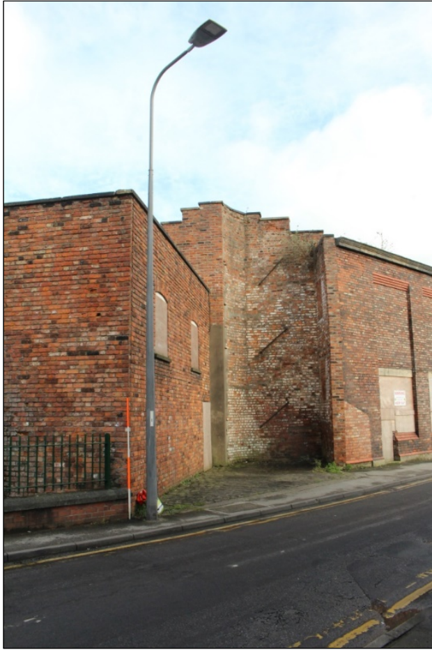
Photo 12: An overview of the stair turret from the south-west.
