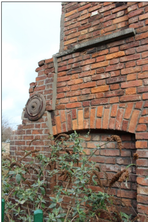
Photo 7: Detail of window opening and tie plate at the northern extent of Elevation 1.
