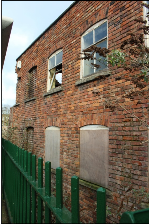
Photo 6: An overview of the northern extent of Elevation 1 from the south.
