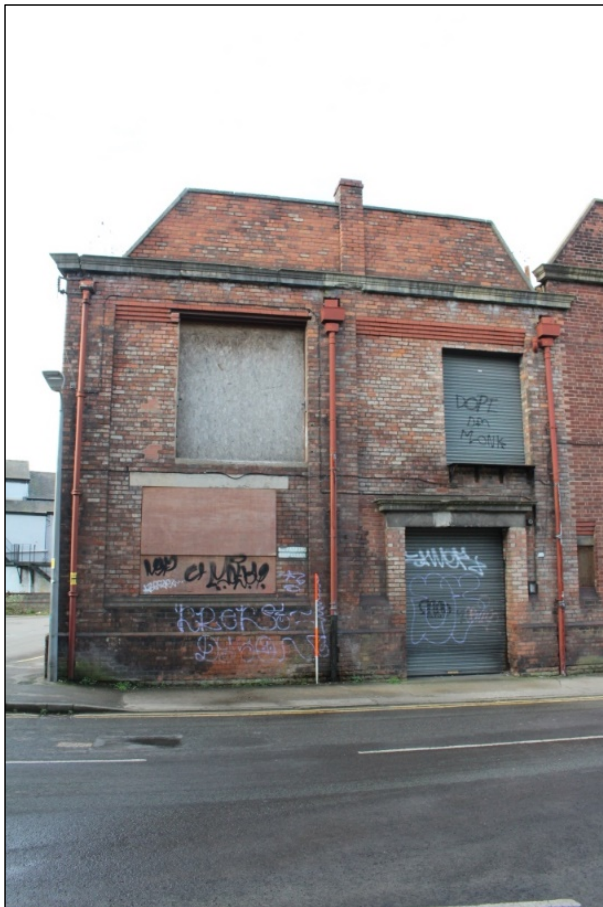
Photo 18: An overview of the southern extent of Elevation 3 from the south-east.
