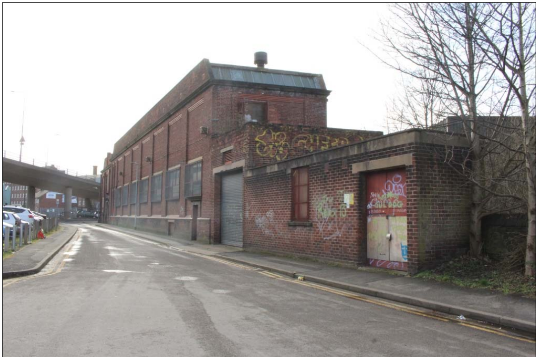
Photo 24: An overview of Elevations 3 and 4 from the north-east.
