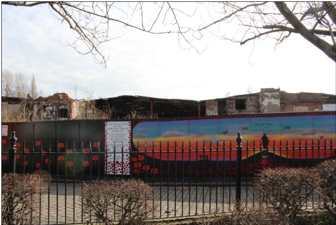
Photo 27: An overview of Elevation 6 from the north-west.
