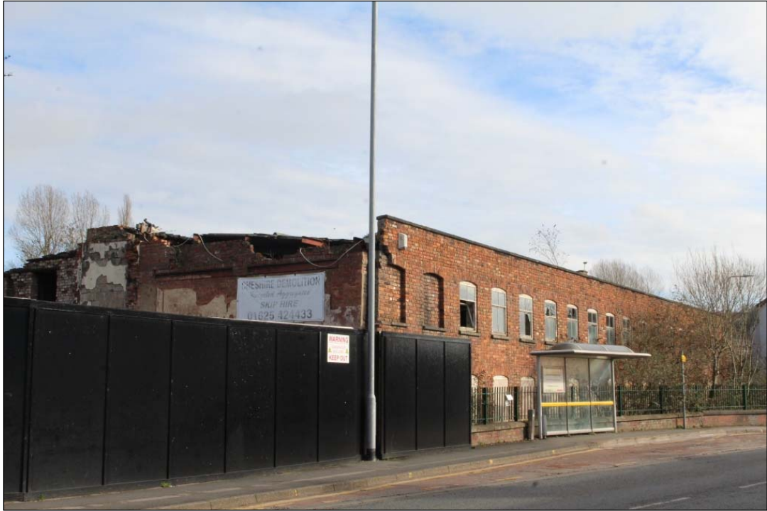
Photo 2: An overview of Elevation 1 from the north-west.
