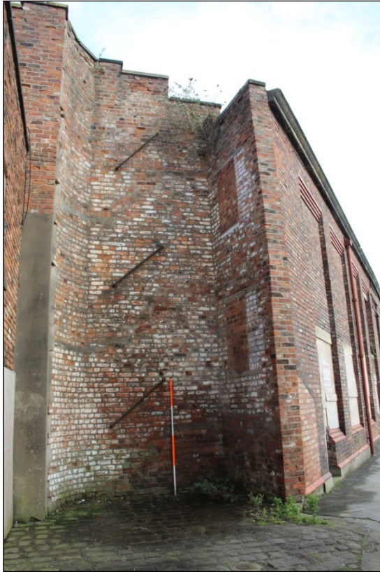
Photo 13: Detail of the stair turret from the south-west.
