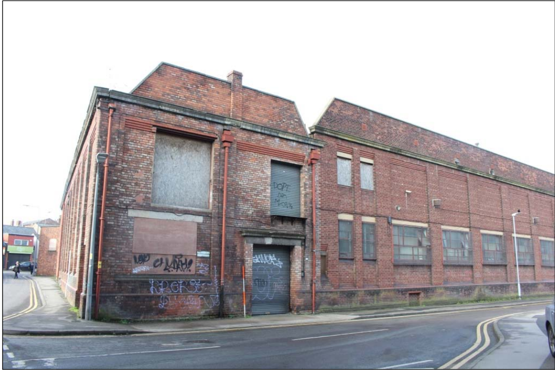
Photo 17: An overview of Elevation 3 from the south-east.
