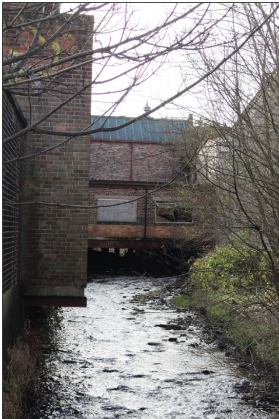
Photo 30: Detail of Elevation 8 from the bridge over the River Bollin.
