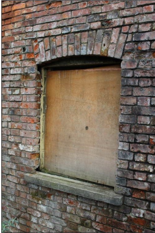
Photo 4: Detail of a brick soldier arch window opening within Elevation 1.
