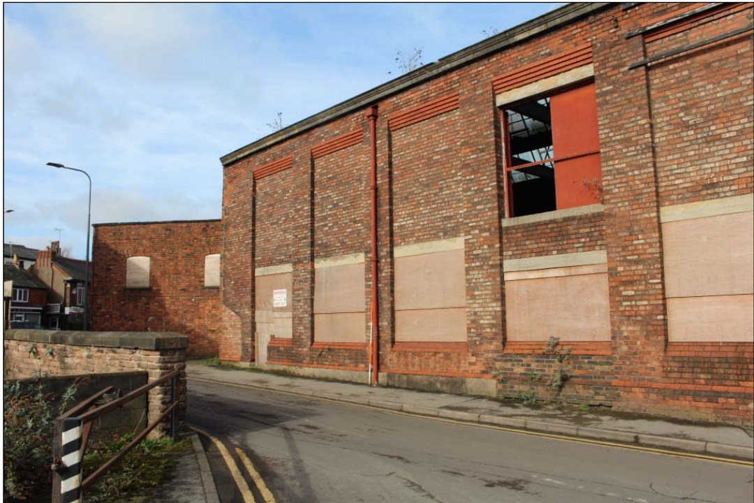
Photo 15: An overview of Elevation 2 from the south-east.
