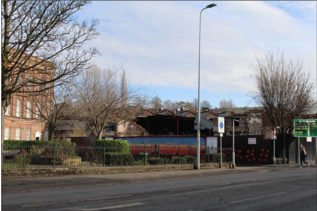
Photo 1: An overview of the site from the north-west.
