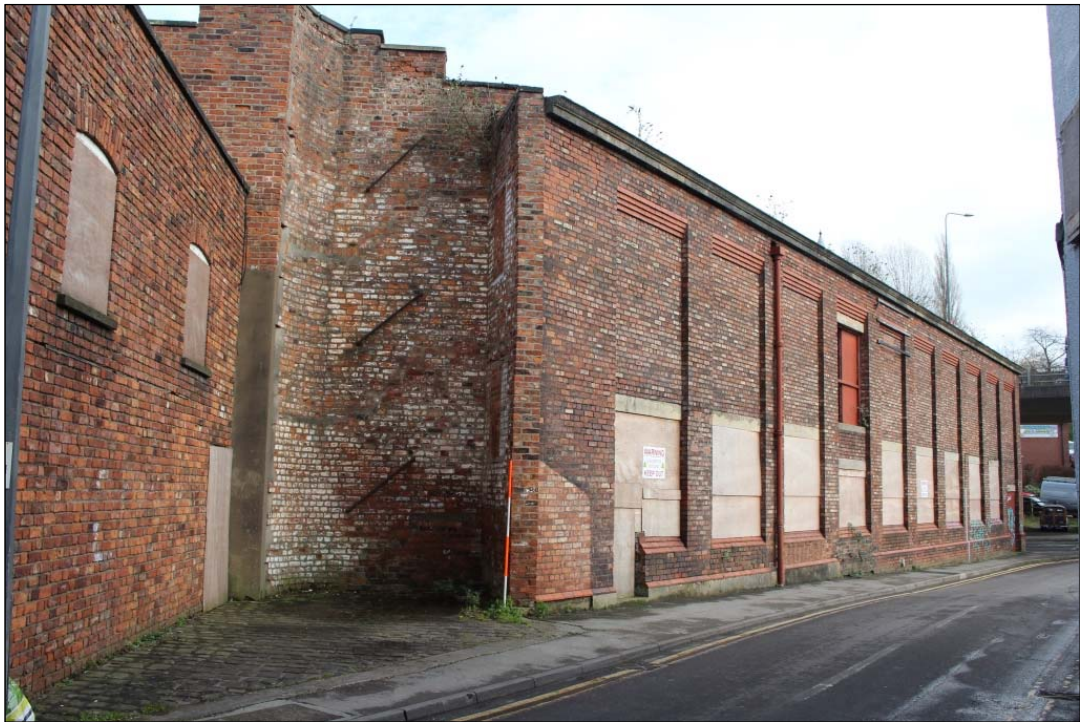
Photo 11: An overview of Elevation 2 from the south-west.
