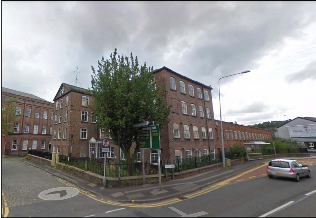
Figure 4: An extract of Google Street View Imagery (2009) showing Elevation 1 alongside the now demolished Park Green Range.
