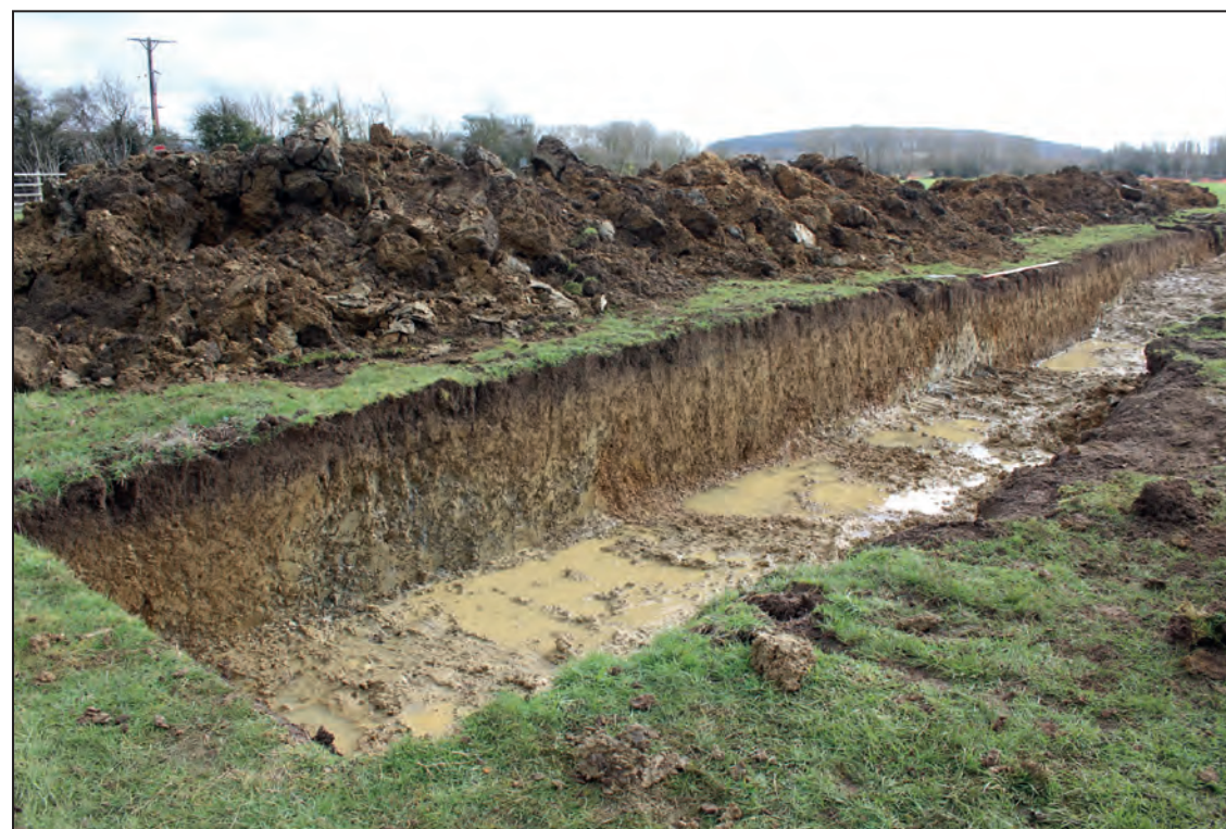
Section AA, looking north-east (2m scale)
