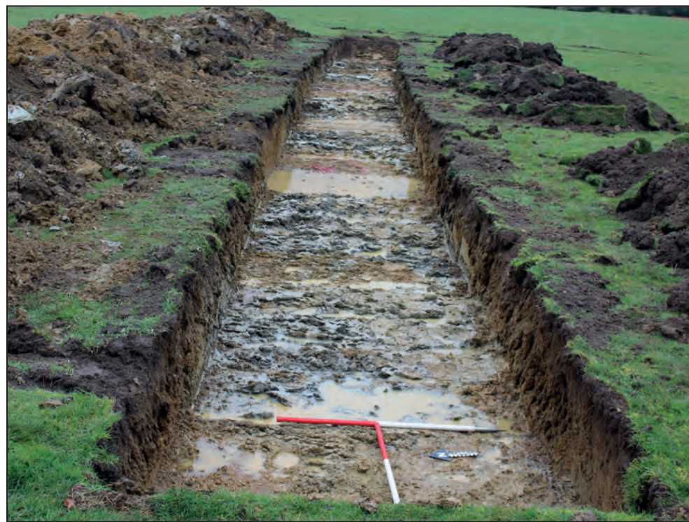
Trench 2, looking south-east (1m scales)
