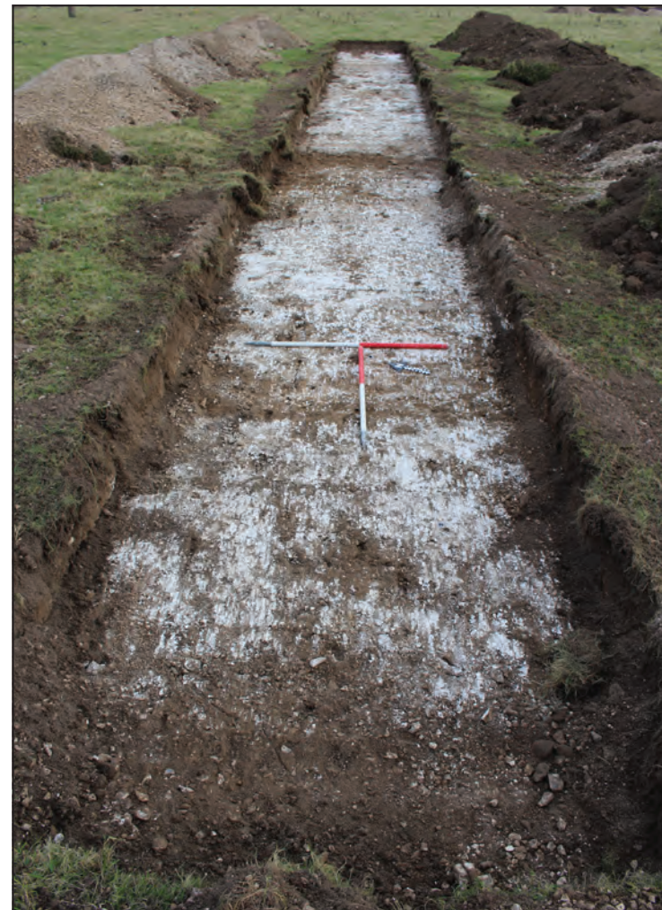
View of trench 35, looking north-east (1m scales)
