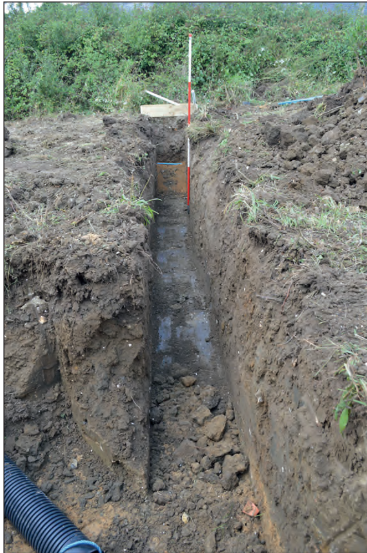
Service trench (north-east portion), looking north-west (2m scale)
