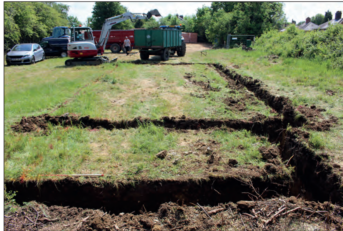
All monitored footing trenches, looking south-east (1m scale)
