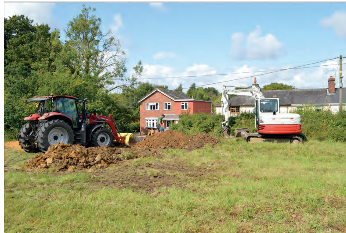
Service trenches being excavated, looking west
