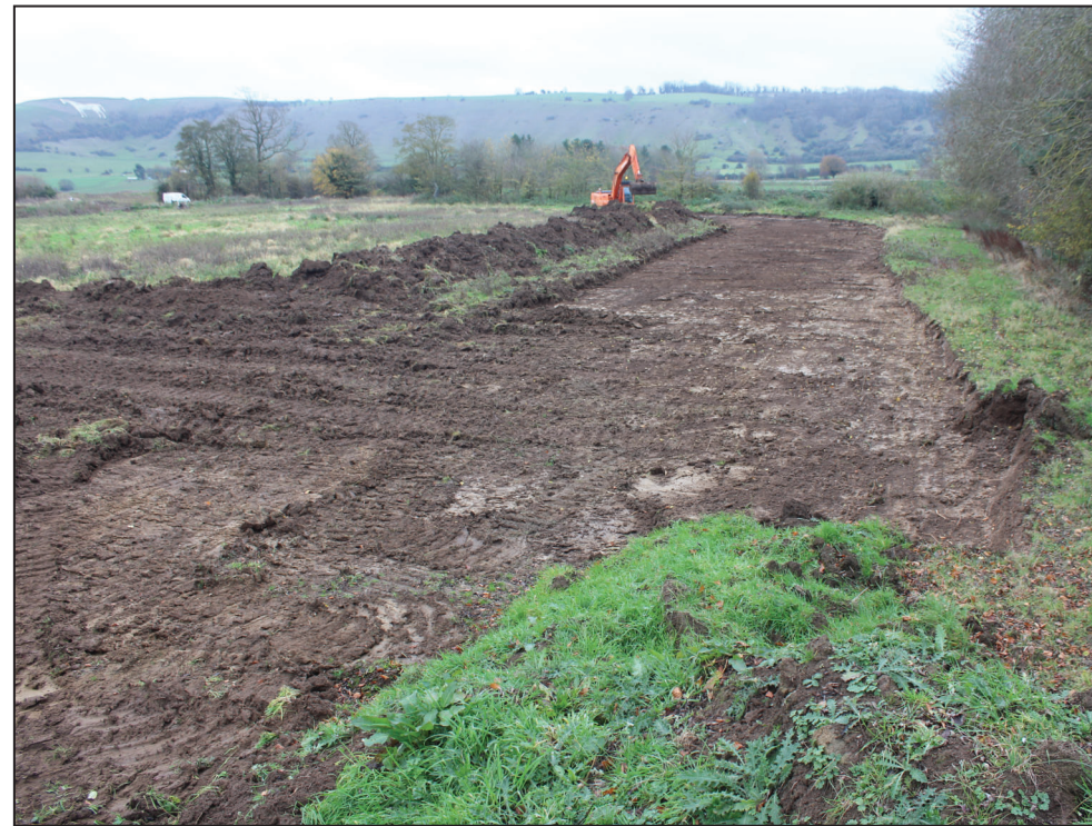
General view of excavated area, looking south-east
