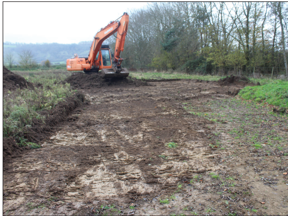
General view of excavated area, looking south
