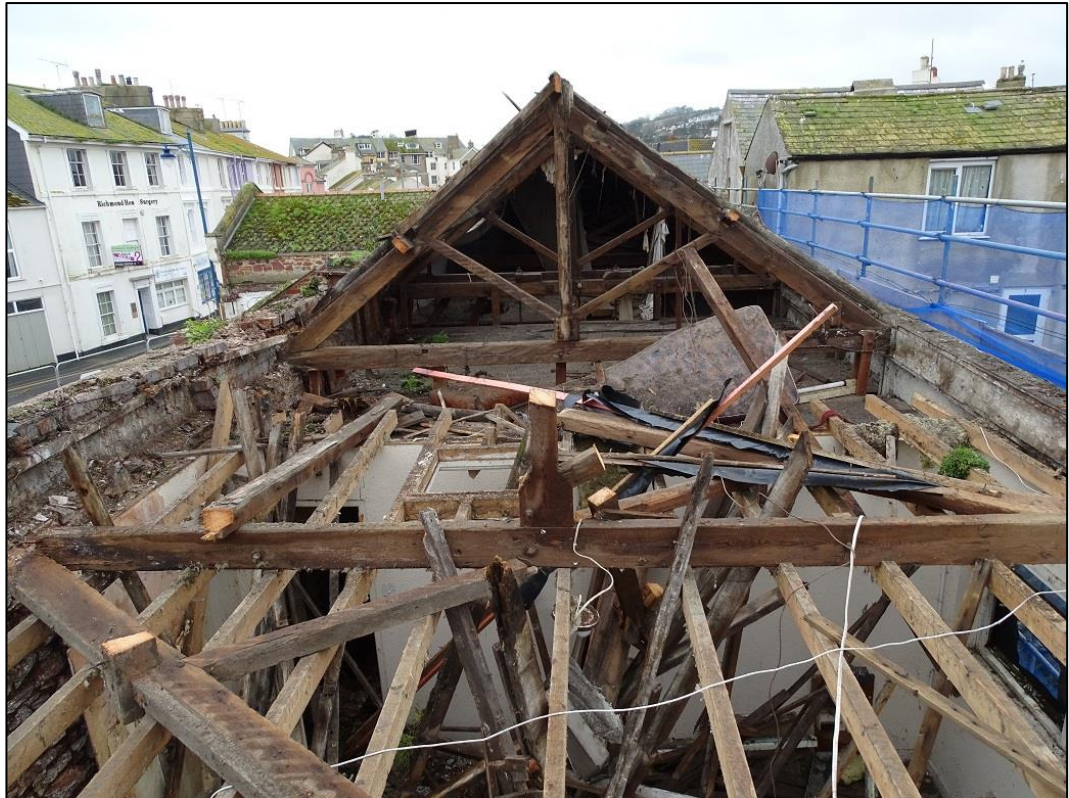
Photo 19: Demolition of the roof from the north elevation of the Building
