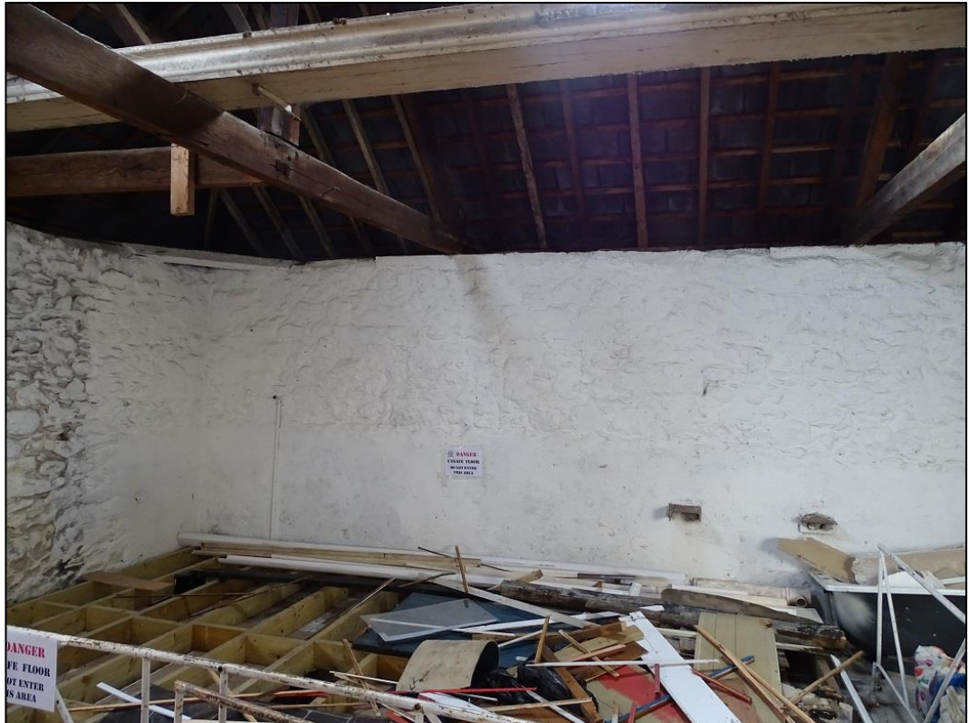
Photo 18: Interior of the Building at its first-floor south aspect looking south
