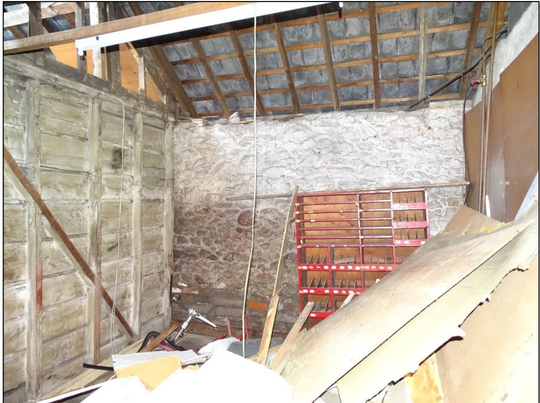
Photo 15: Interior of the Building at its first-floor north aspect looking east
