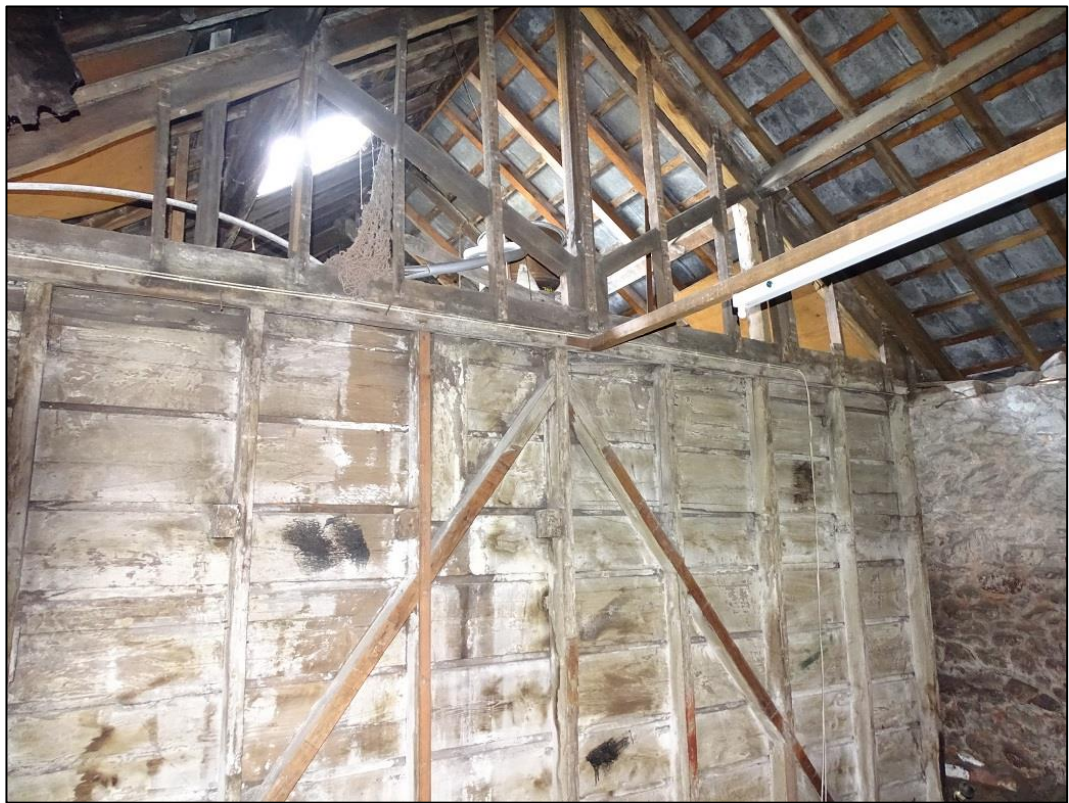
Photo 14: Interior of the Building at its first-floor north aspect looking north
