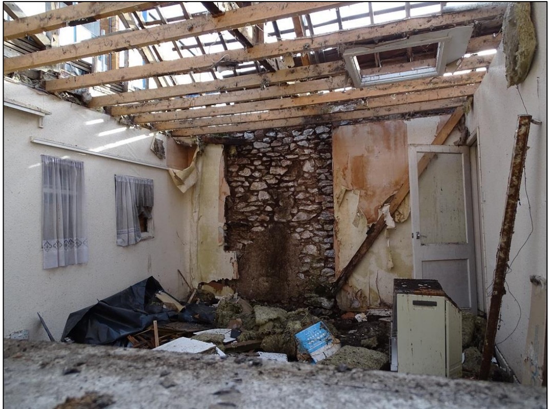
Photo 17: Interior of the Building at its first-floor north aspect looking south
