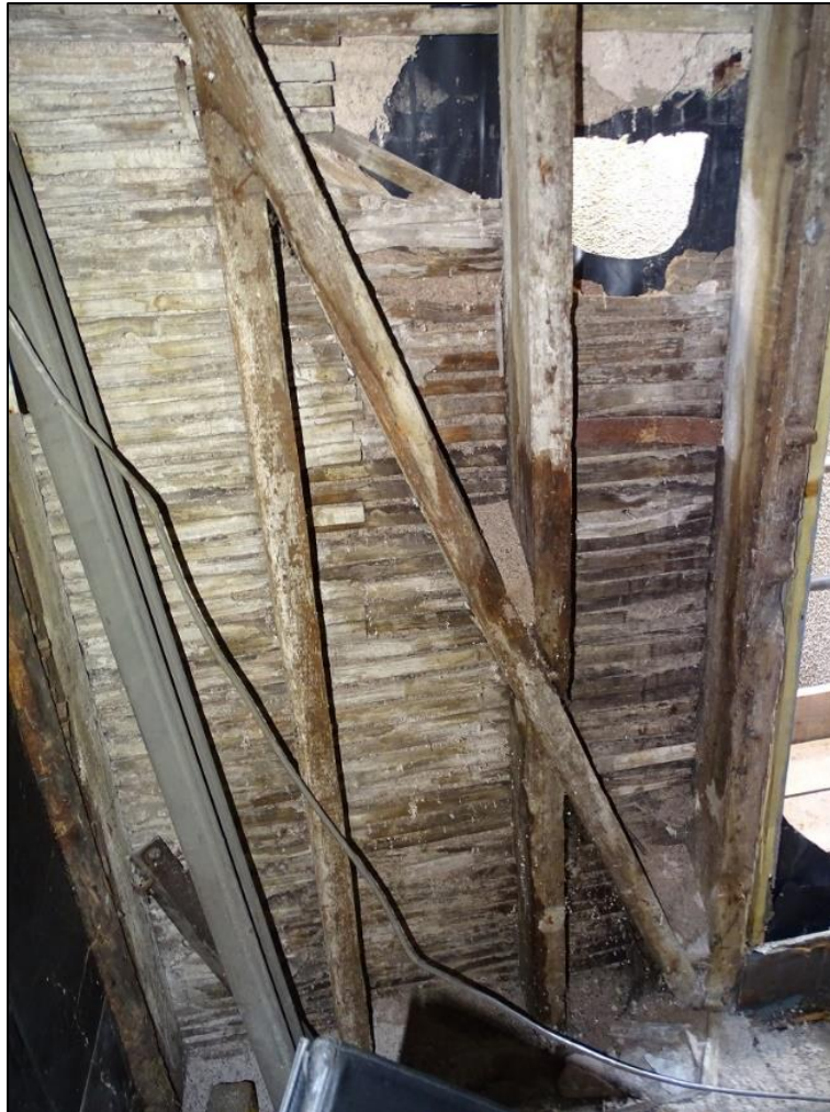
Photo 16: Interior of the Building at its first-floor north aspect looking west
