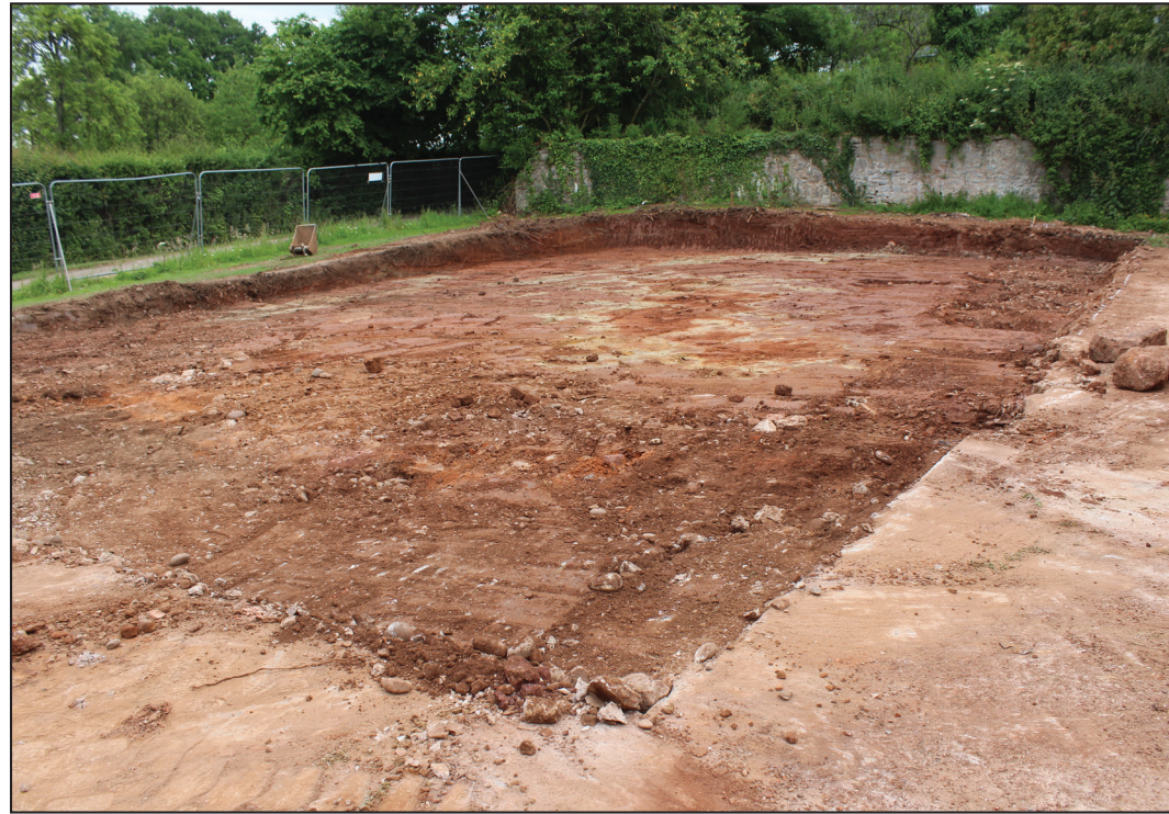
General shot of the site following ground reduction, looking south-east
