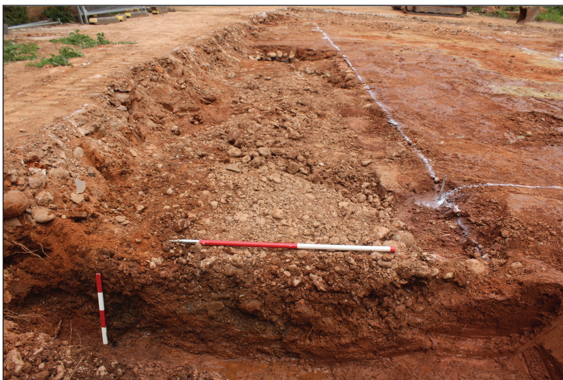
Section through foundation 104 and possible stream 105, looking north (0.4m and 1m scales)
