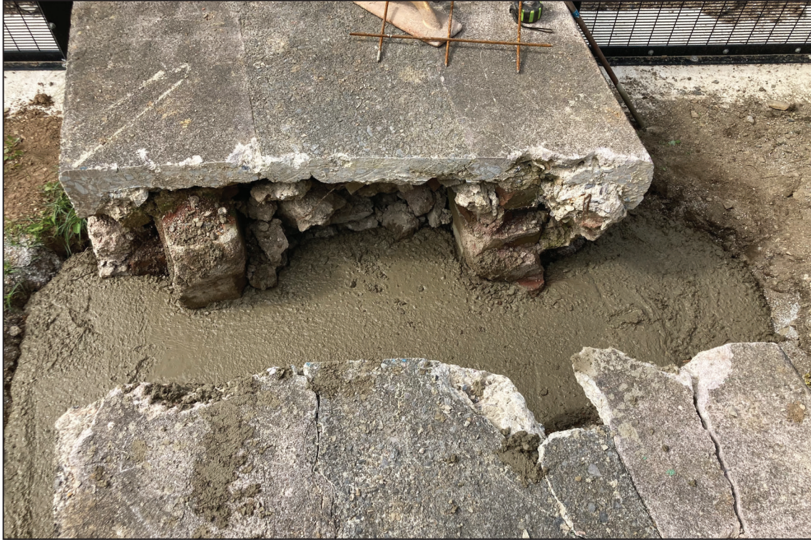
Infilling of concrete above mesh
