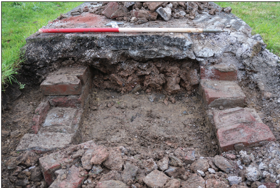
Trench 3: tramway pier structures 301 and 302, looking north-east (1m scale)
