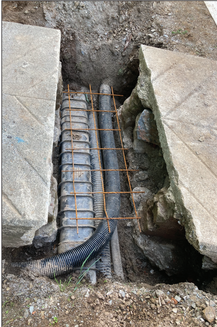
Iron mesh laid over services
