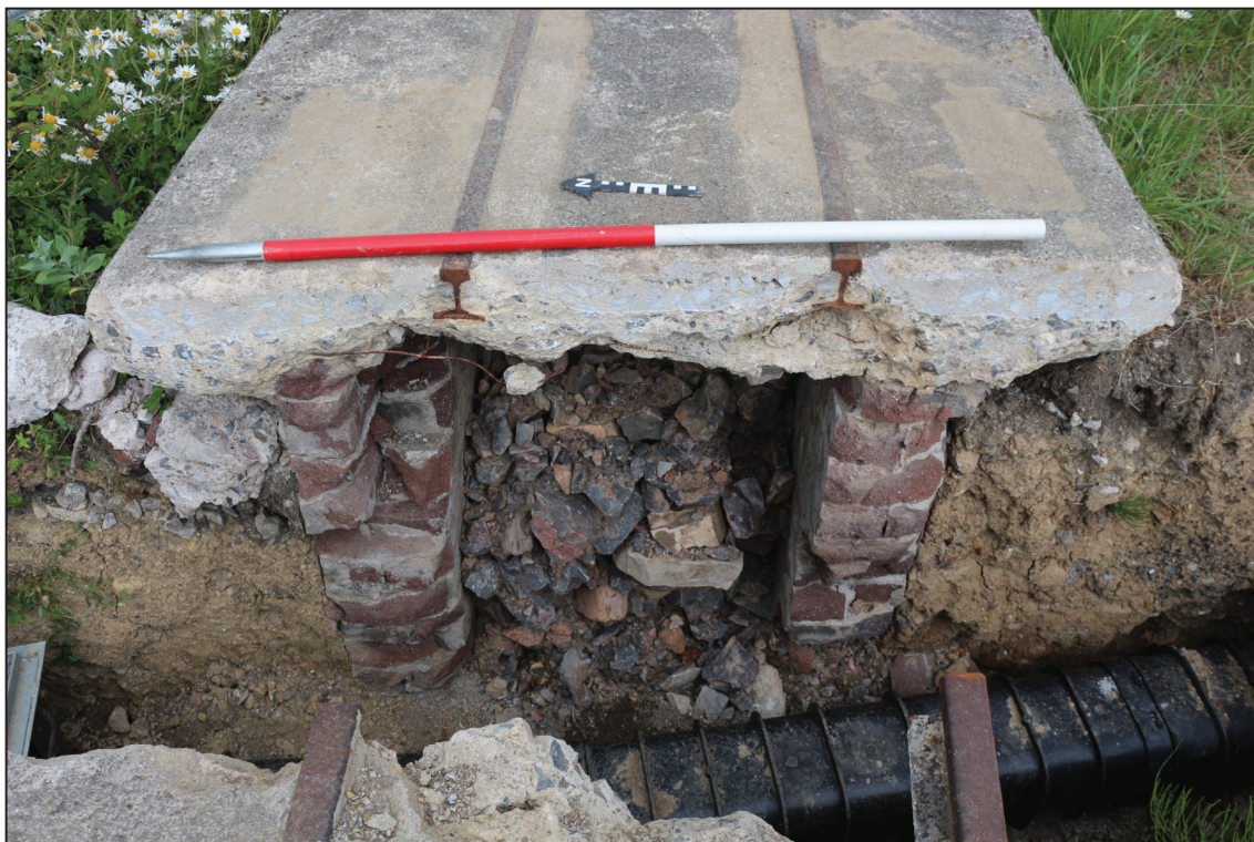
Tram piers 3002 and 3003, looking north-east (1m scale)
