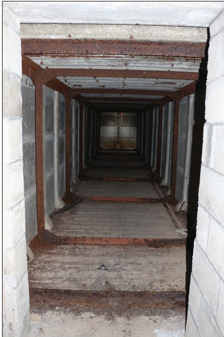
Main chamber of shelter 203, looking south-east (1m scale)
