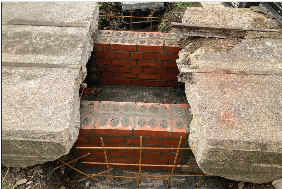
Reconstructed brick plinths at piers 3002 and 3003
