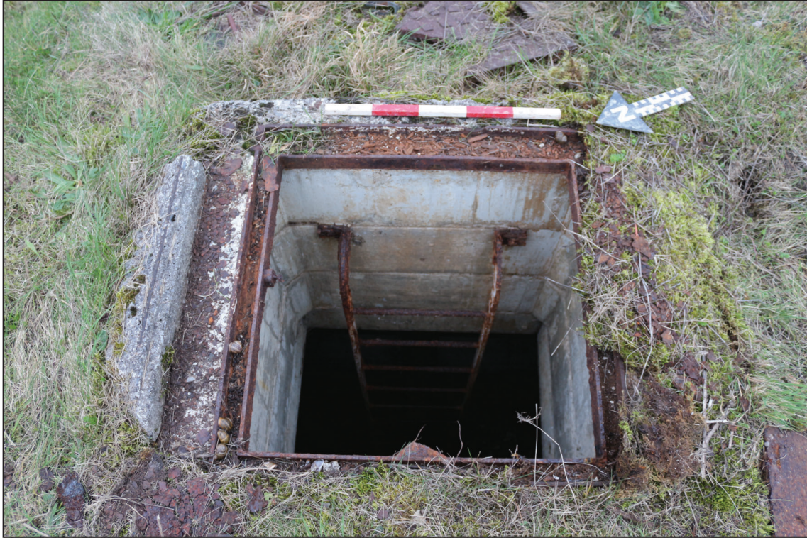
Exit hatch from shelter 203, looking south-east (0.5m scale)
