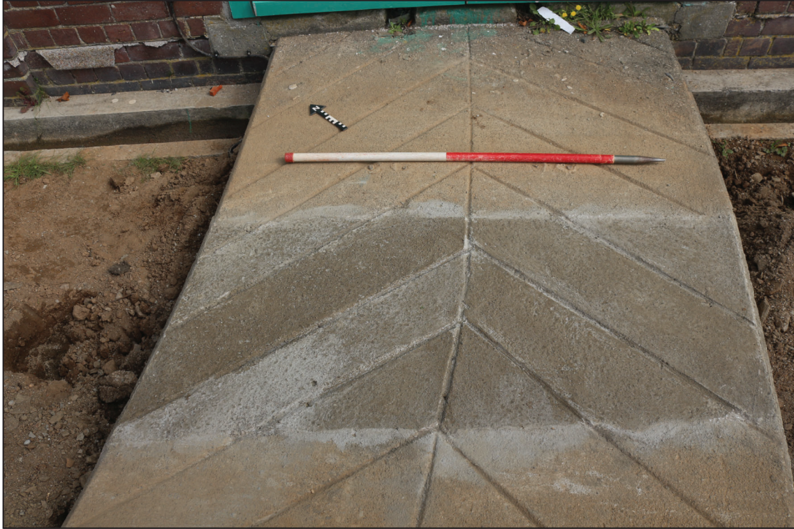
Reconstructed ramp at piers 3027 and 3028, looking north-east (1m scale)
