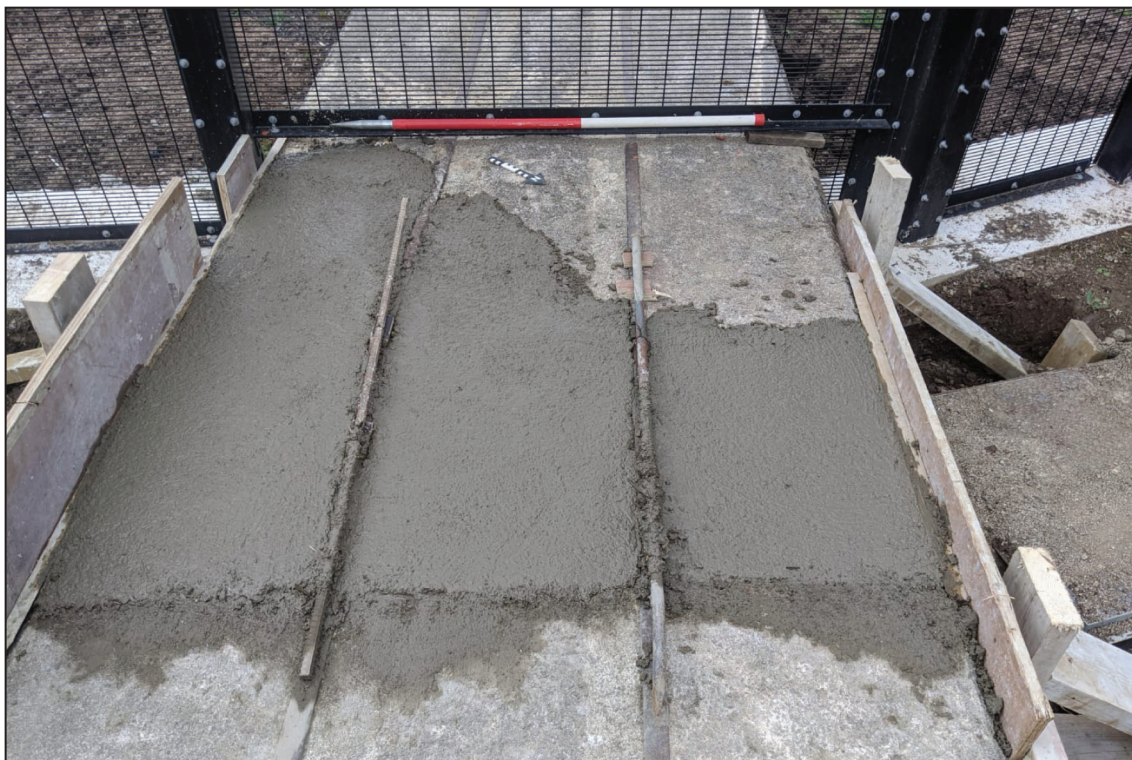
Concrete tramway and replacement metal rails (1m scale)
