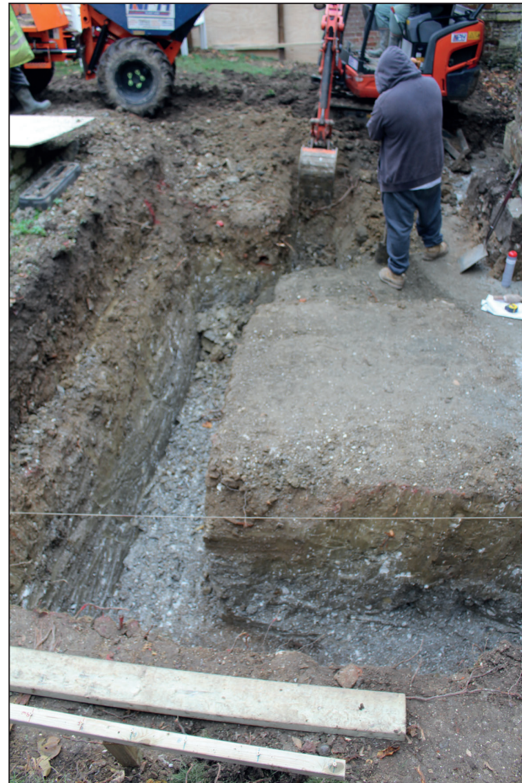
Foundation trench excavations, looking north-east (1m scale)
