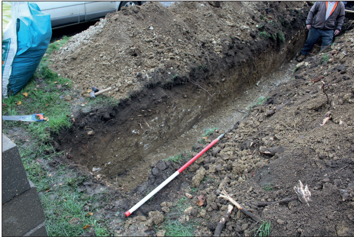
Pipe trench, looking north-east (1m scale)
