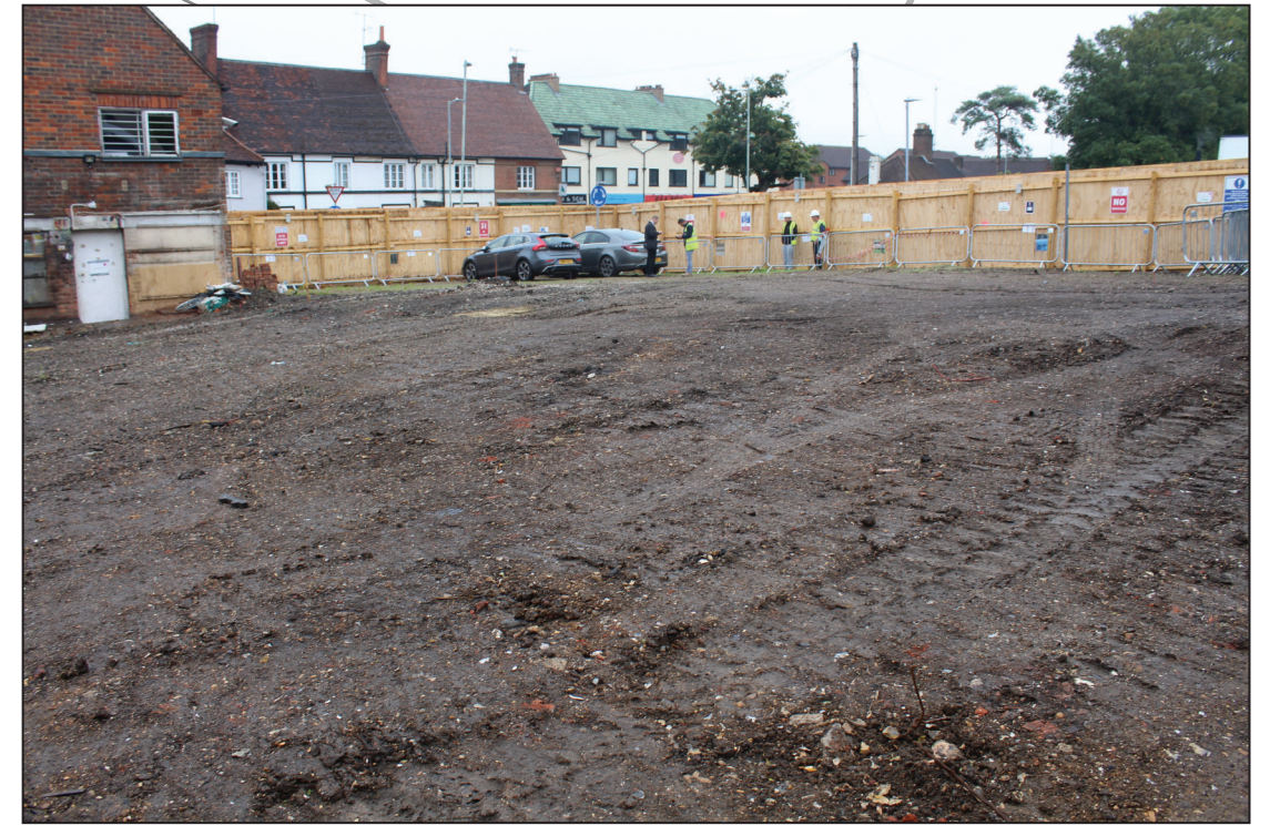
General view of the site, looking north-east
