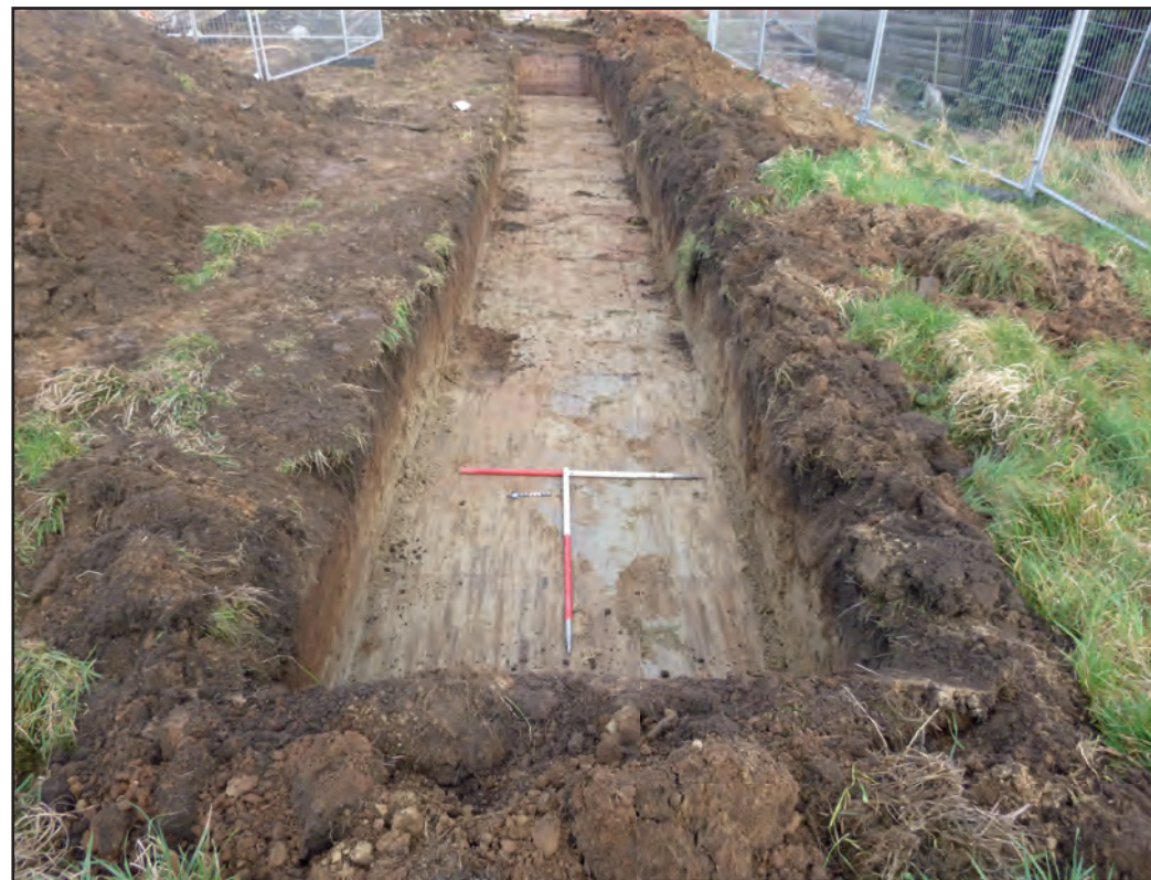
Trench 4, looking east (1m scales)
