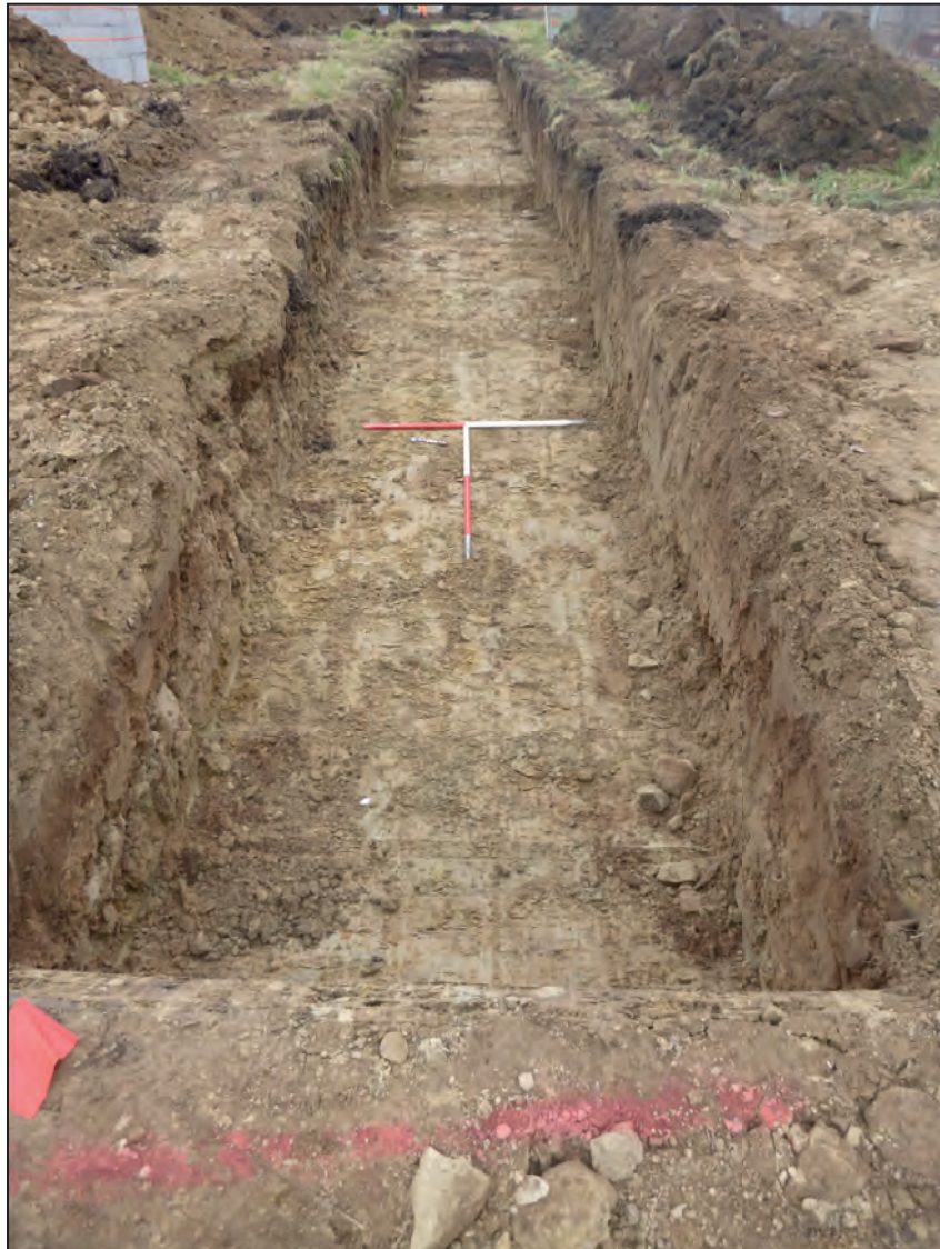
Trench 3, looking east (1m scales)
