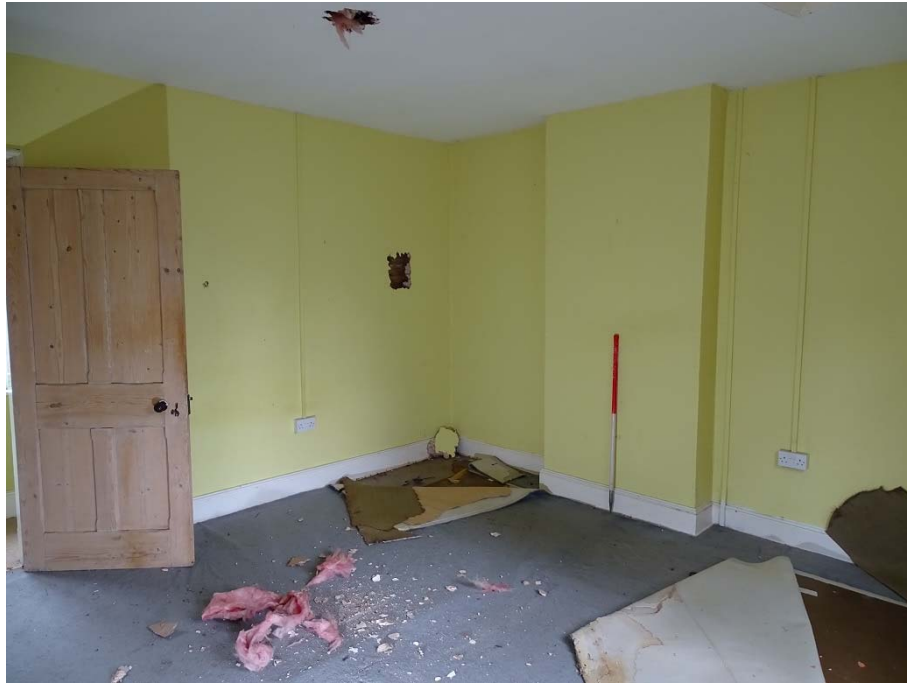
Photo 110: Cottages first floor room 10 looking north
