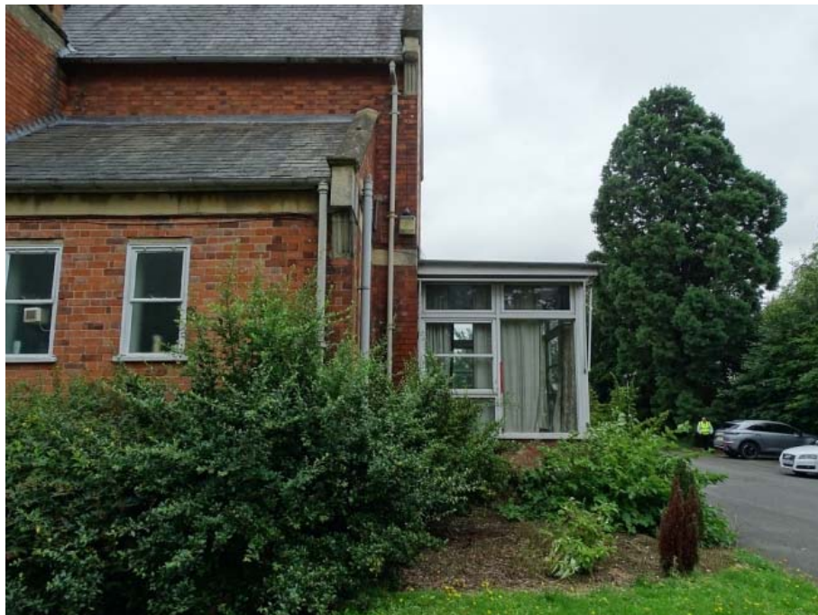
Photo 5: South elevation of the House looking east at the 20th century porch extension
