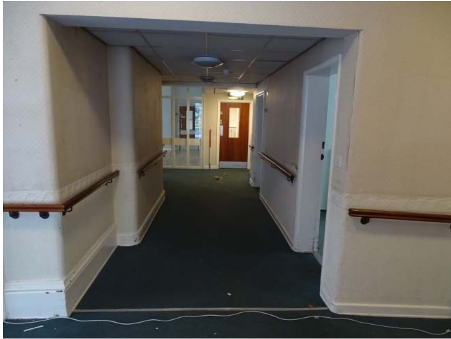
Photo 28: Ground floor north/south corridor looking north
