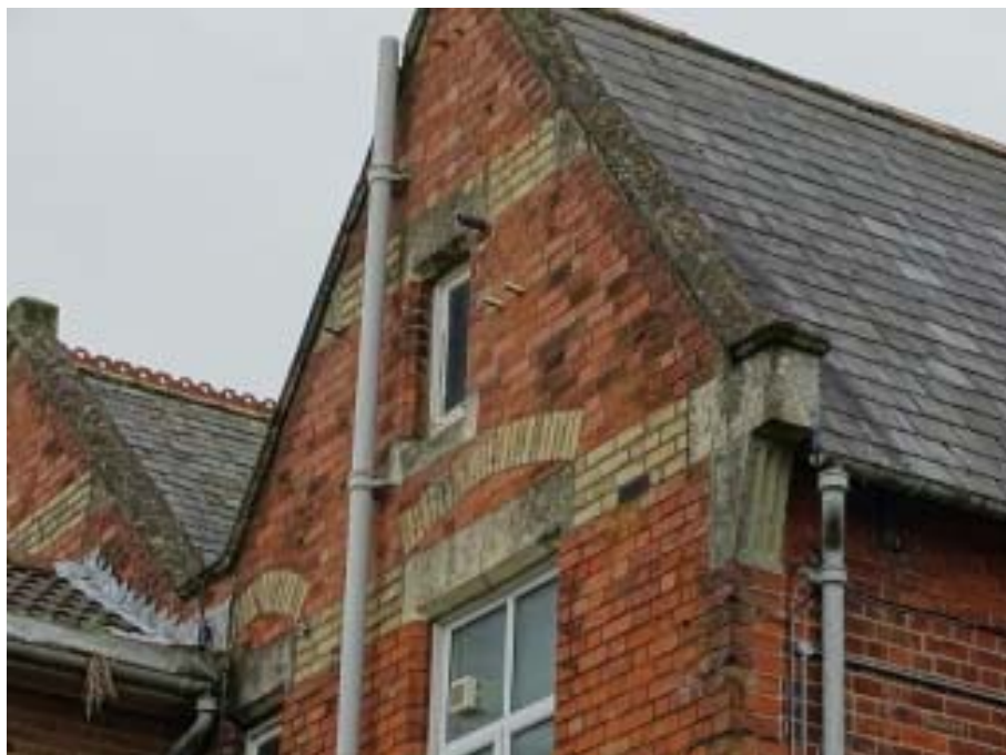
Photo 15: East elevation gable of the House at the south aspect detail
