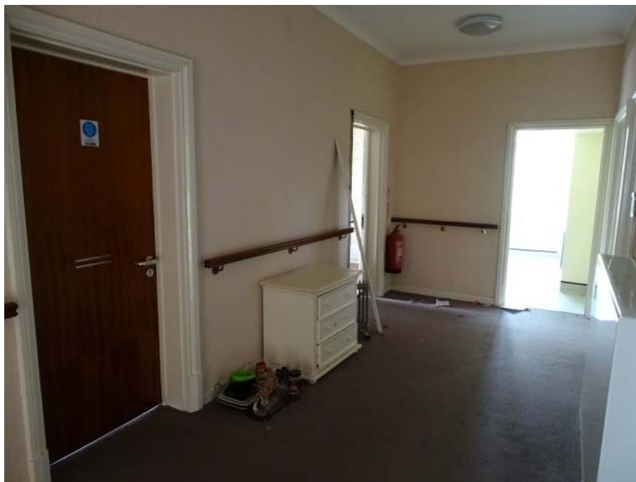
Photo 47: First floor east/west corridor of the House looking west
