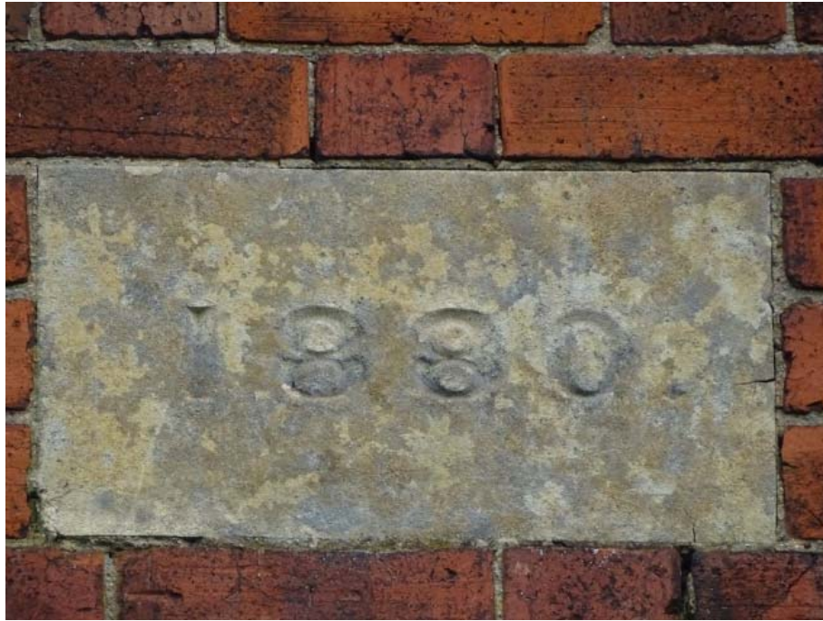
Photo 79: The Cottages date stone at south elevation
