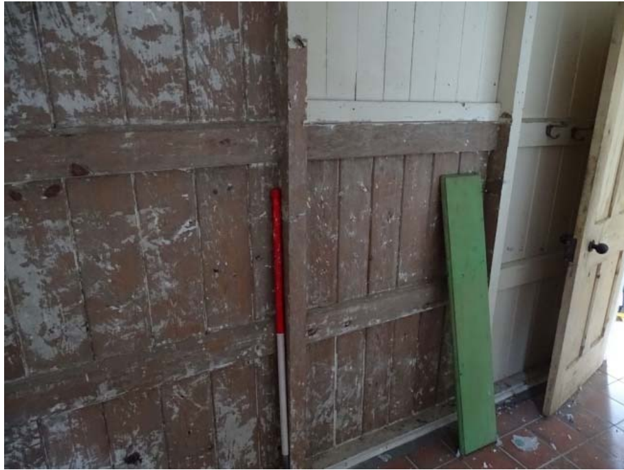
Photo 90: Cottages ground floor room 3 timber partition arrangement
