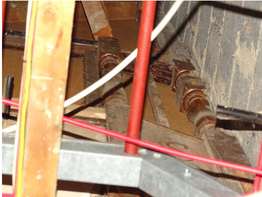
Photo 117: Staircase behind suspended ceiling in the ground floor of the House
