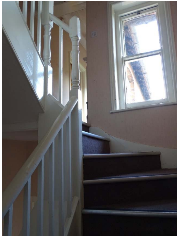
Photo 68: First to second floor staircase looking north
