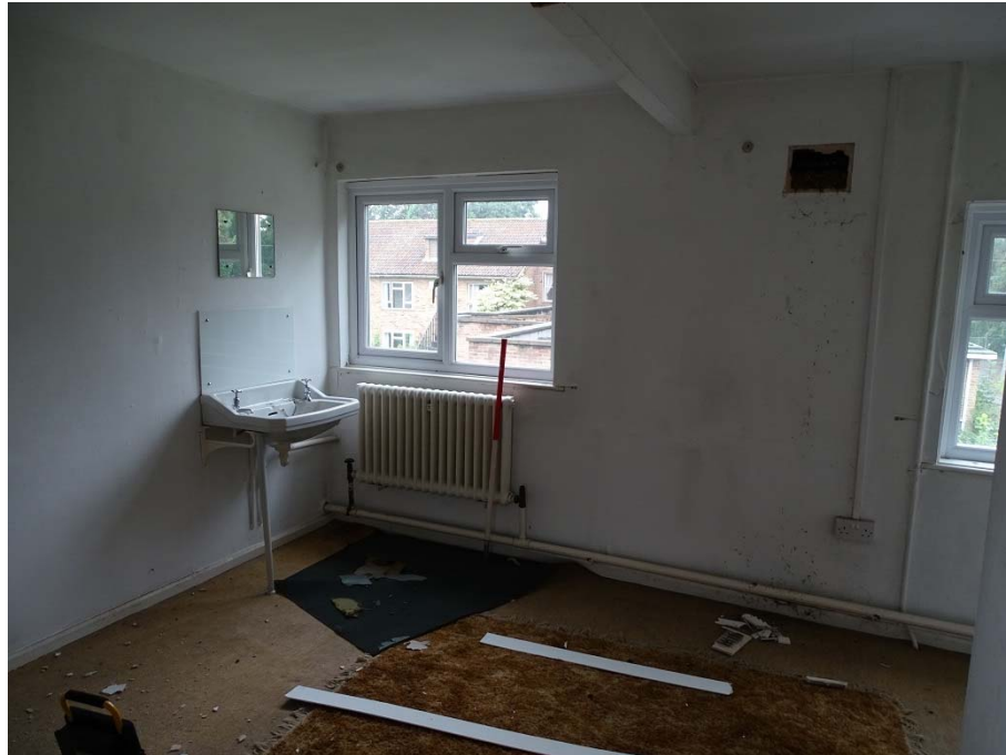
Photo 112: Cottages first floor room 12 looking south
