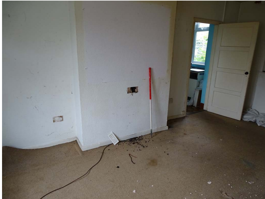
Photo 101: Cottages ground floor room 6 fireplace area
