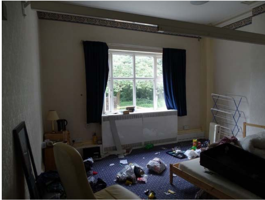
Photo 25: Room 4 at ground floor of the House looking west
