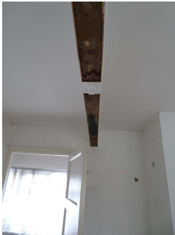
Photo 113: Cottages first floor room 12 full span timber beam
