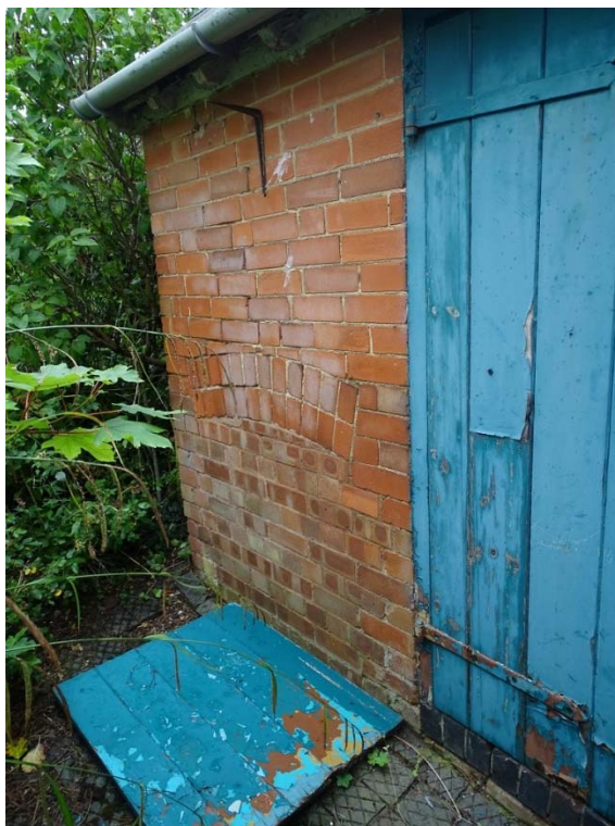
Photo 82: The Cottages outbuilding 2 at west elevation wall detail
