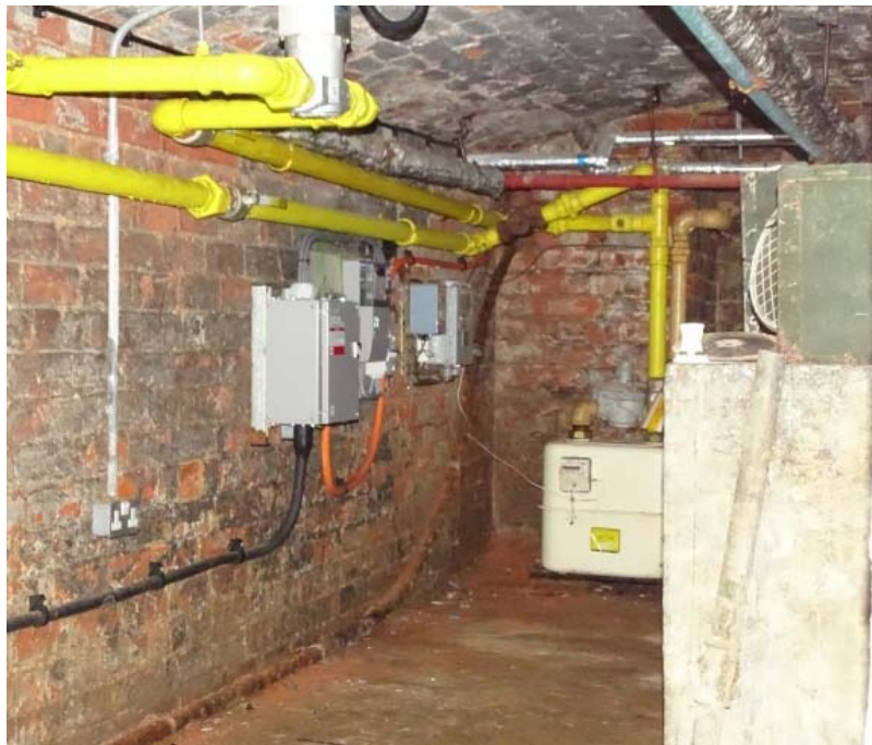
Photo 41: Basement/cellar of the House looking west at south aspect
