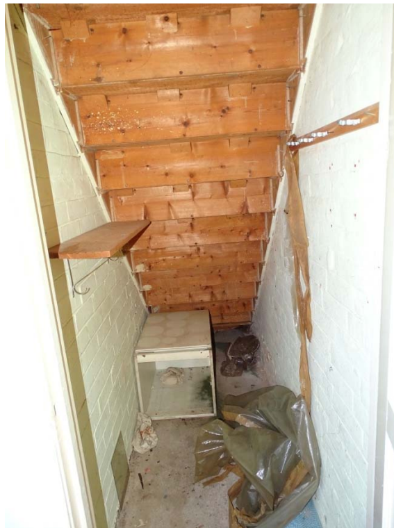
Photo 100: Cottages ground floor room 6 under stairs cupboard area
