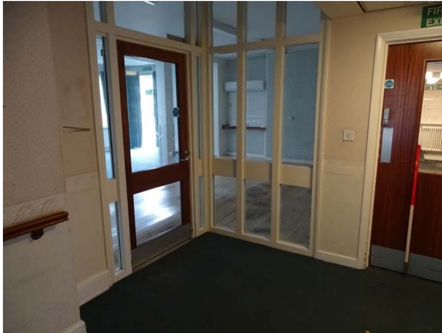
Photo 32: Entrance to ground floor room 7 of the House
