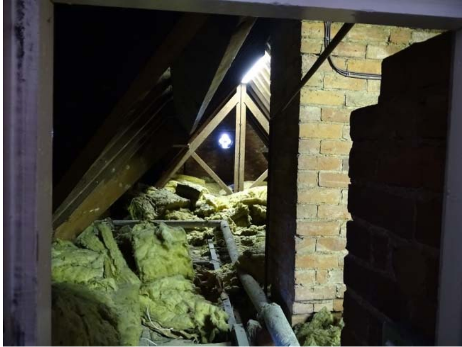
Photo 74: Second floor attic space 2
