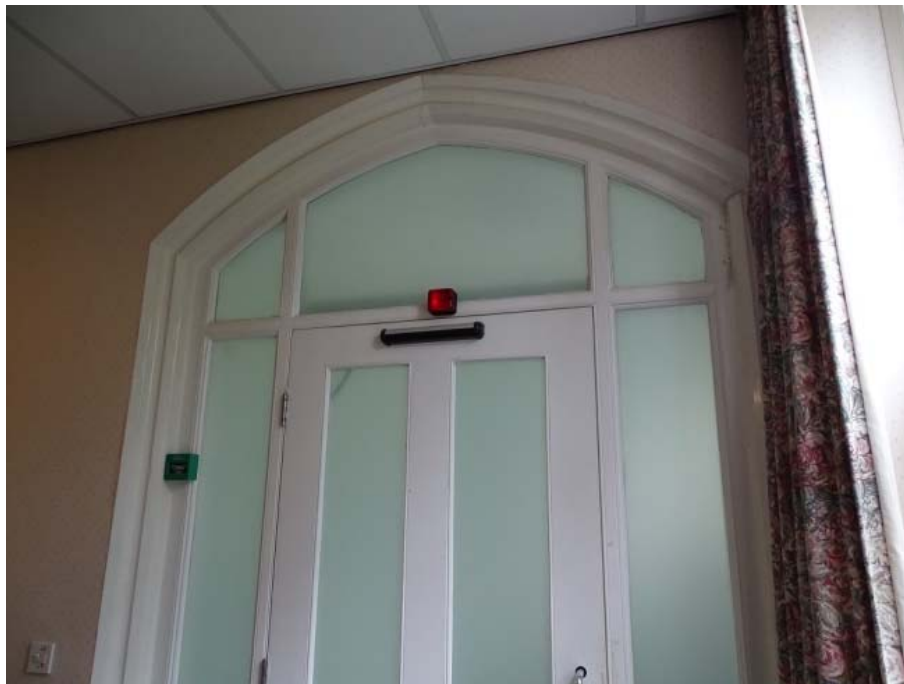
Photo 23: Ornate door at entrance to room 3 arch detail
