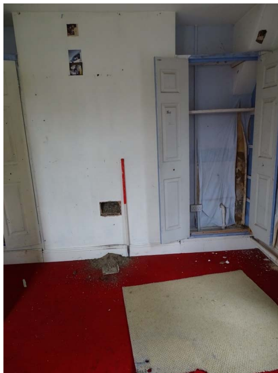
Photo 107: Cottages first floor room 9 fireplace area
