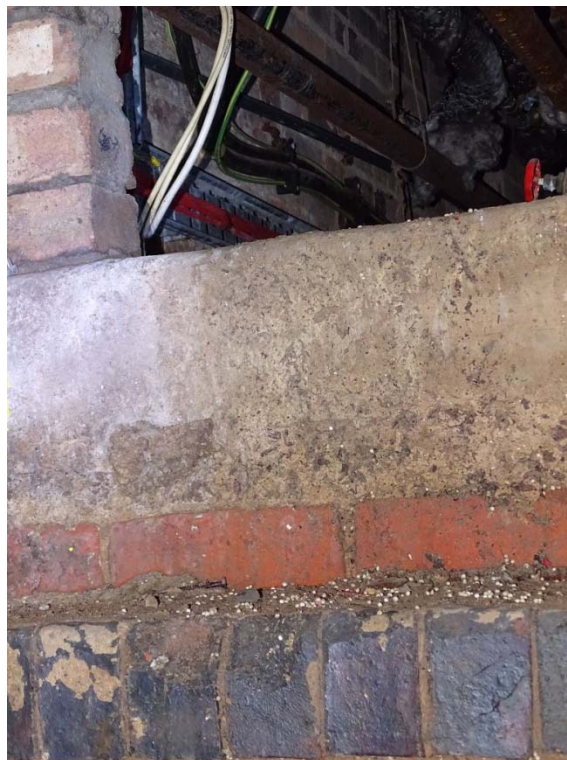
Photo 39: Basement/cellar of the House looking north
