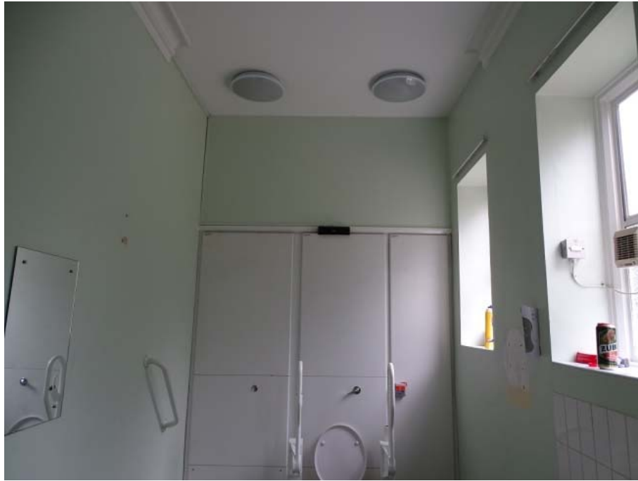
Photo 24: Room 3 at ground floor of the House
