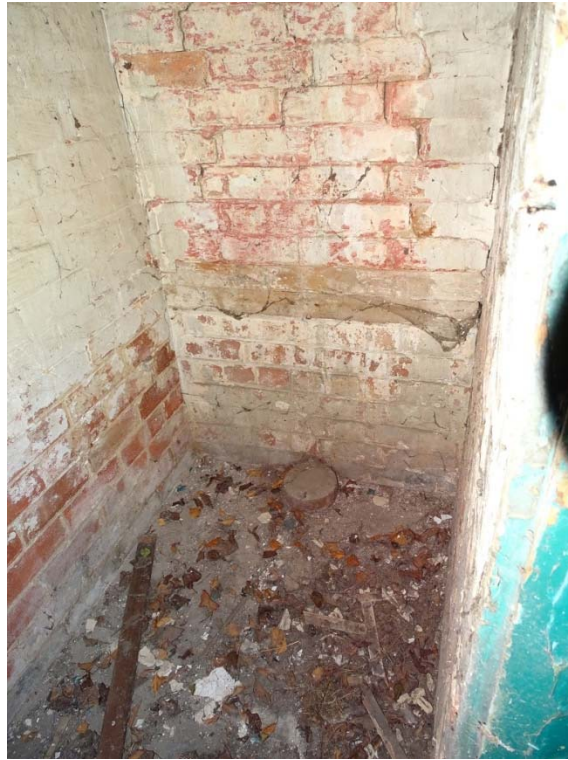
Photo 83: The Cottages outbuilding 2 interior detail
