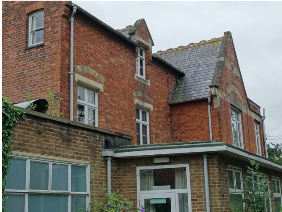
Photo 11: West elevation of the House at the north aspect looking south
