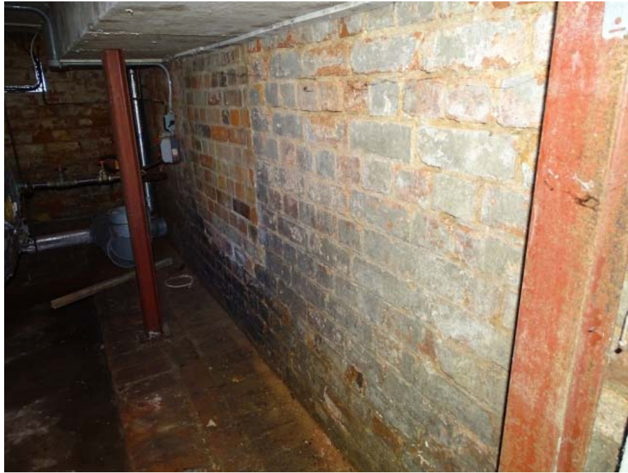
Photo 36: Entrance to the basement/cellar of the House
