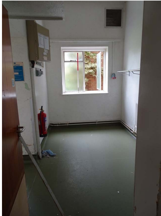
Photo 30: Room 6 at ground floor of the House
