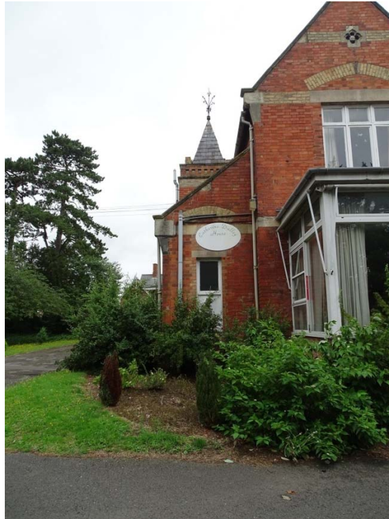
Photo 6: South elevation of the House west aspect looking north
