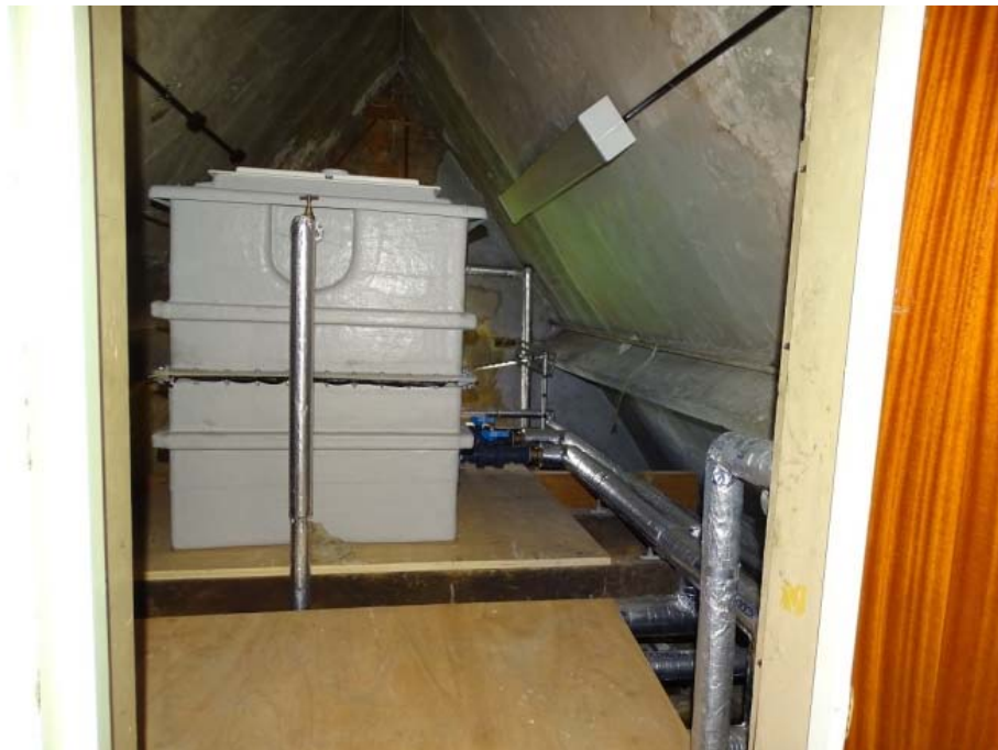
Photo 73: Second floor attic space 1
