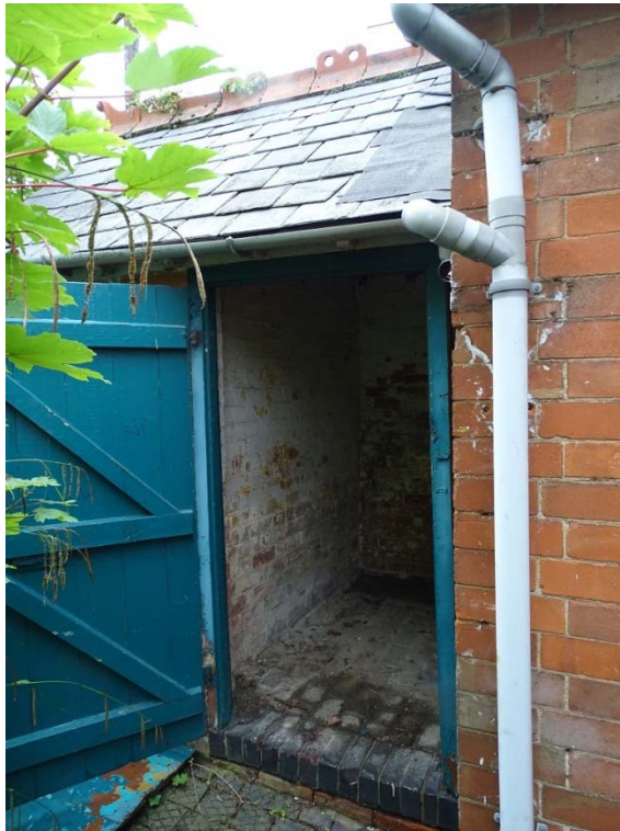
Photo 81: The Cottages outbuilding 1 at west elevation
