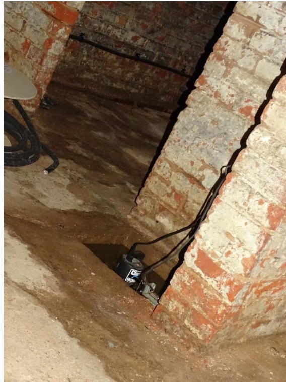
Photo 40: Basement/cellar of the House looking south
