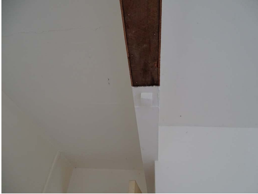
Photo 116: Cottages first floor room 14 full span timber beam
