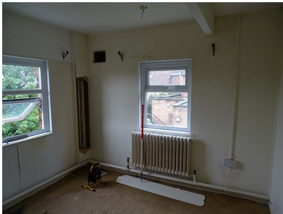
Photo 115: Cottages first floor room 14 looking south
