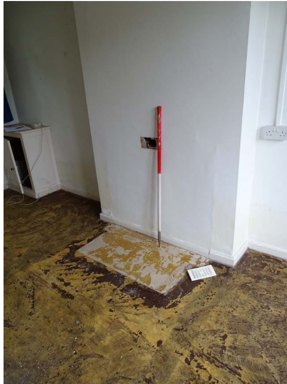
Photo 98: Cottages ground floor room 5 fireplace area
