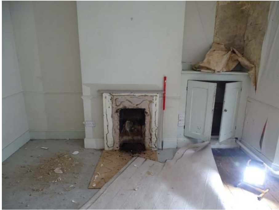
Photo 88: Cottages ground floor room 2 fireplace detail
