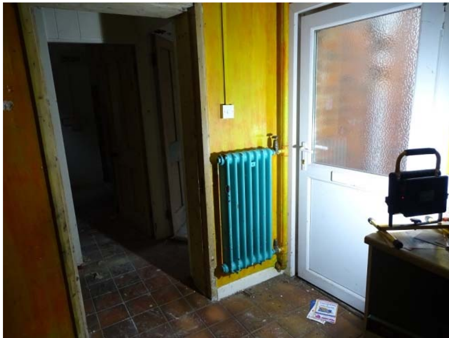
Photo 85: Room 1 of the Cottages looking east
