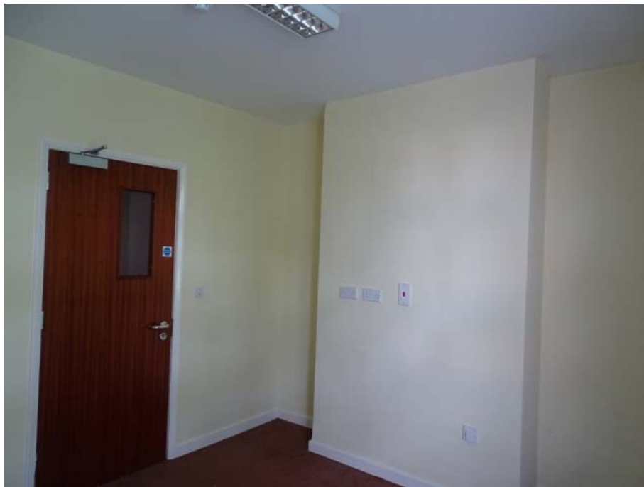
Photo 61: First floor room 14 of the House looking south east
