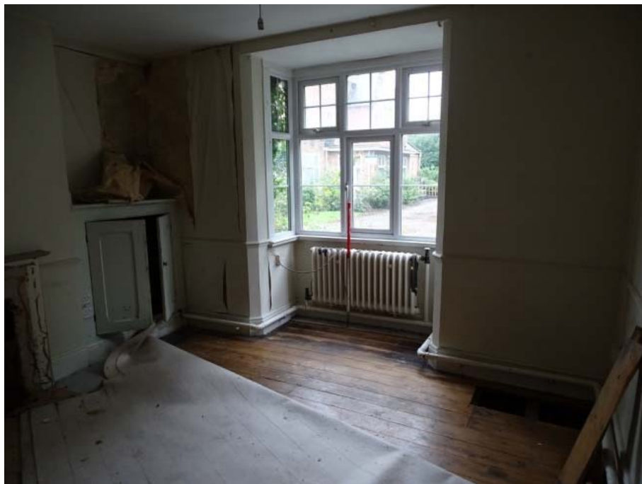
Photo 87: Cottages ground floor room 2 looking south
