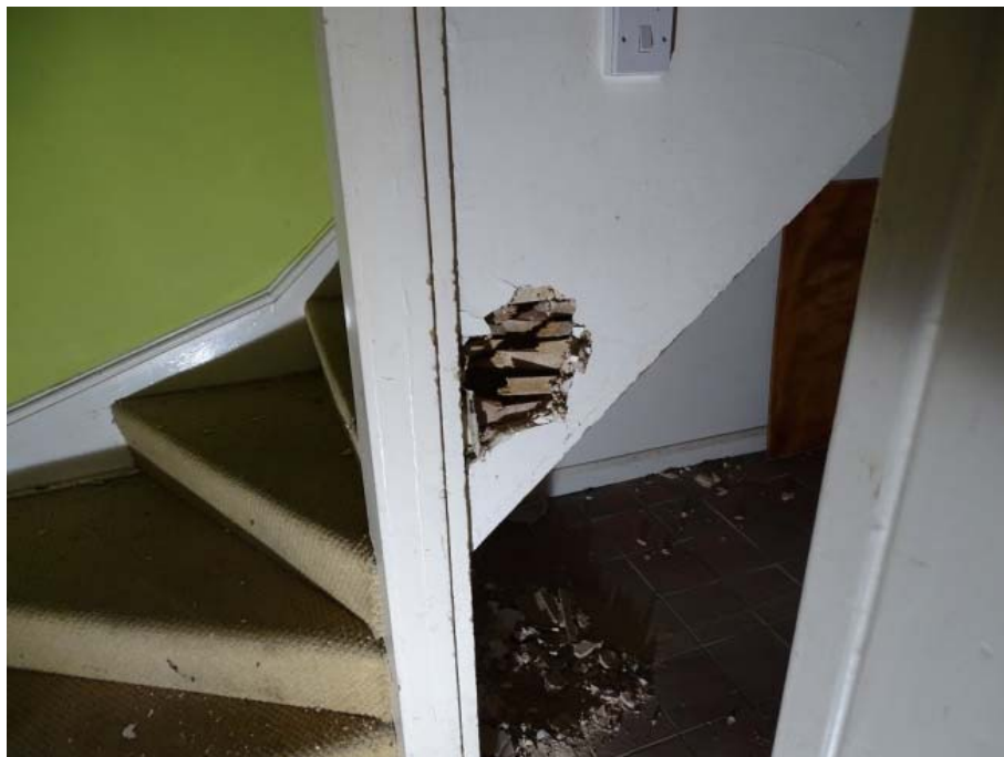
Photo 89: Cottages ground floor room 3 lath and plaster partition detail
