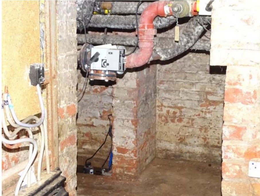
Photo 38: Basement/cellar of the House looking west at north aspect
