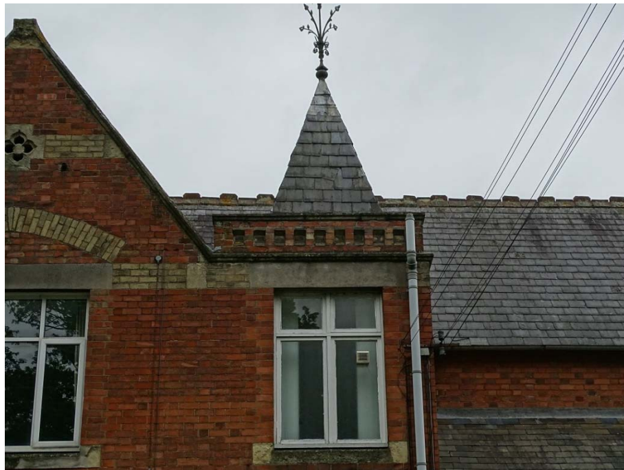
Photo 08: West elevation of the House parapet and turret detail
