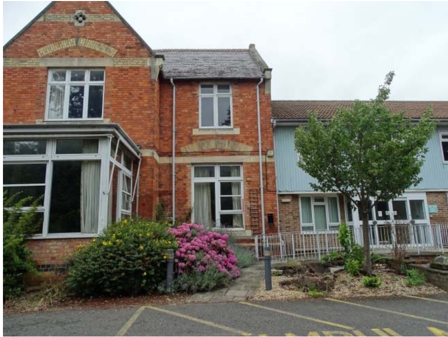
Photo 2: South elevation of the House east aspect
