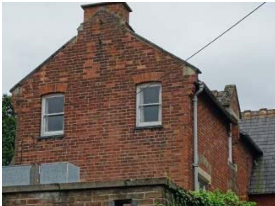
Photo 12: North elevation of the House
