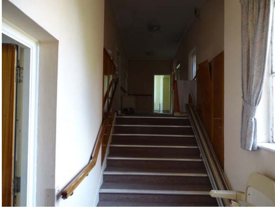
Photo 46: Entrance to the house at the first floor from the east aspect 20th century extension
