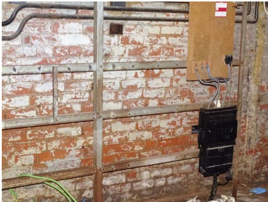
Photo 37: Basement/cellar of the House looking south
