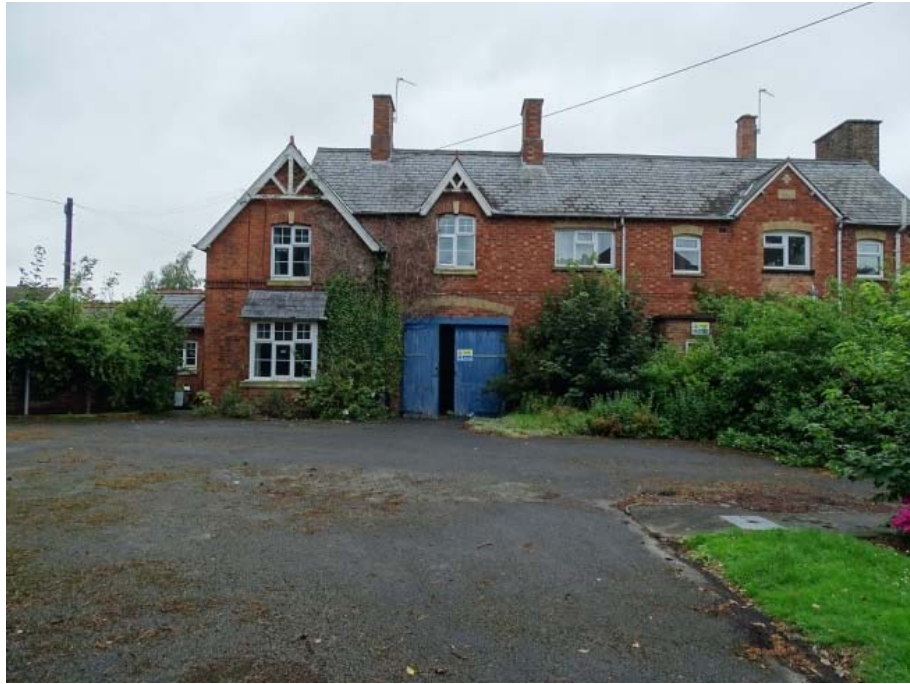
Photo 75: The Cottages south elevation
