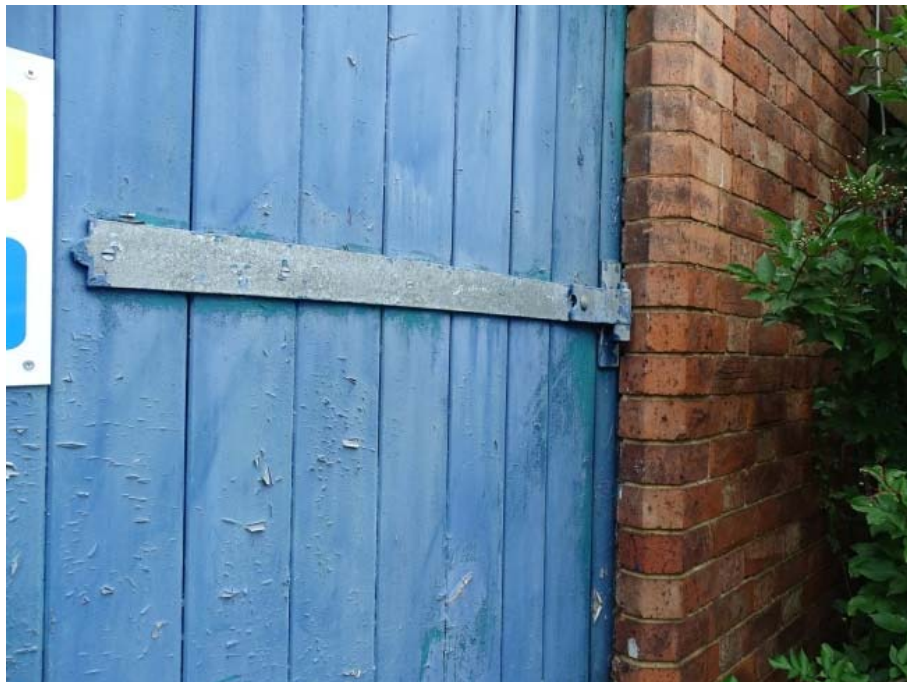
Photo 92: Cottages ground floor room 4 door detail east aspect
