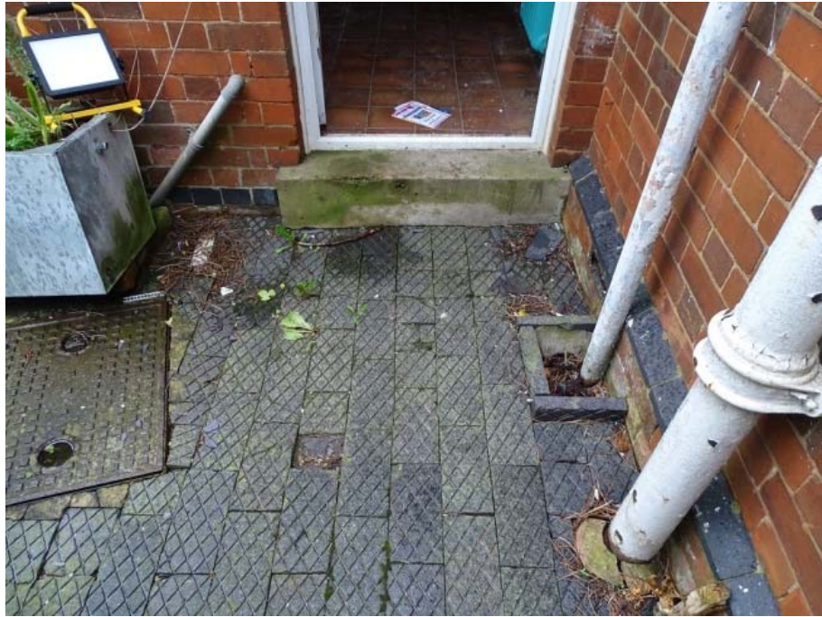
Photo 84: Entrance to Cottages at the west elevation
