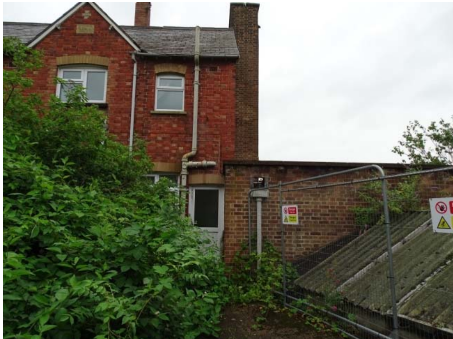
Photo 78: The Cottages south elevation intersection with 20th century extension
