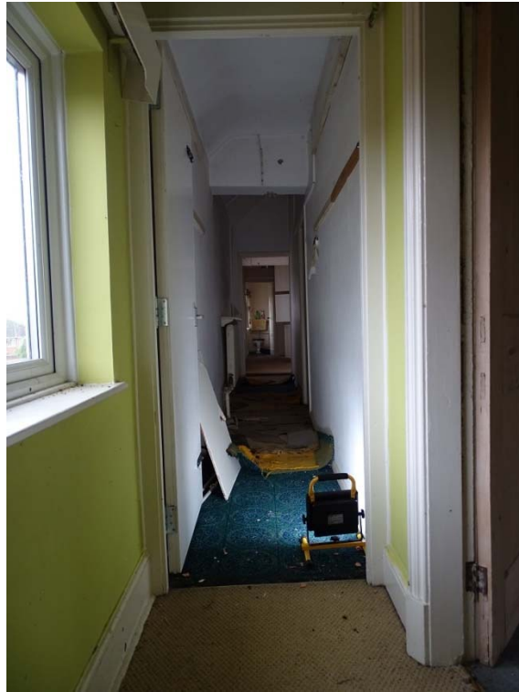
Photo 104: Cottages first floor east/west corridor looking east
