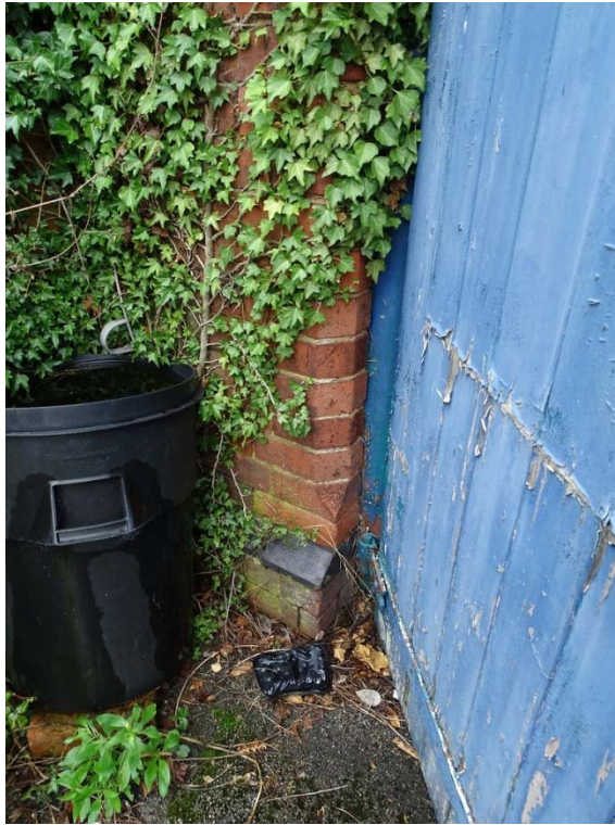
Photo 93: Cottages ground floor room 4 door detail west aspect
