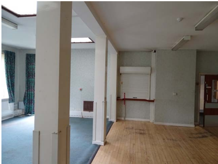
Photo 34: Looking north in ground floor room 7 of the House
