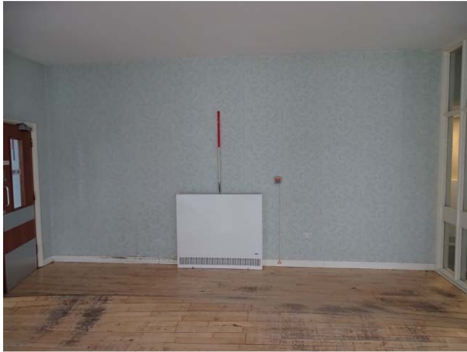
Photo 35: Looking east in ground floor room 7 of the House
