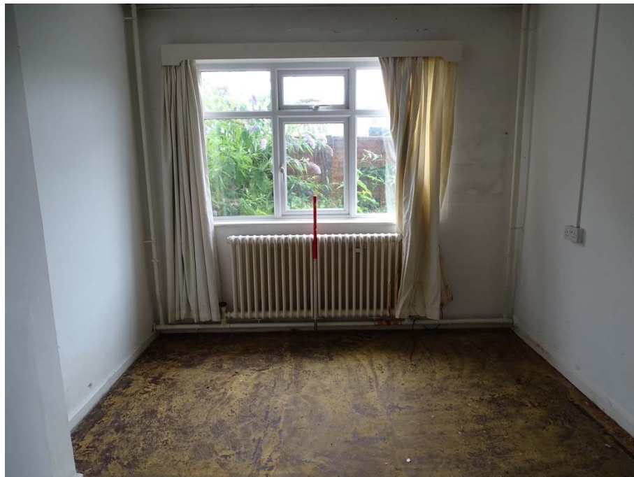
Photo 97: Cottages ground floor room 5 looking south
