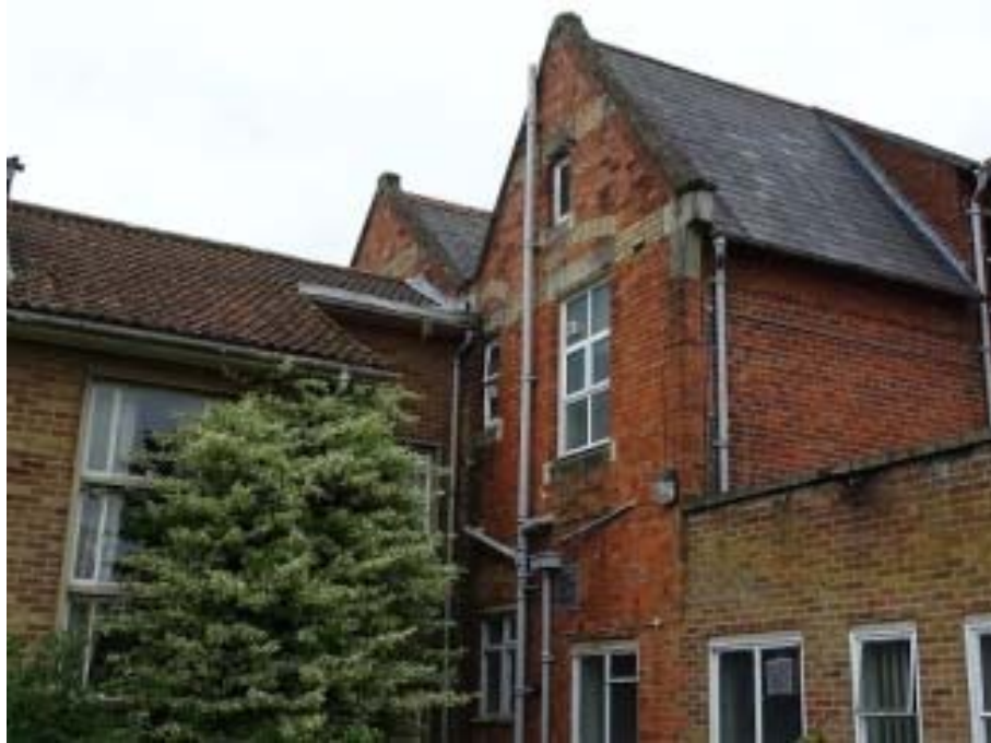
Photo 14: East elevation of the House at the south aspect
