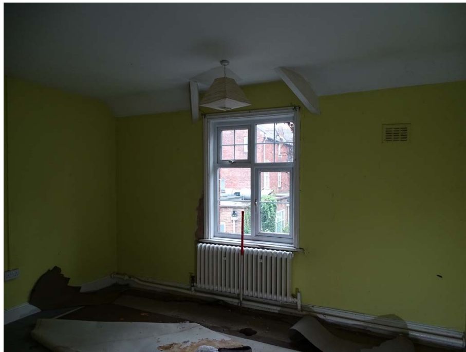
Photo 108: Cottages first floor room 10 looking south
