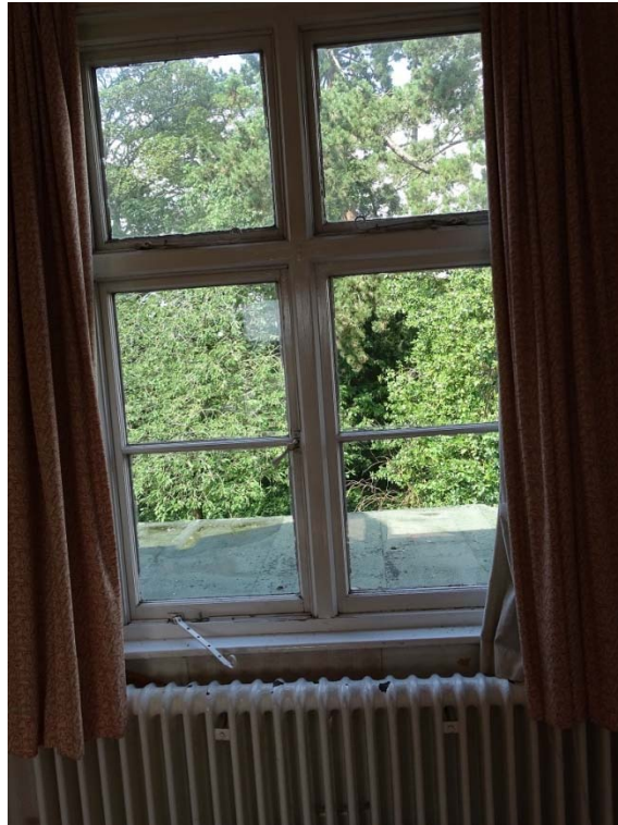
Photo 64: First floor room 15 of the house looking east
