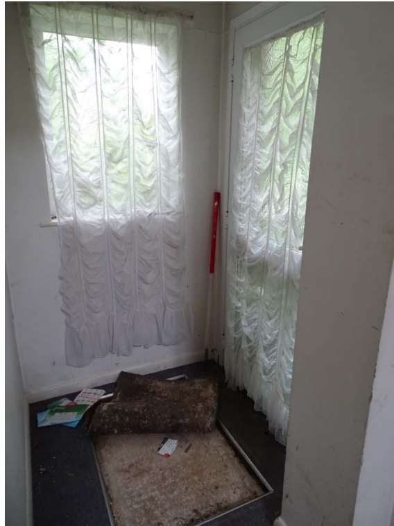
Photo 96: Cottages ground floor porch arrangement
