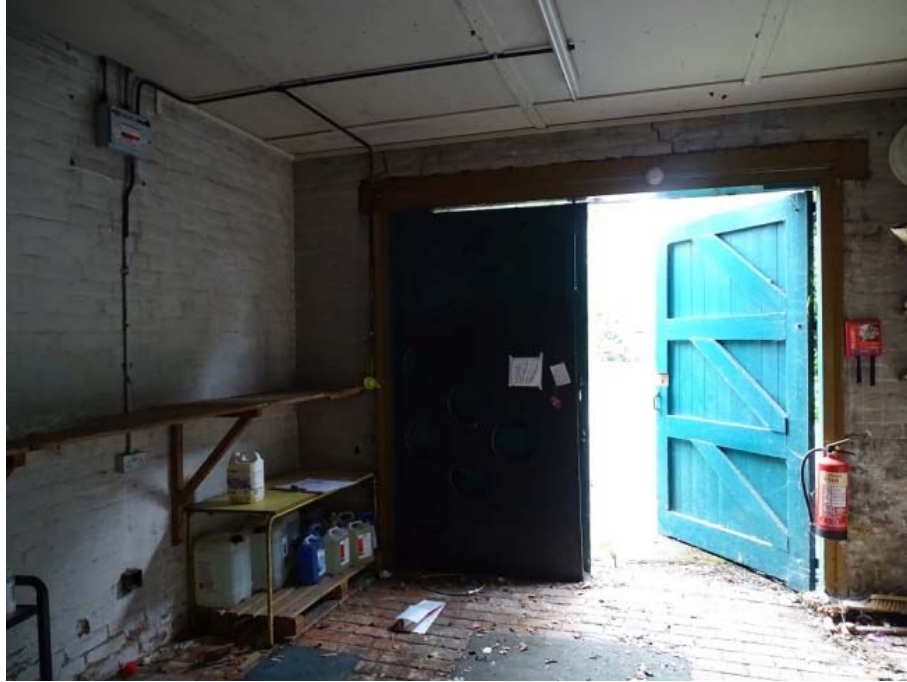
Photo 95: Cottages ground floor room 4 looking south
