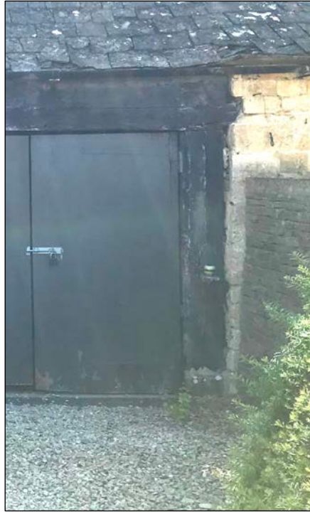
Fig. 40 View of junction between garage door and wall, south garage
