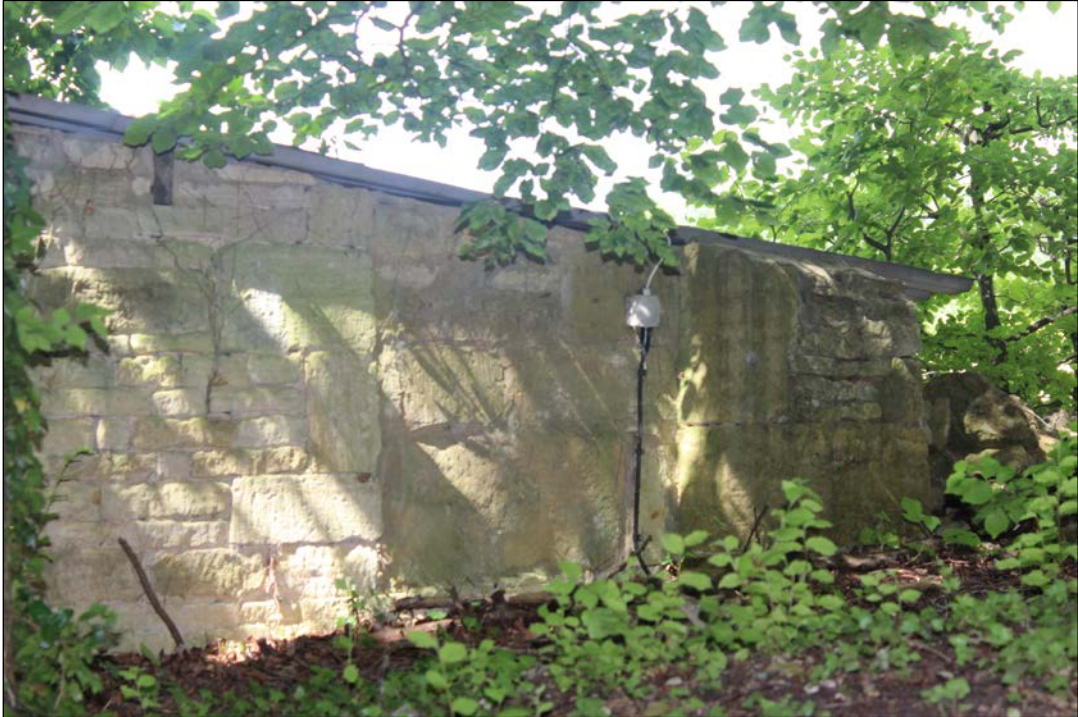
Fig.14 Filled-in doorway on north elevation
