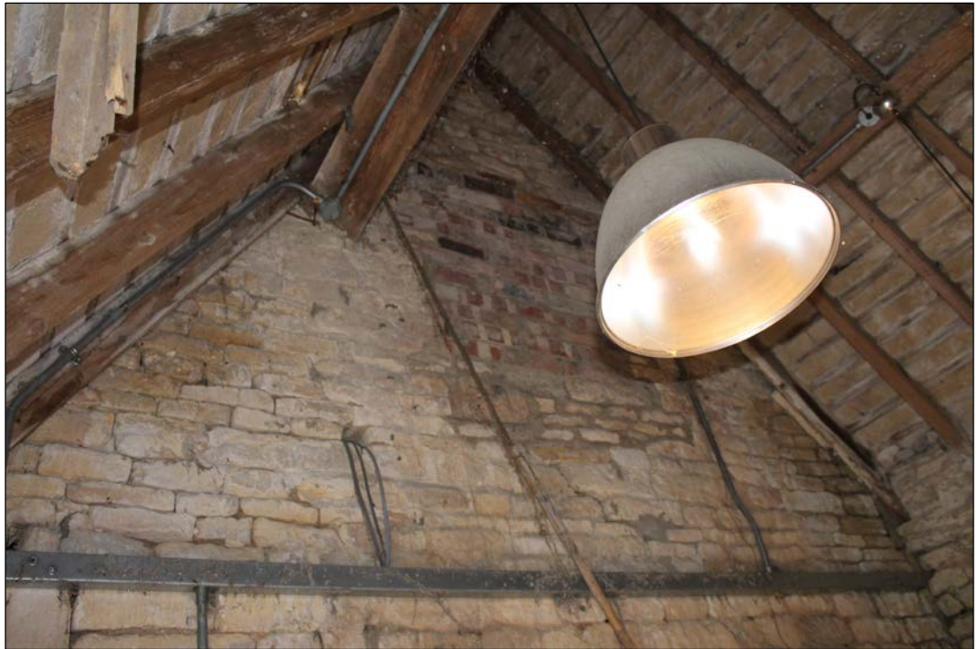
Fig. 33 Brick infill to the north gable wall of the south garage
