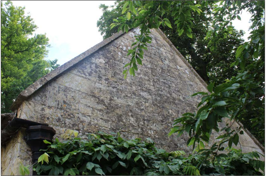
Fig. 22 South gable wall of south garage
