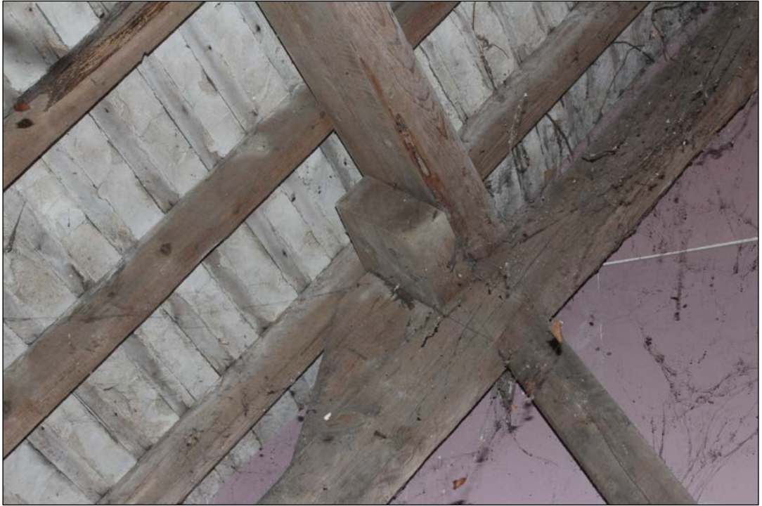
Fig. 30 Stacked back purlins with a cleat in the northern roof section
