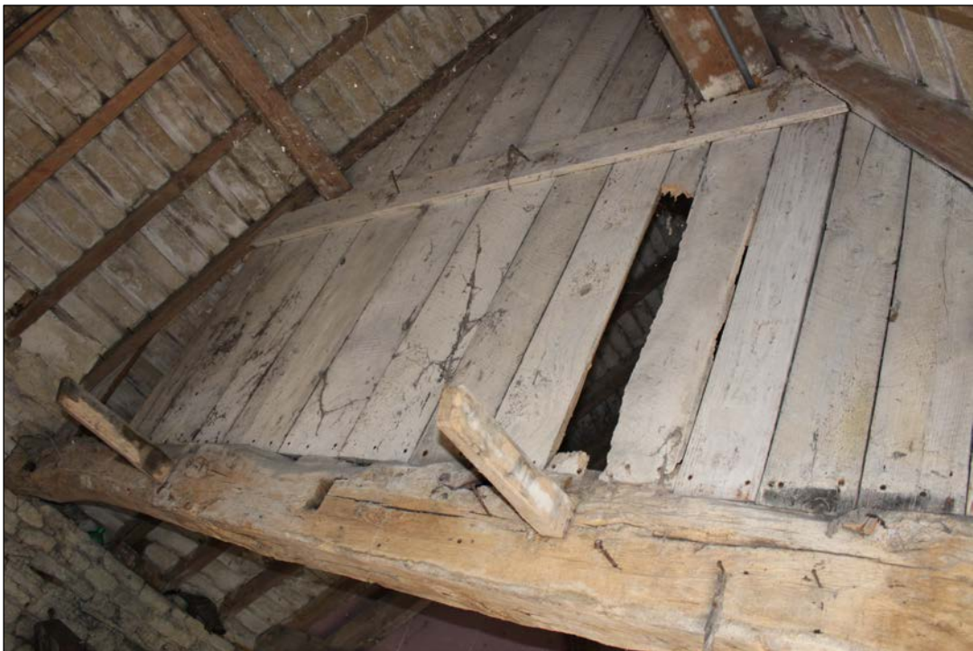
Fig. 29 Old oak tie beam in northern section, with timber board screen above
