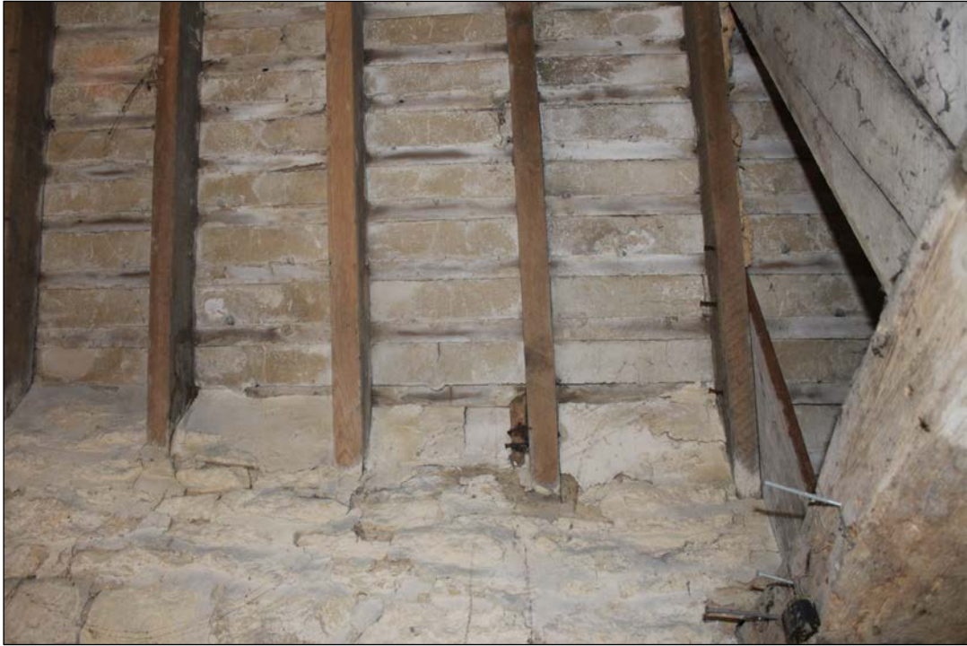
Fig. 32 Torching between rafters in northern section
