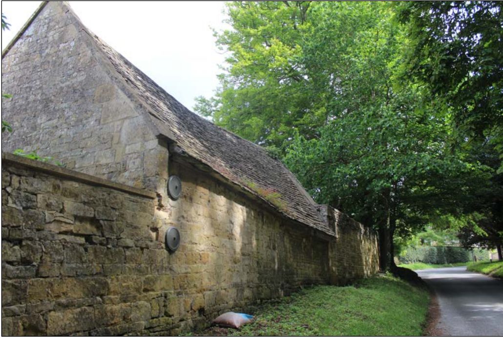
Fig. 36 East elevation of south garage, view to the north, showing metal ties
