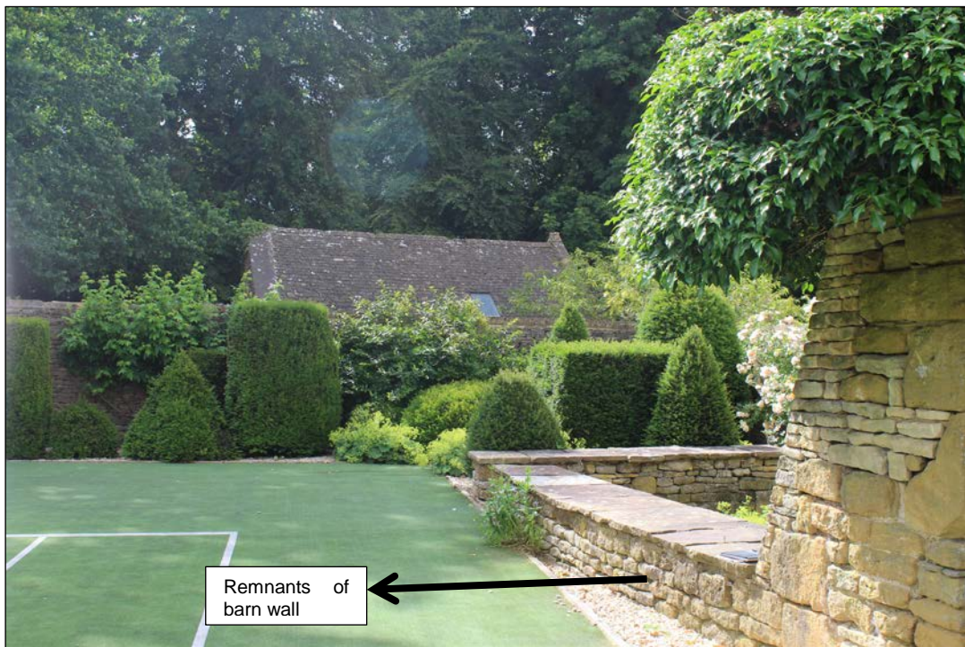
Fig. 8 View of remains of barn wall, view looking east towards the garages
