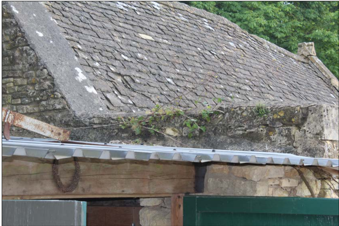
Fig.17 West gable capped in mortar
