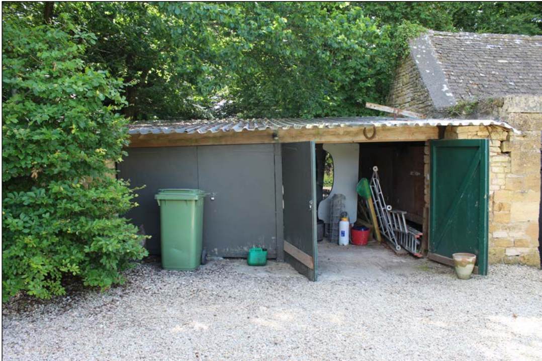
Fig. 11 View east to the northern garage
