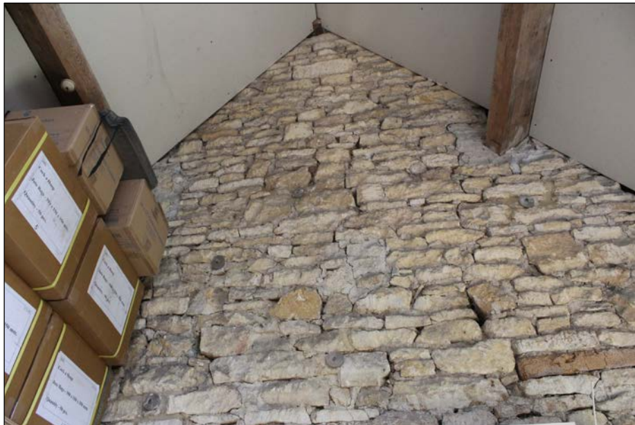
Fig. 23 Internal south gable wall of south garage
