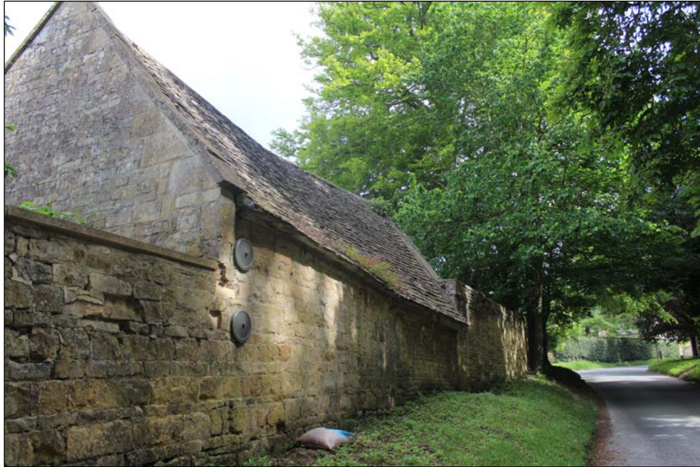
Fig. 9 East, roadside elevation of the garages, view to the north
