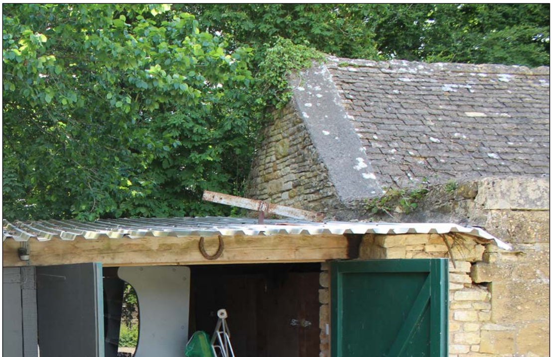
Fig. 34 External face of north gable wall to south garage
