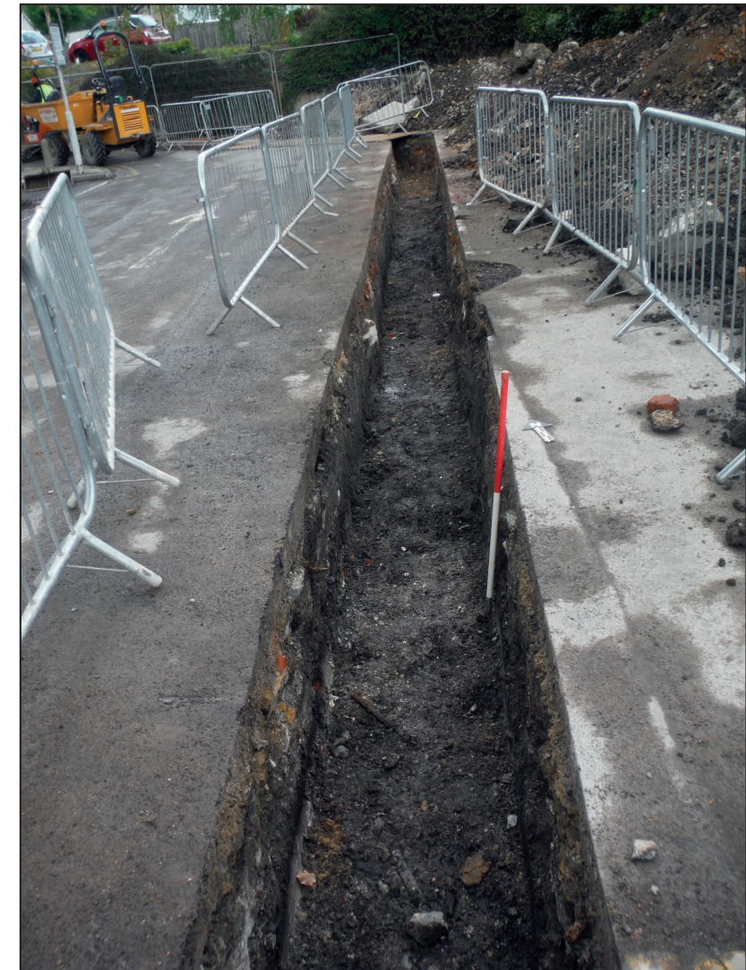
Trench 3, monitored groundworks, looking north (1m scale)
