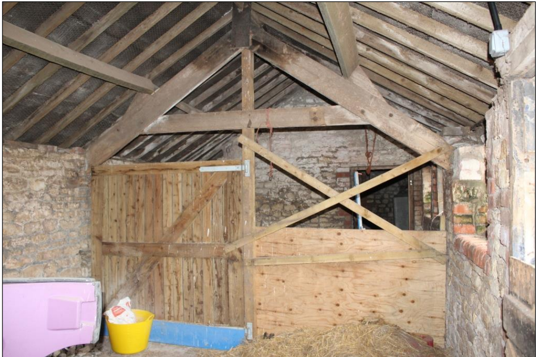
Photograph 9 Timber dividing wall between rooms 2 and 3
