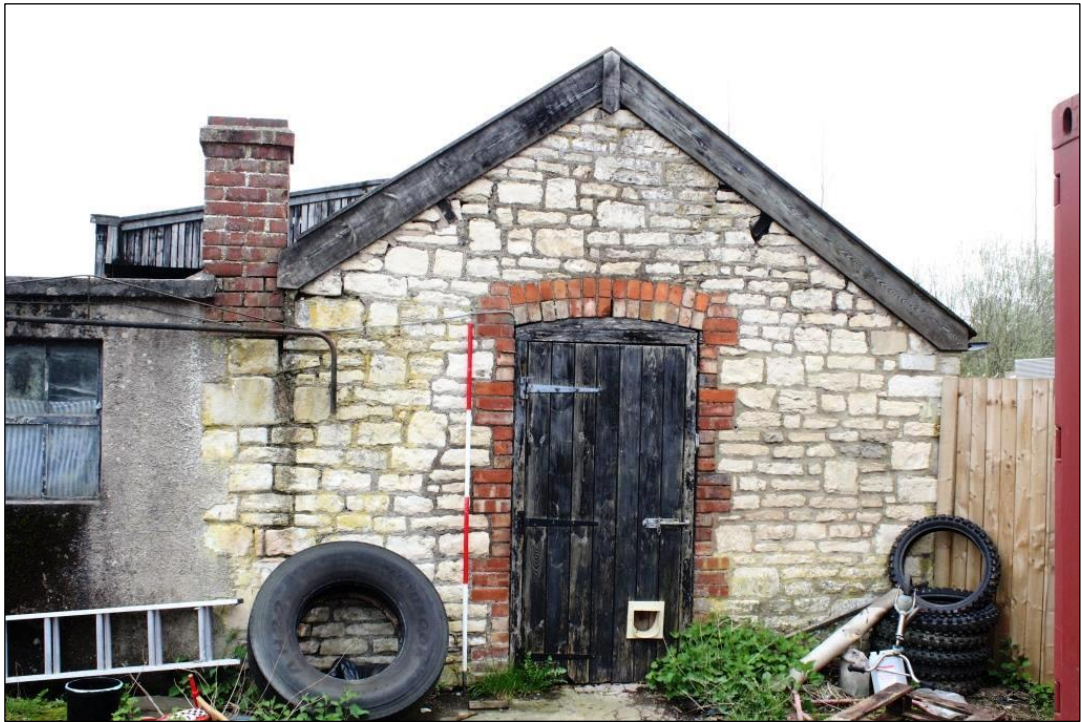
Photograph 1 Western range of north facing elevation of the bull pen
