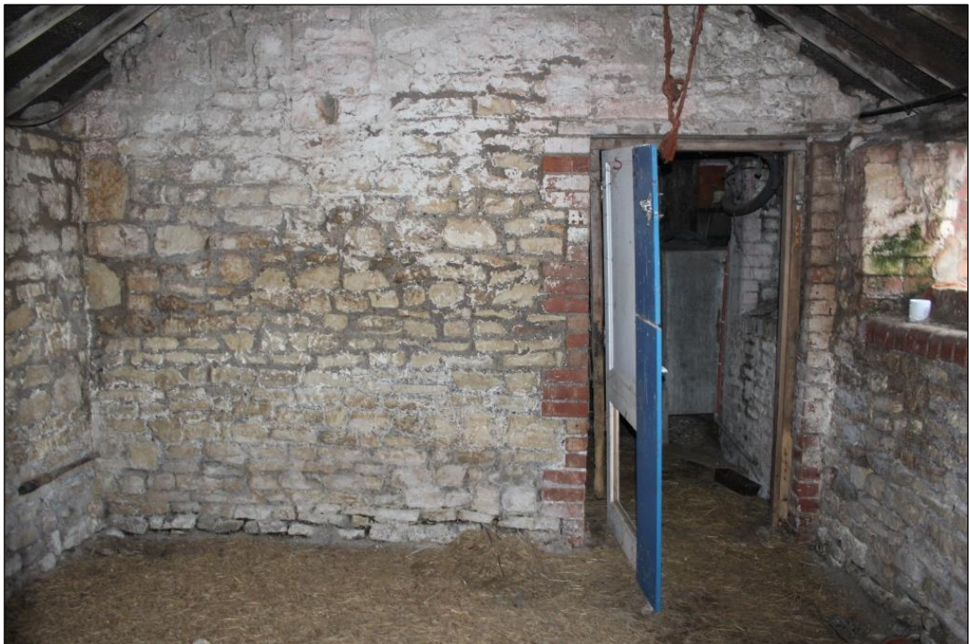
Photograph 8 Stone dividing wall between rooms 1 and 2
