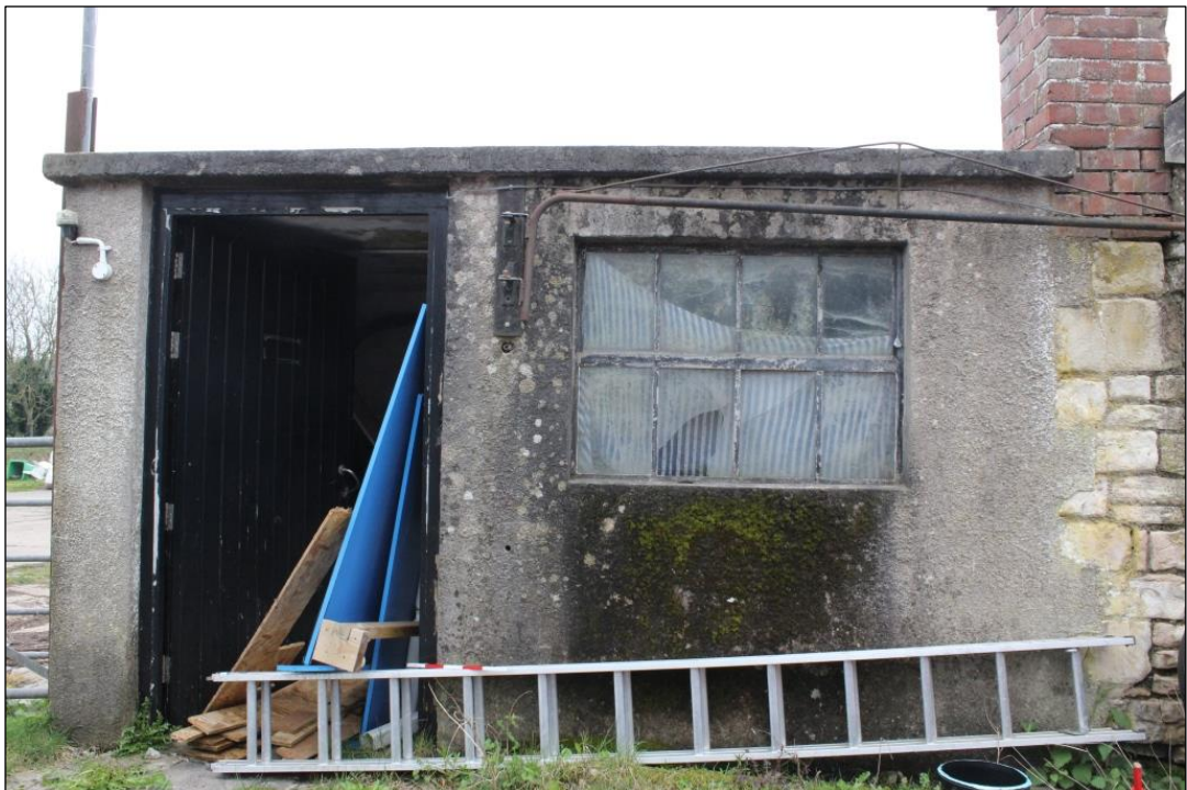
Photograph 2 Eastern range of north facing elevation of the bull pen
