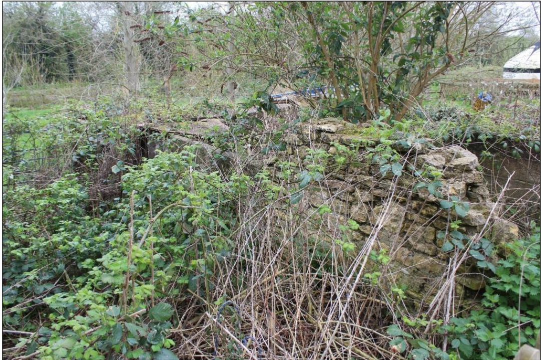
Photograph 14 General view of pig sty
