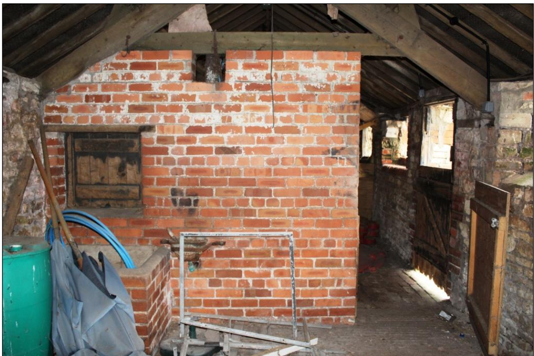
Photograph 10 Brick dividing wall between rooms 3 and 4 with hatch
