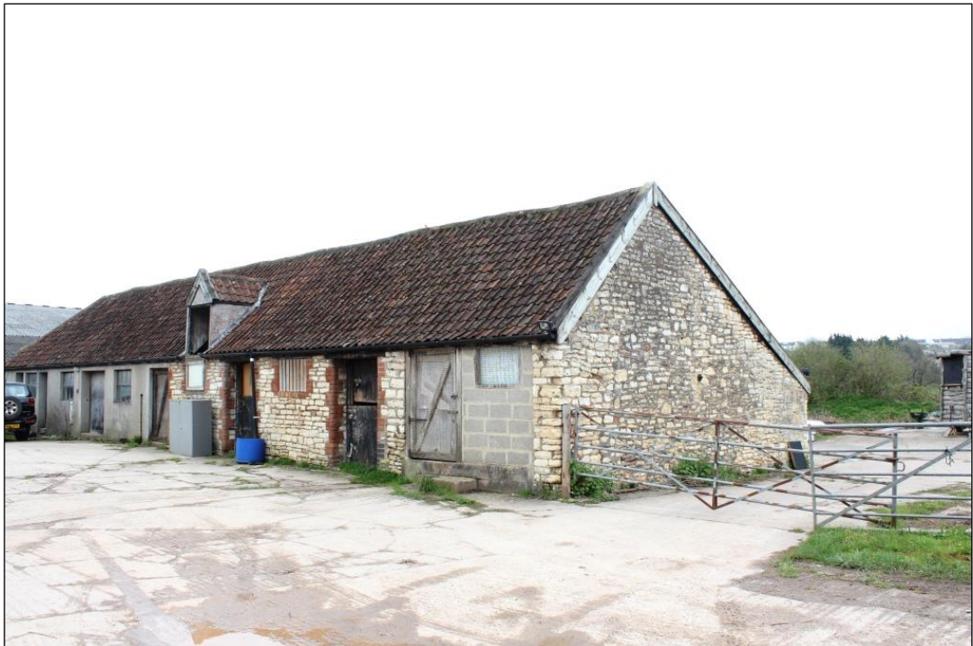
Photograph 11 North facing elevation of the stable and dairy block
