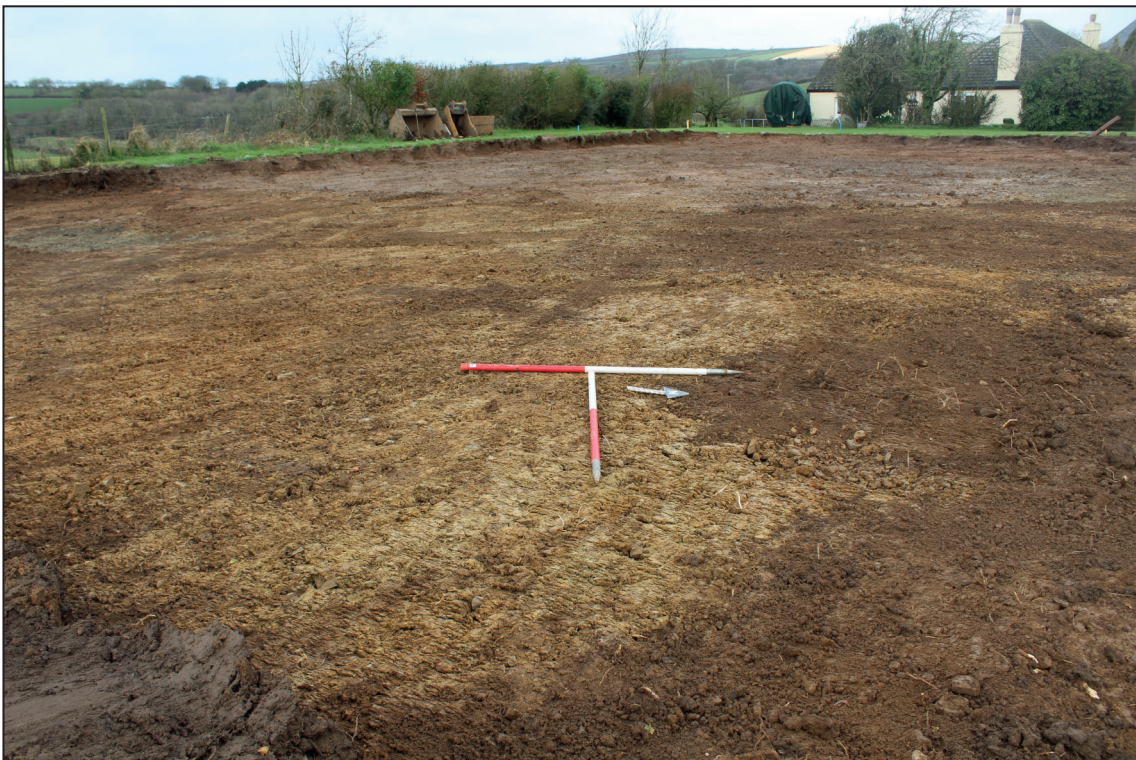
Monitored groundworks, post-excavation, looking west (1m scales)
