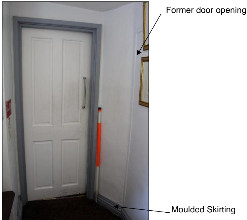
Photo 65: Detail of four panelled door between the landing and eastern corridor.
