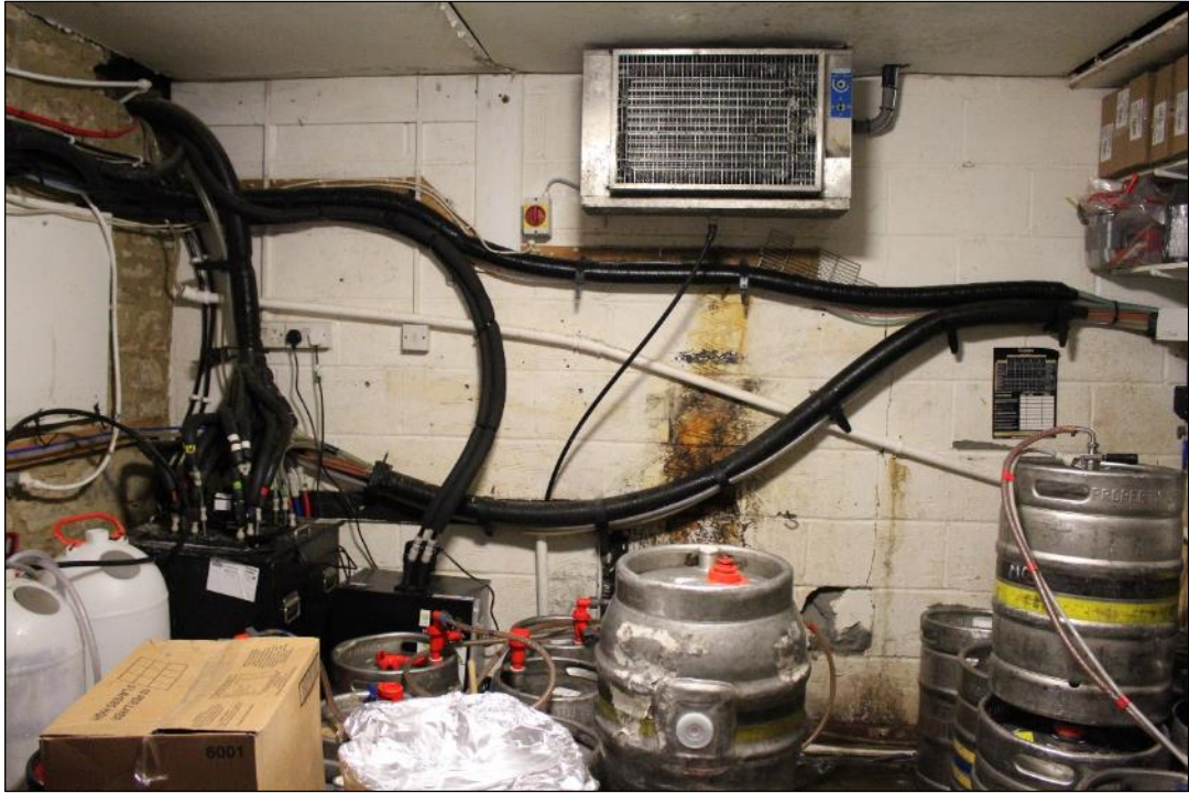
Photo 44: The northern wall of the cellar is of breezeblock construction.
