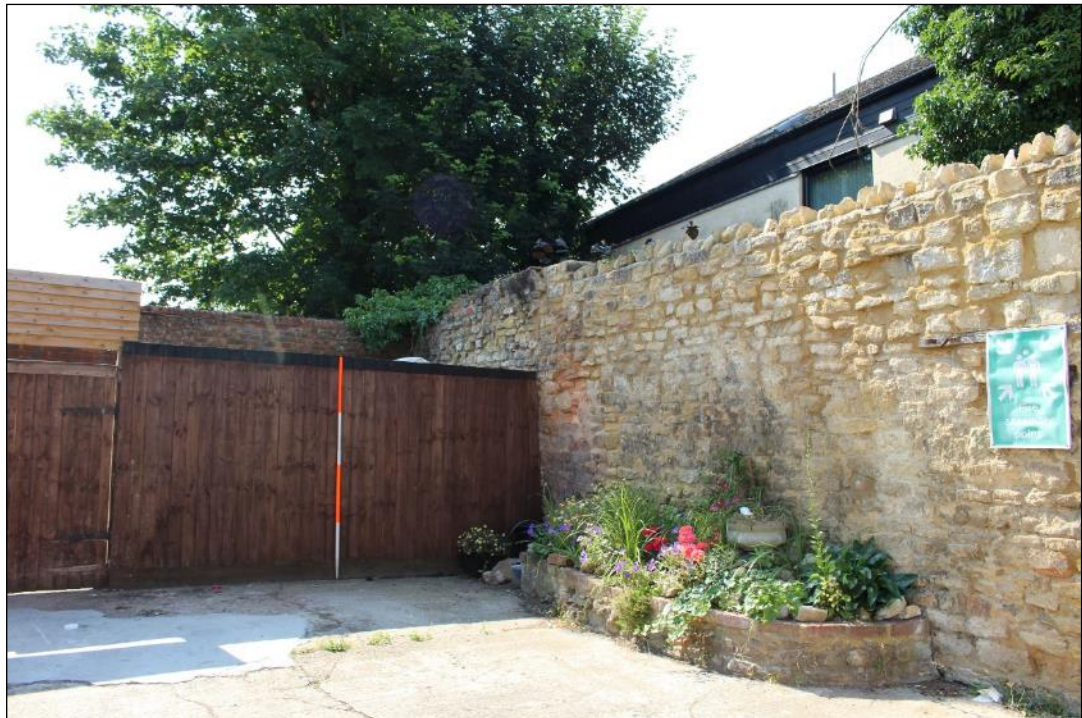
Photo 56: The southern boundary wall form the north-west.
