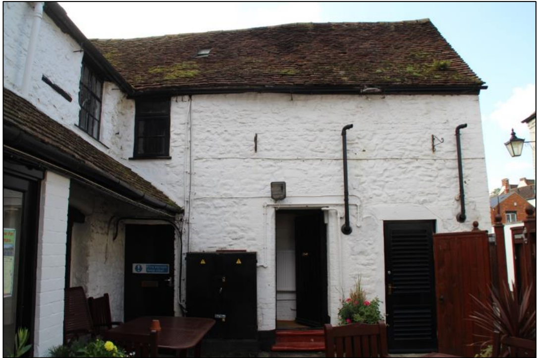
Photo 4: Northern elevation of the late 18th/early 19th-century southern range.
