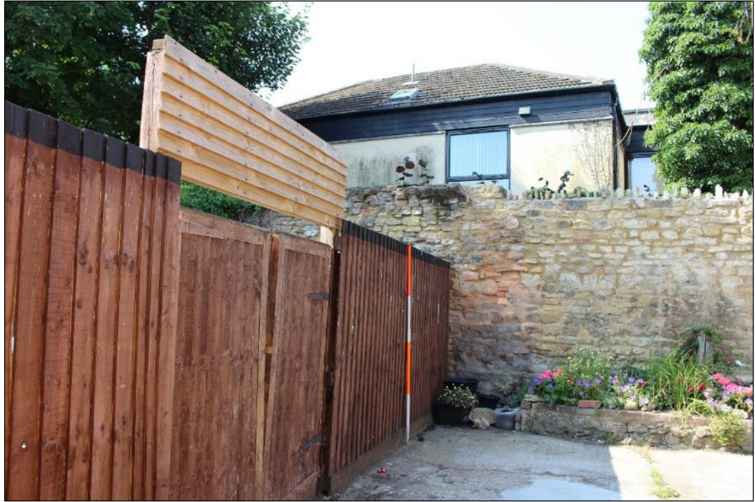
Photo 57: The eastern extent of the boundary wall from the north.
