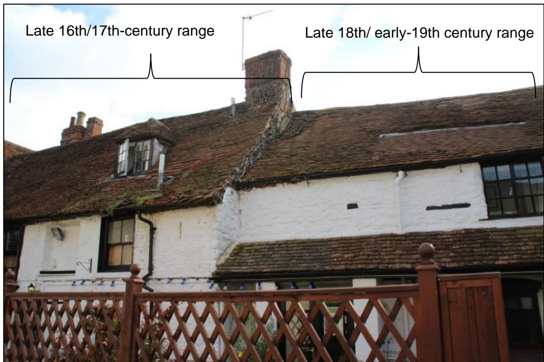
Photo 3: The western elevation of The Old George fronting into George Yard.
