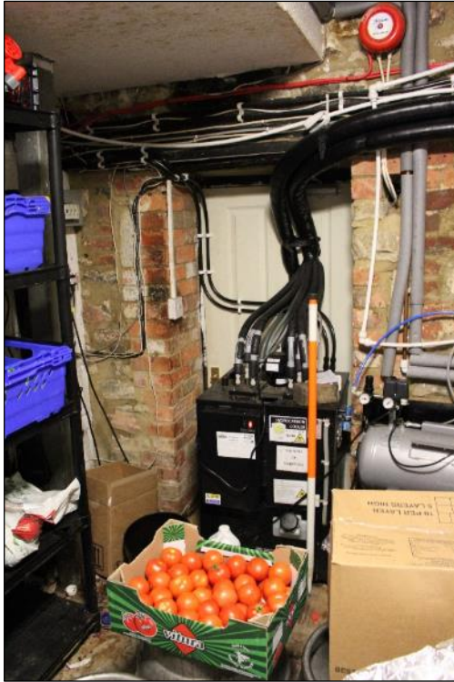
Photo 42: Door opening between the early 20th-century cellar and the northern extent of the dining room.
