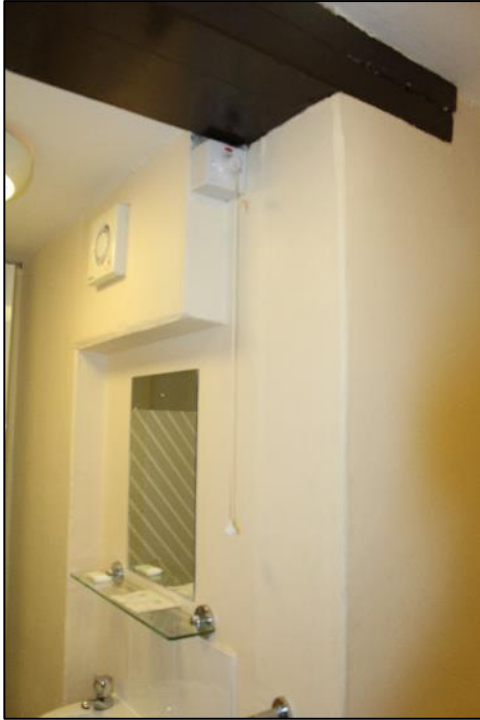
Photo 36: Detail of boxed timber within the en-suite bathroom of Room 7.
