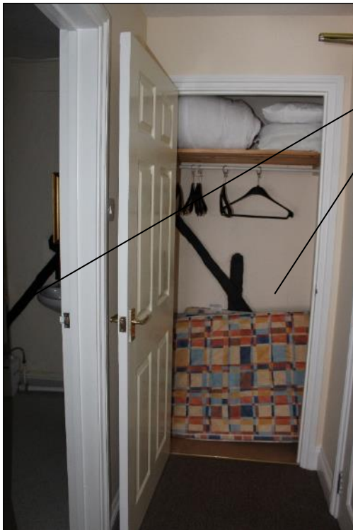
Photo 60: An overview of exposed timber framing within the cupboard of Room 10.
