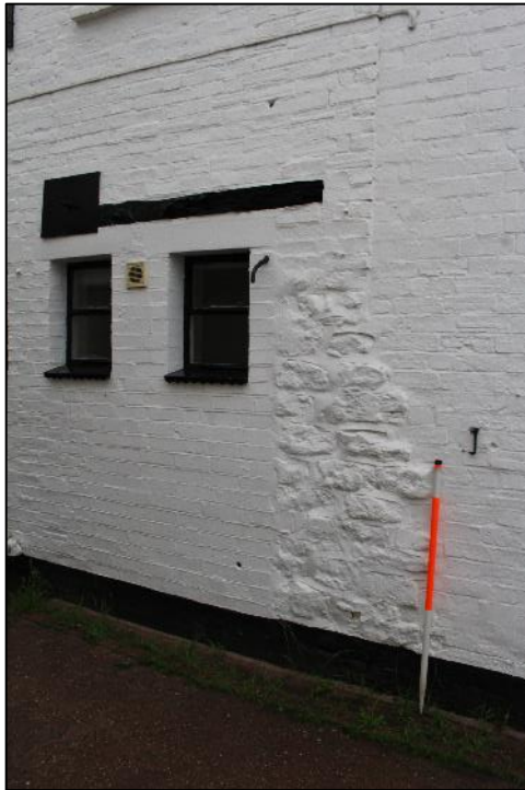
Photo 10: An area of rubblestone within the re-built western gable end.
