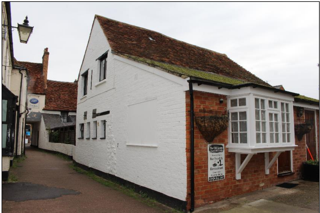
Photo 7: The eastern and southern elevations from the south-west.
