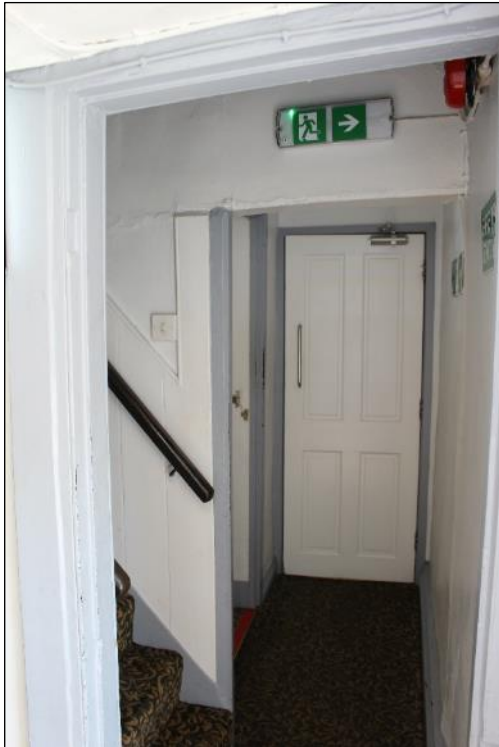
Photo 75: An overview of the southern extent of the eastern corridor.
