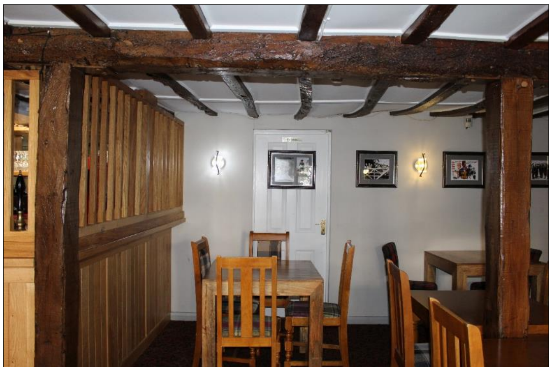
Photo 12: The eastern wall of the northern dining room with access to the cellar.
