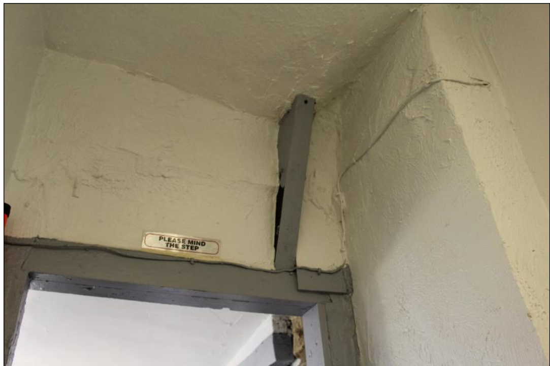
Photo 72: Detail of bracket above door opening within the western corridor.
