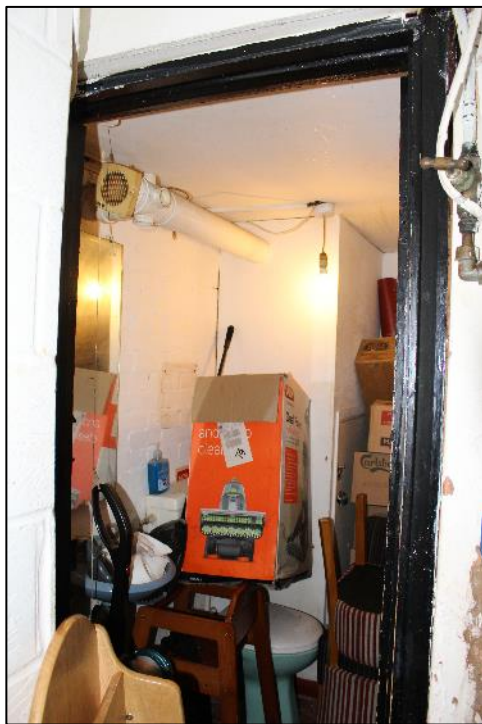
Photo 29: Detail of timber door opening.
