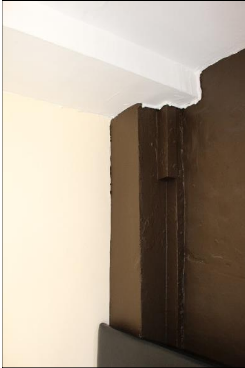
Photo 19: Detail of beam and post within the north-eastern corner of Room 7.
