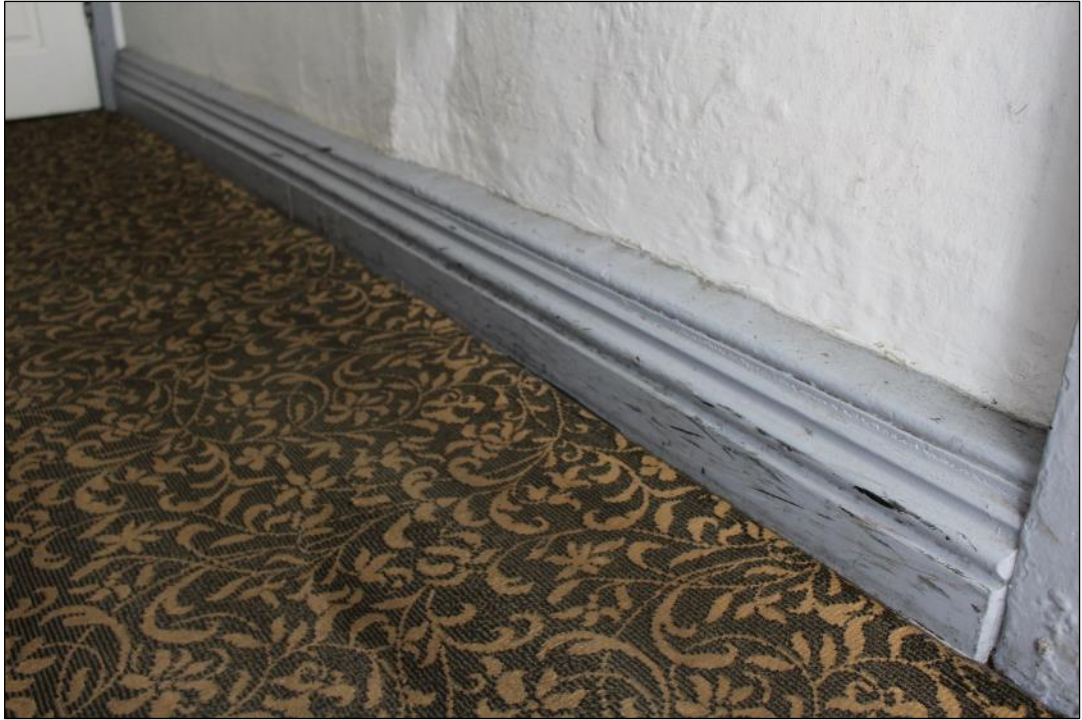
Photo 76: Detail of moulded skirting against the eastern elevation of the eastern corridor.
