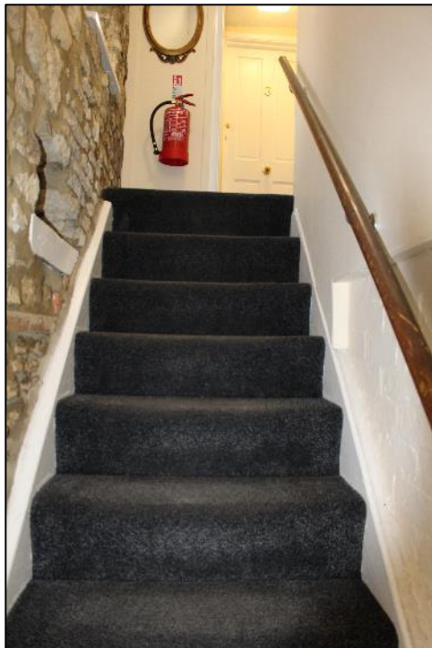
Photo 23: An overview of the stairwell.
