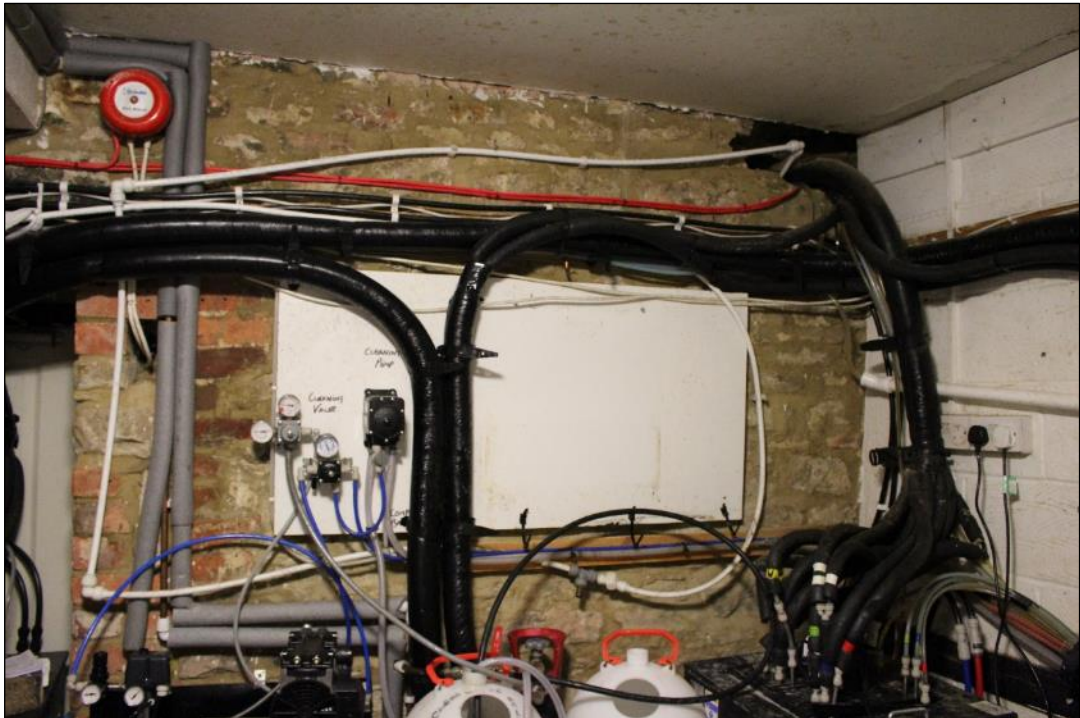
Photo 43: The western wall of the cellar is of rubblestone construction.
