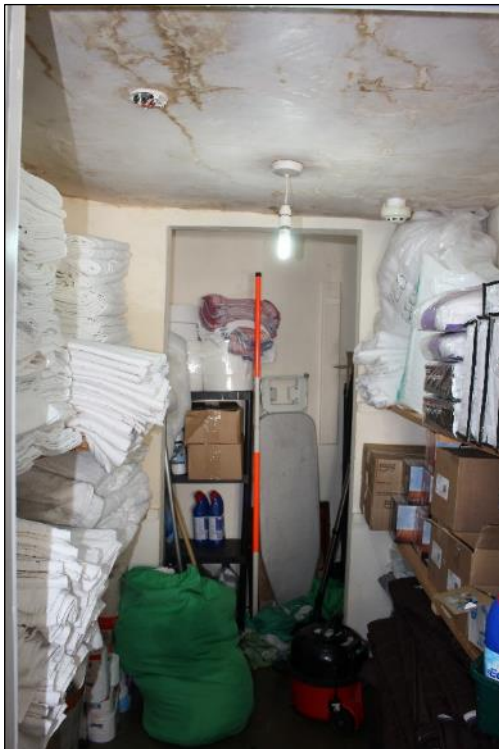
Photo 70: An overview of the Linen Cupboard from the west.
