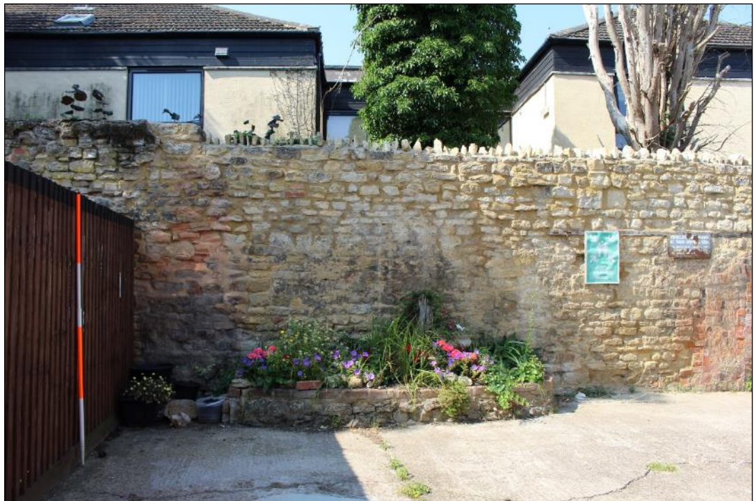
Photo 58: The western extent of the southern boundary wall is finished with upright coping stones.
