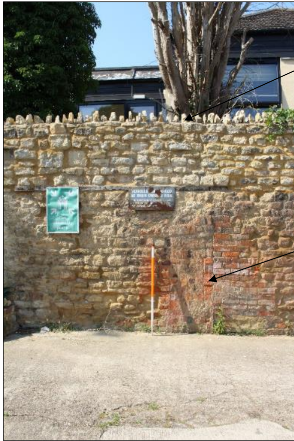
Photo 55: Evidence of a former brick fireplace and flue relating to a now demolished structure visible on the 1st edition Ordnance Survey map.
