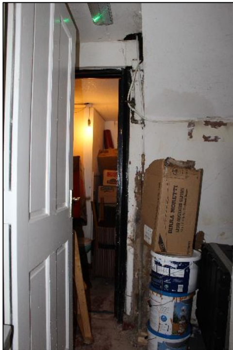
Photo 27: The Staff WC/store from the east.
