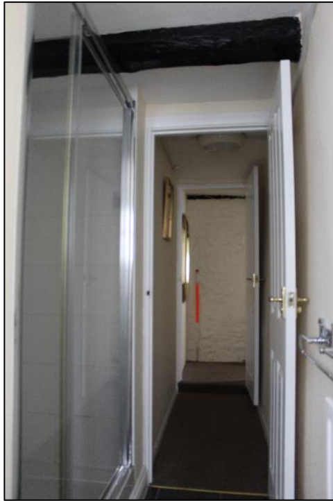
Photo 32: Timber beam within the en-suite bathroom of Room 6.
