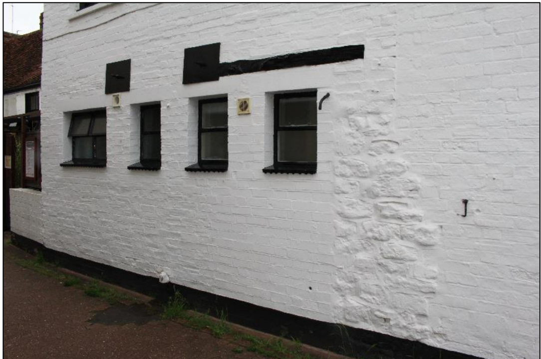
Photo 9: Detail of metal framed window openings within the gable end of the late 18th/early 19th century range.
