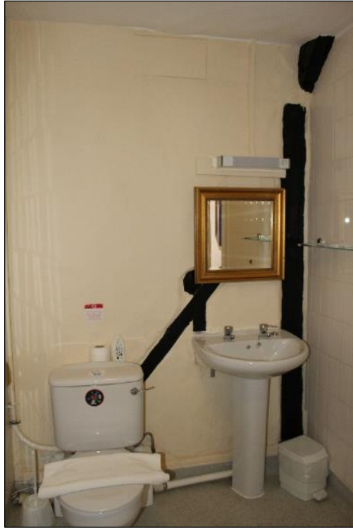
Photo 61: An overview of the timber roof truss set within the southern wall of Room 10.
