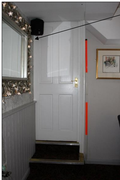
Photo 16: Access between the southern extent of the Dining Room and the staff toilet within the gable end Building.
