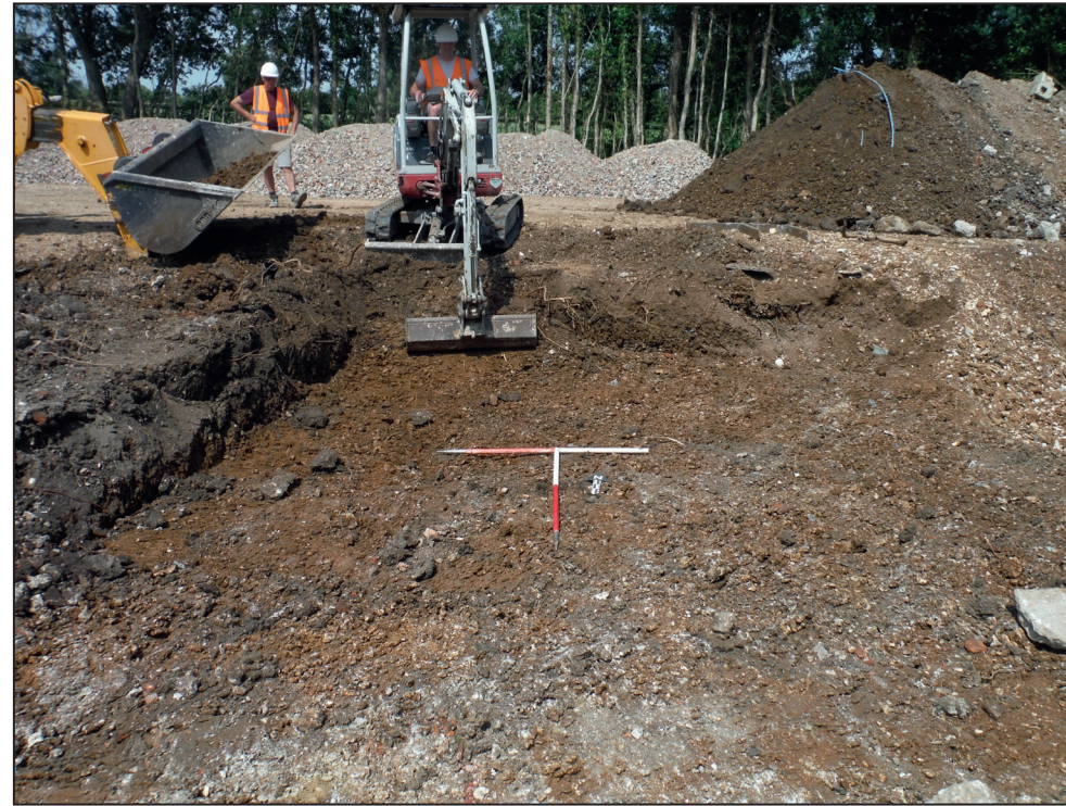
Trench 2, looking south (1m scales)
