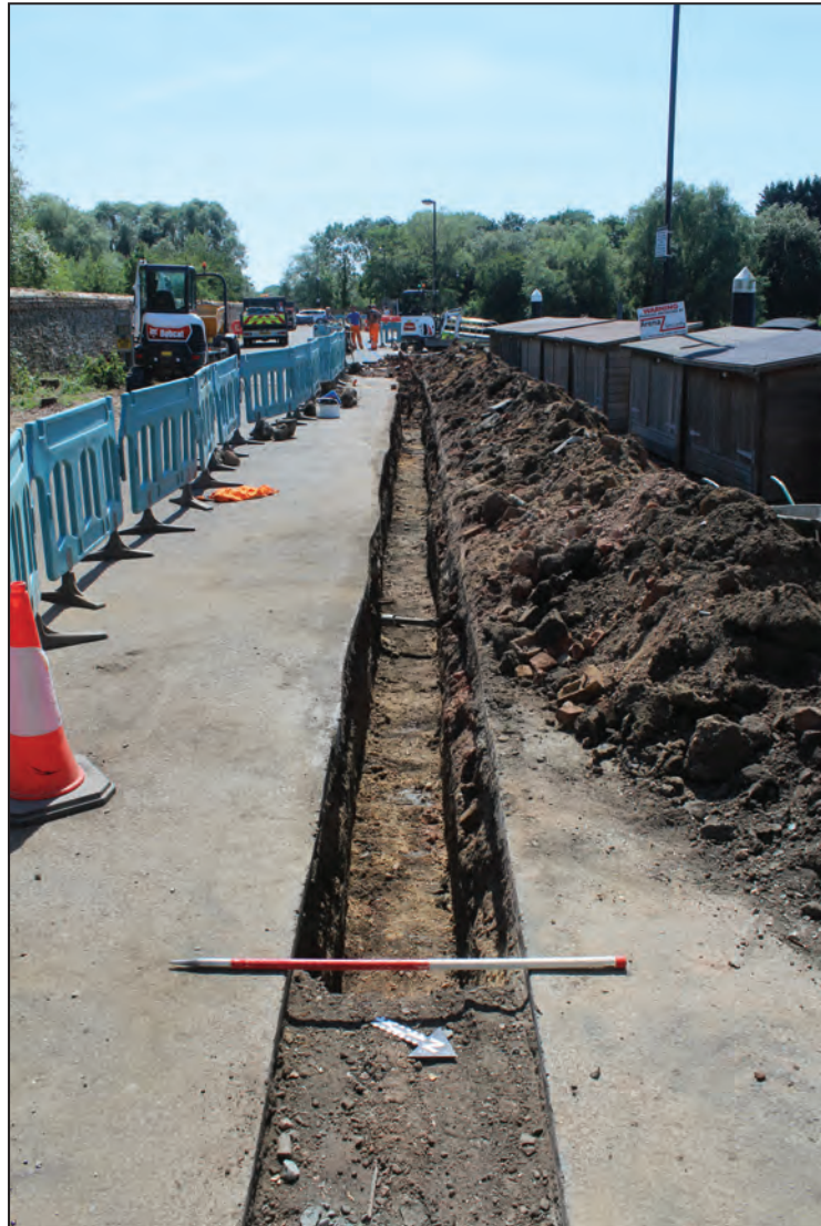
Working shot, looking south-west (1m scale)
