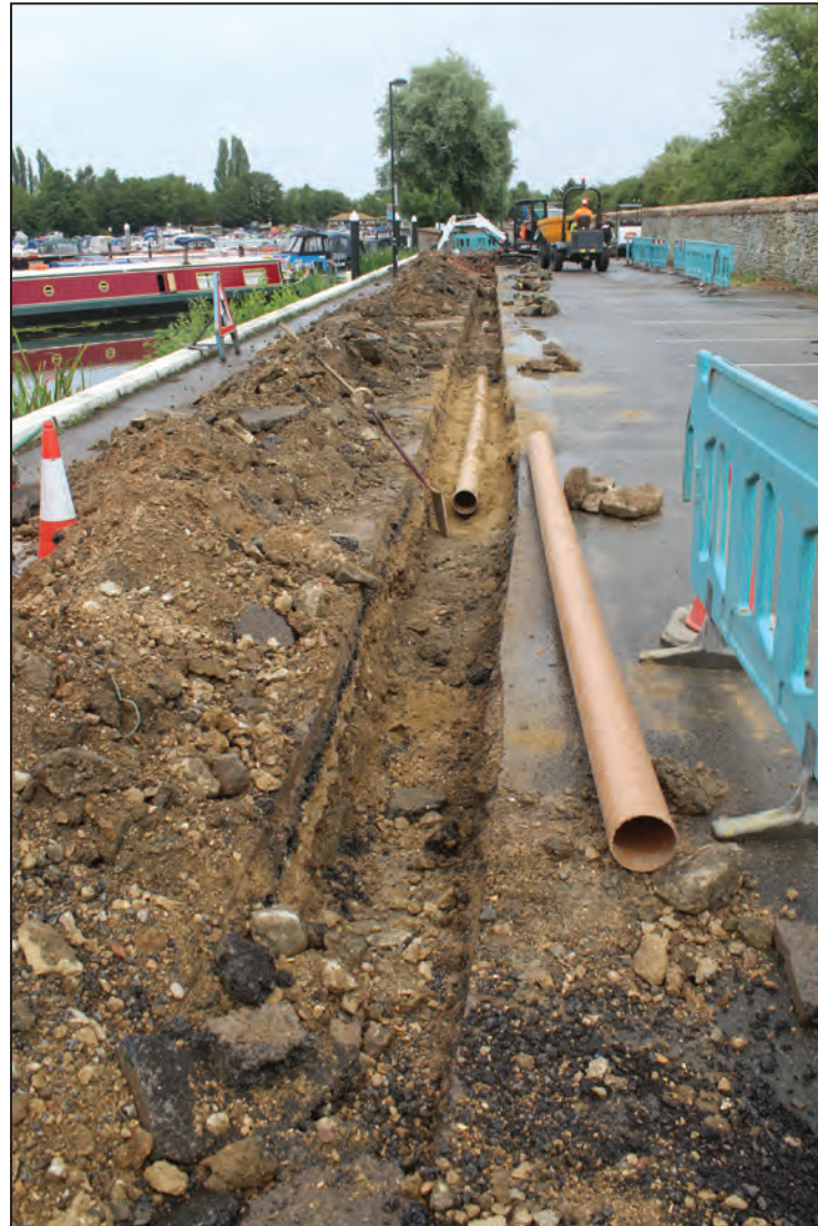
Working shot, looking north-east
