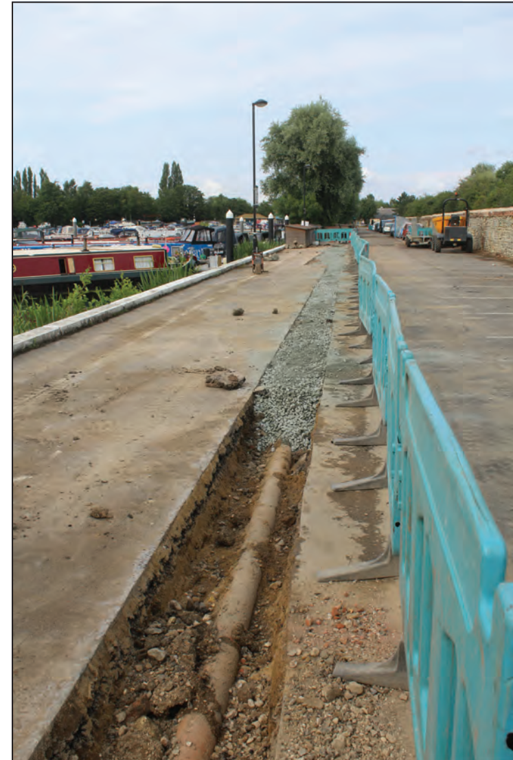
Working shot, looking north-east
