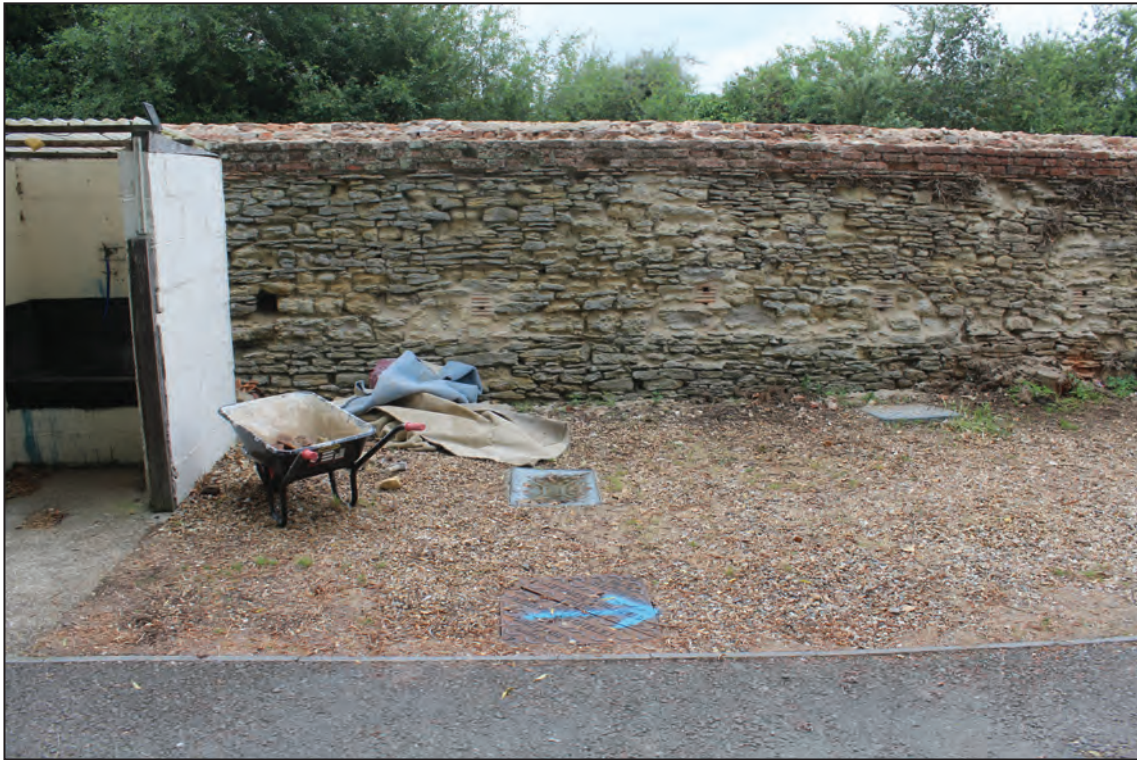
Pre-excitation shot showing boundary wall, looking south-east
