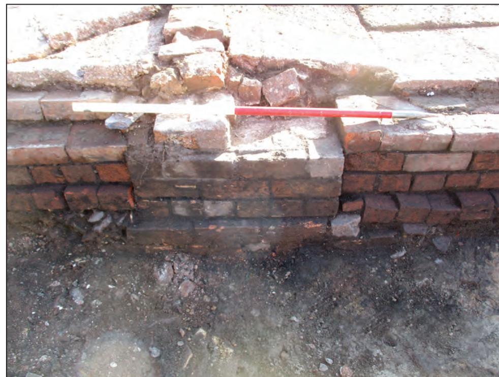
Building B, blocked doorway 1057, looking east (1m scale)
