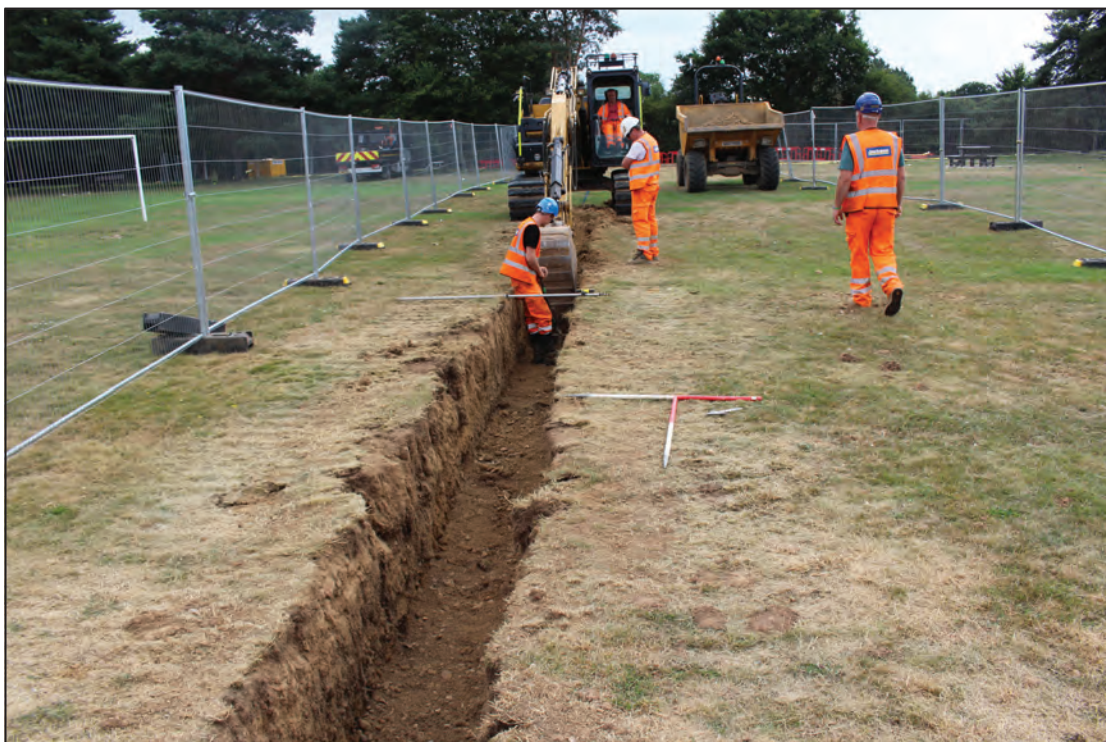
General view of Trench 2.1, looking south-east (1m scales)
