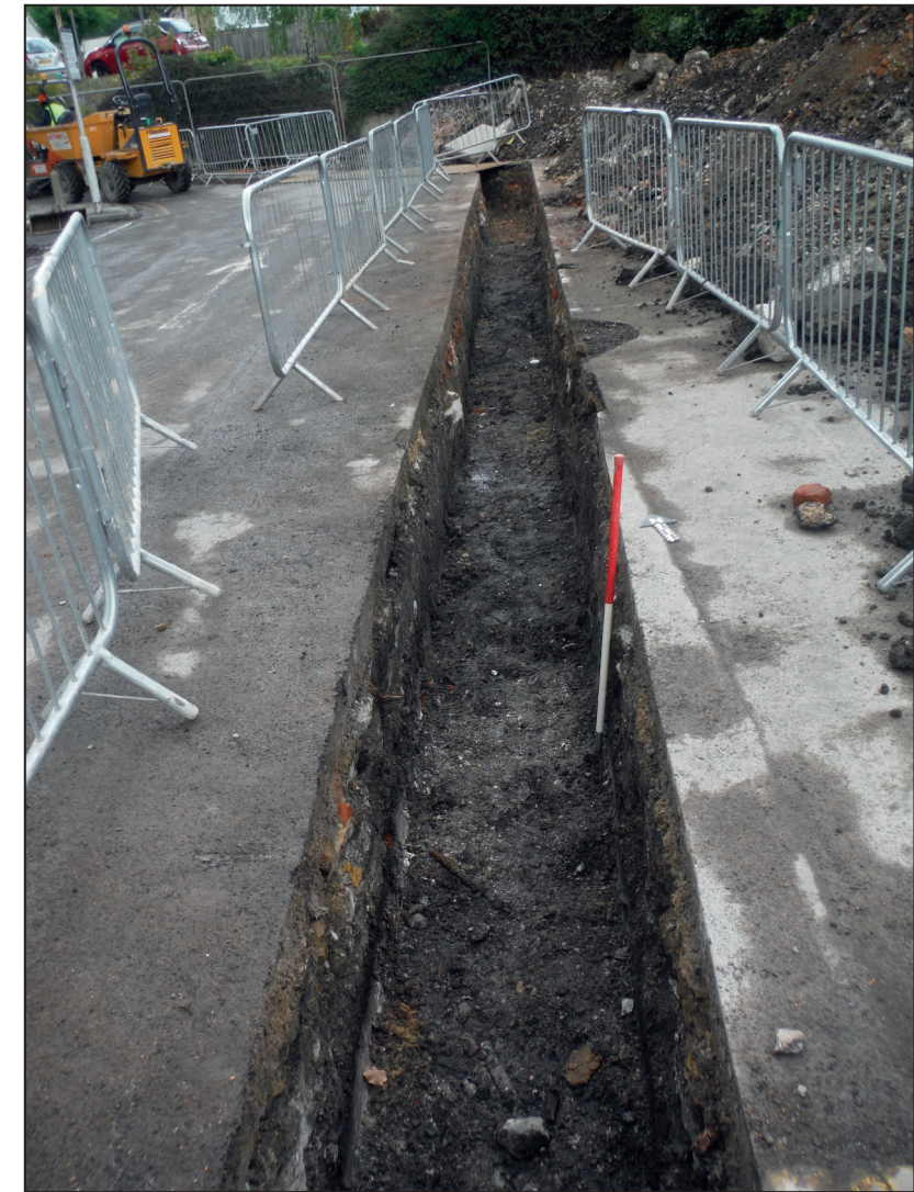
Trench 3, monitored groundworks, looking north (1m scale)
